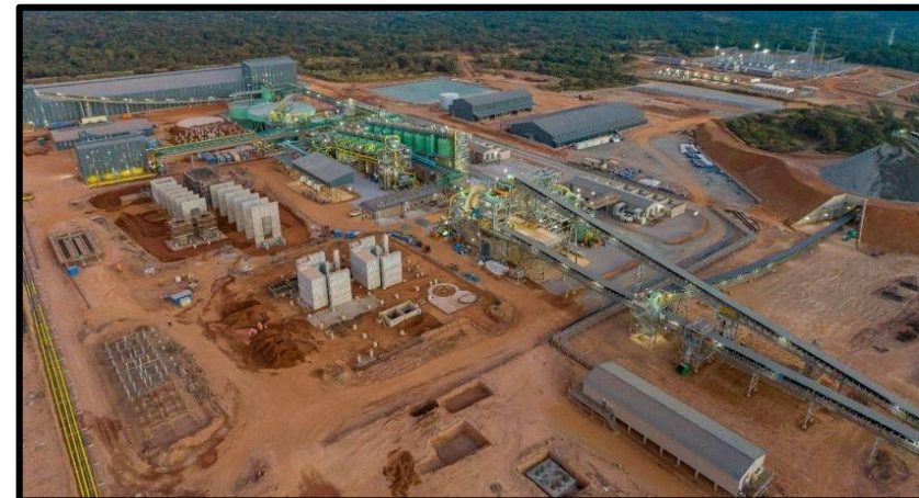
Kamoia-Kakula's Phase 1 concentrator plant, with the foundations for the Phase 2 concentrator on the left.
