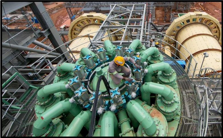
Left: Connecting pneumatic control valves on the primary mill cyclones.
