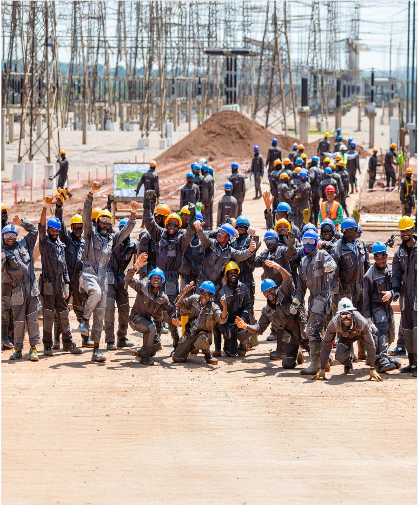
Construction crew assembled at the Kamoa-Kakula Converter Station site.
