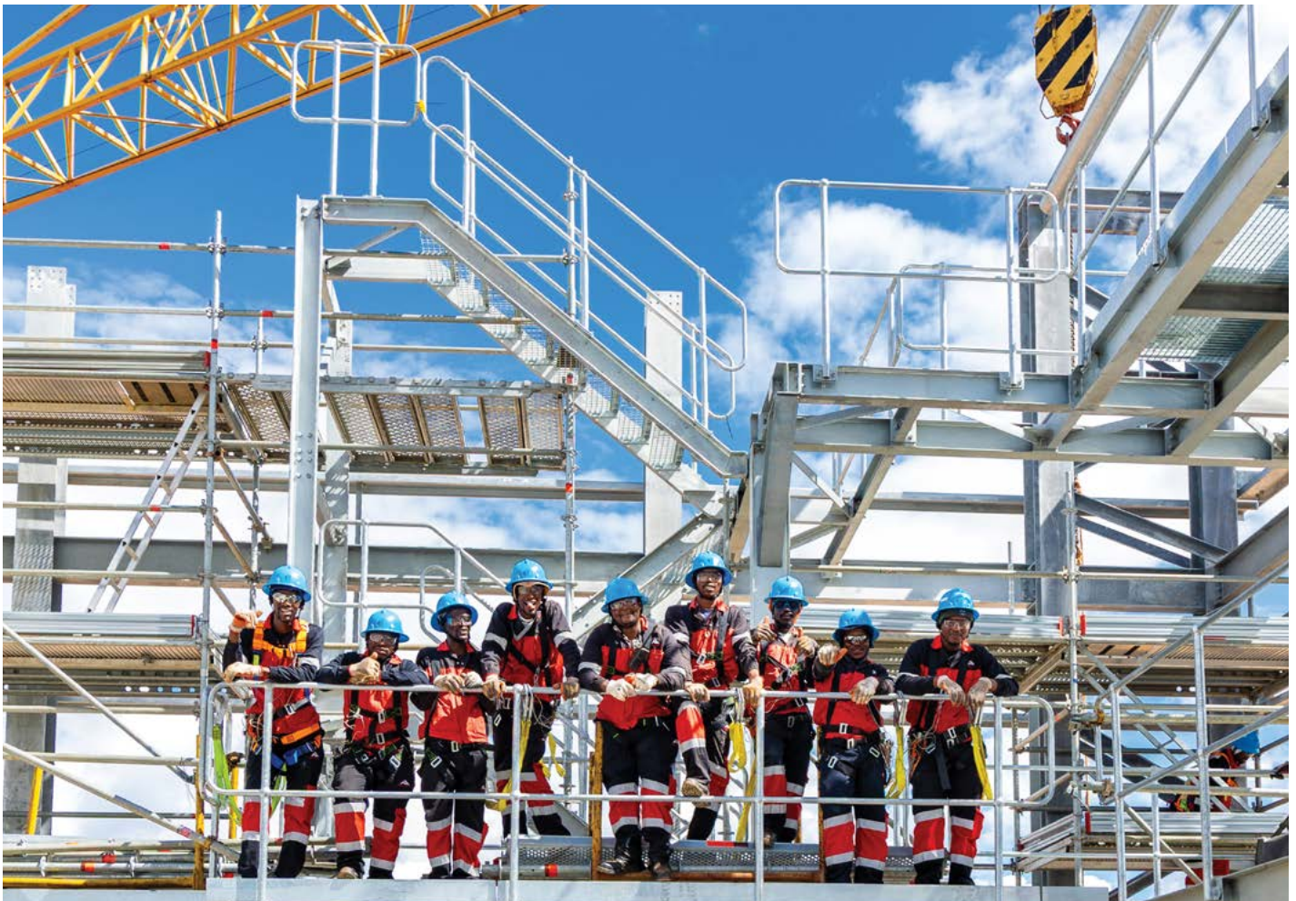
Steel structure workers at the top of Shaft #2 at the Platreef Project.
