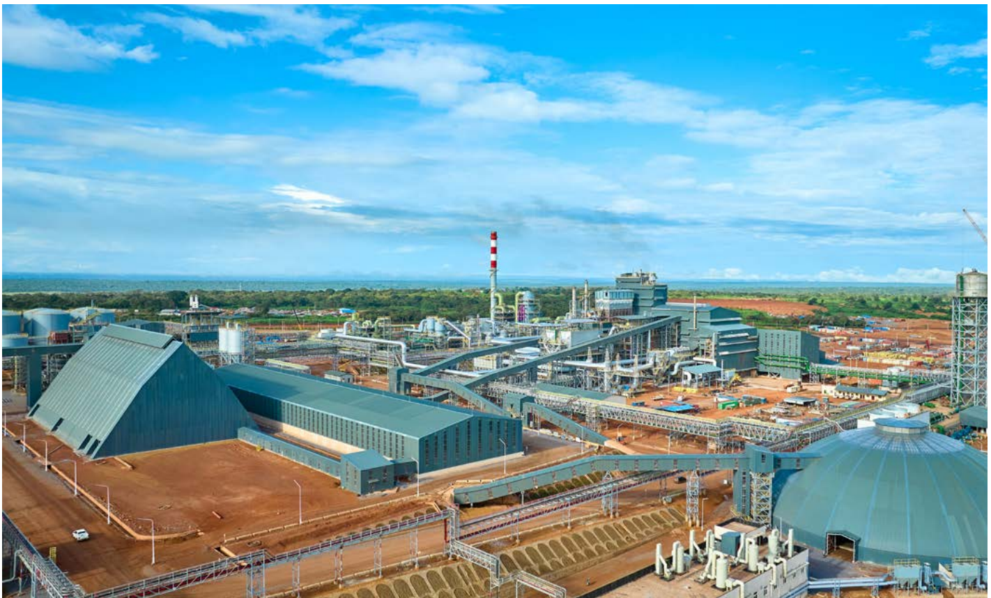
The Kamoā-Kakula smelter complex features the concentrate blending building (right), concentrate storage facility (left), and the smelting building in the background.
