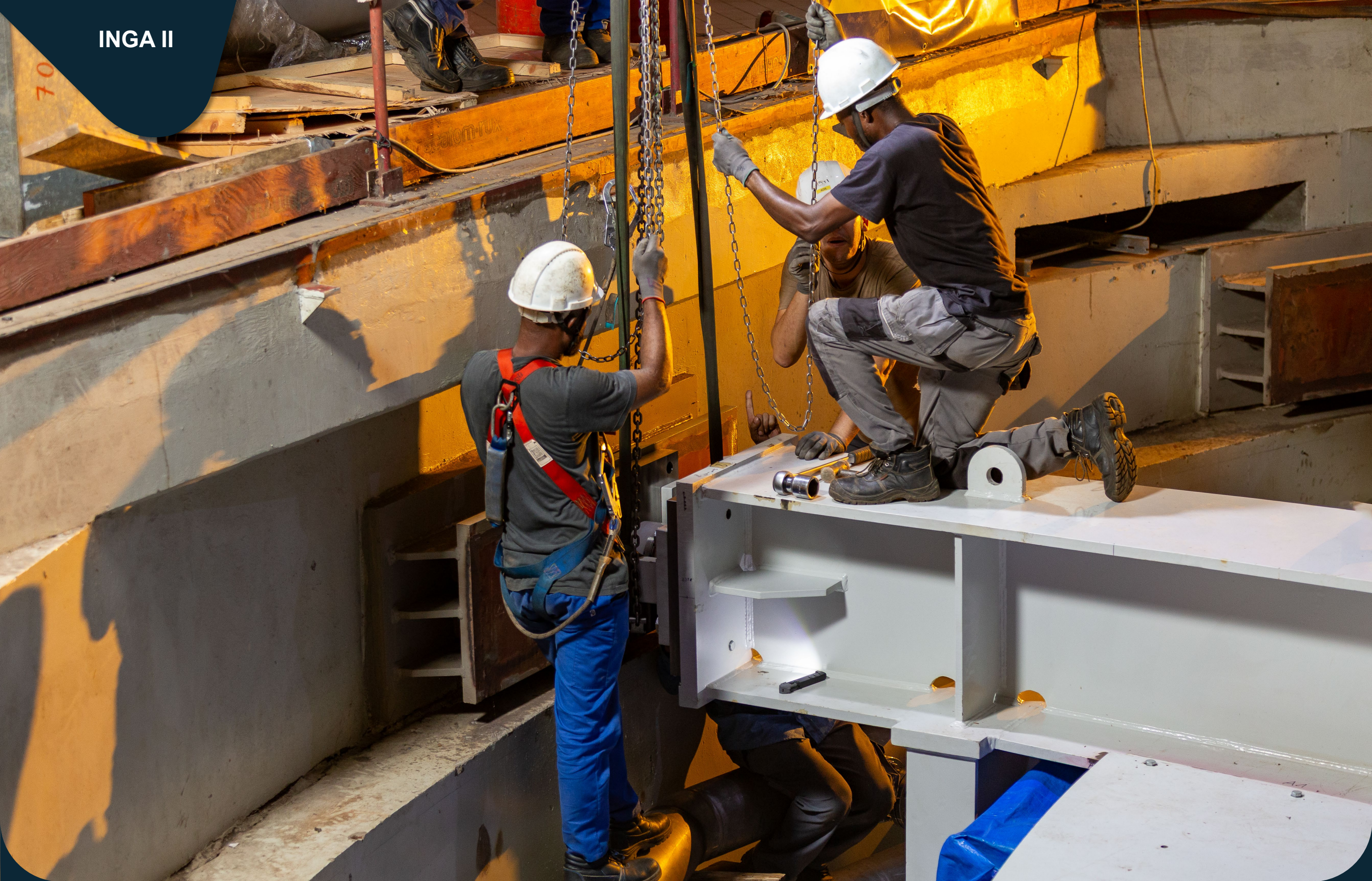
Members of the Inga II project team fitting the thermal expansion dampeners on the turbine upper bracket.
