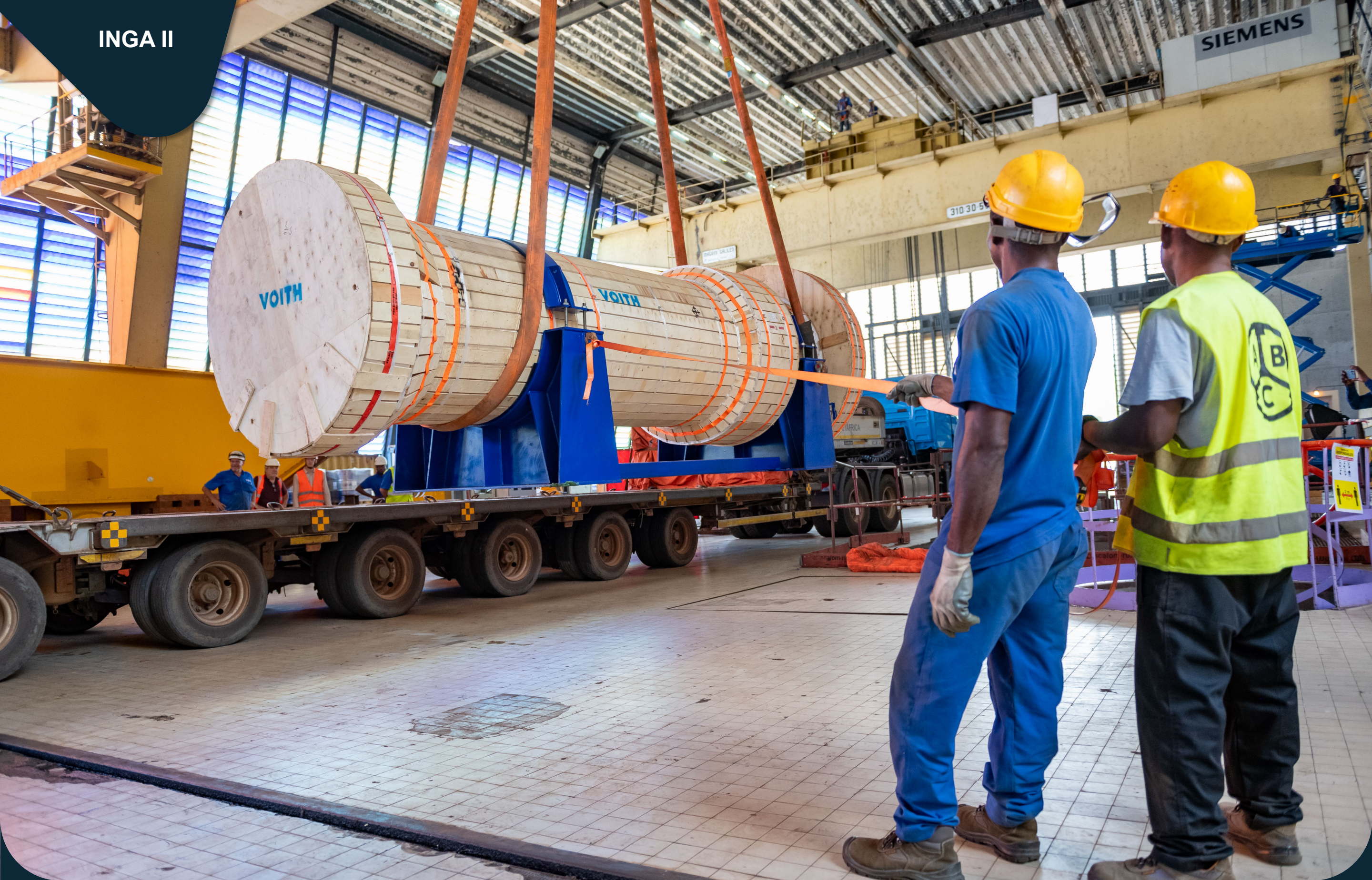
The delivery and unloading of Turbine #5's new turbine shaft inside the turbine hall at Inga II.
