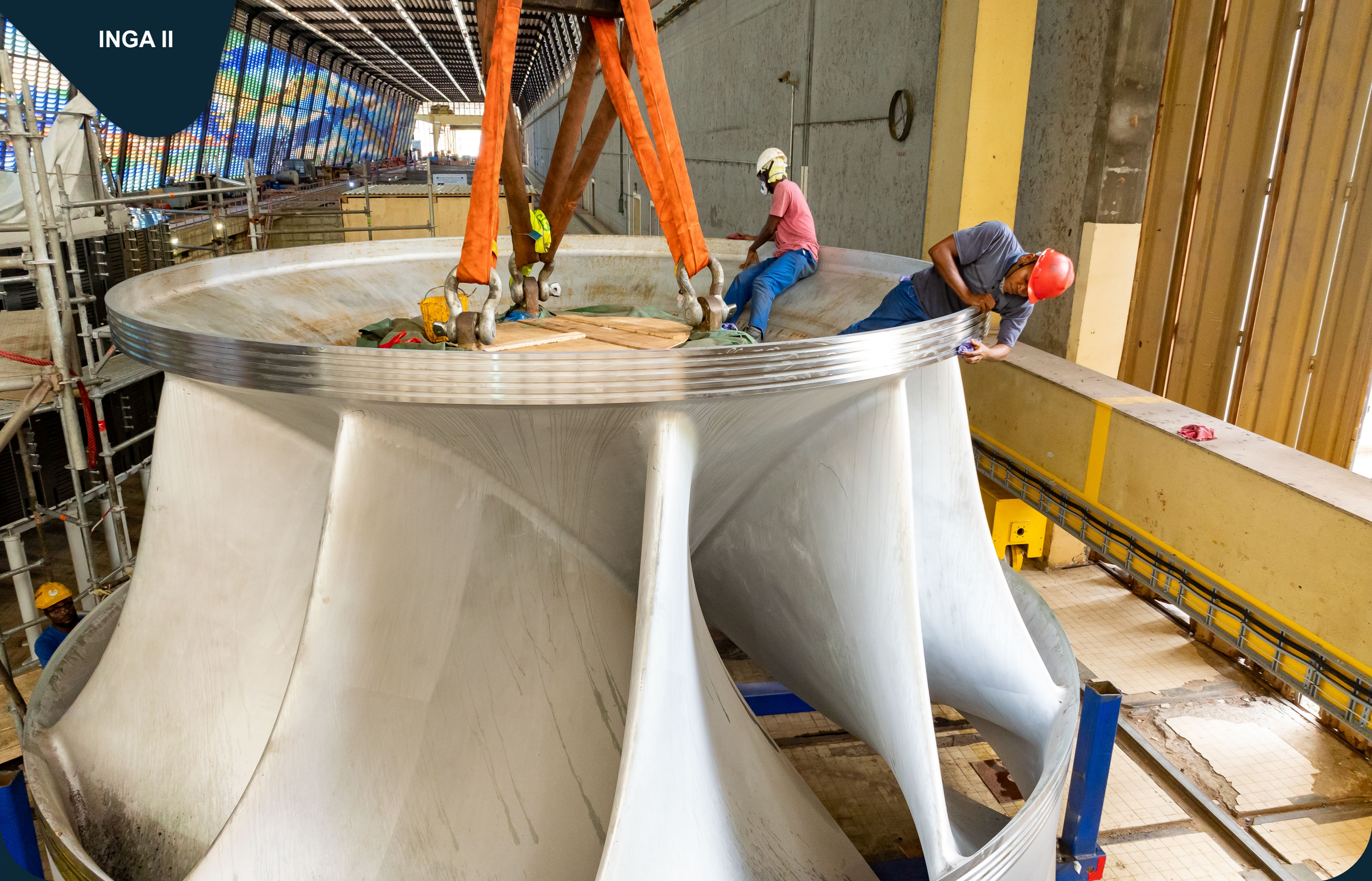
Crew members preparing the newly delivered runner for Turbine #5, before being lowered into the turbine pit and installed.
