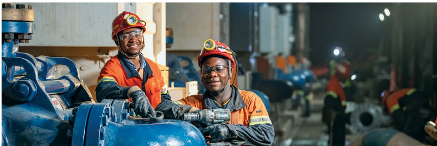
Patrick Motomb Kasamb (L), and Vital Mumbi Nkulu (R), performing maintenance operations at the underground pump station of Kamoa-Kakula.
