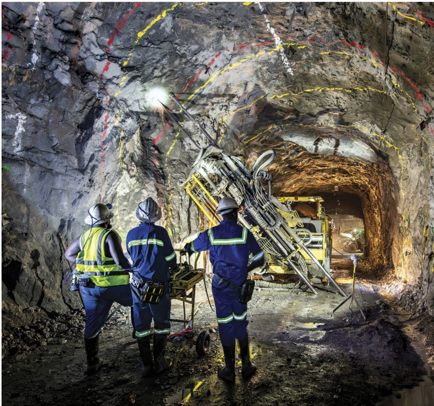
A remotely-operated Simba 1354 longhole drill rig, with its remote operator (center), drilling the stope slot holes on the 1,220-metre level underground at Kipushi.
