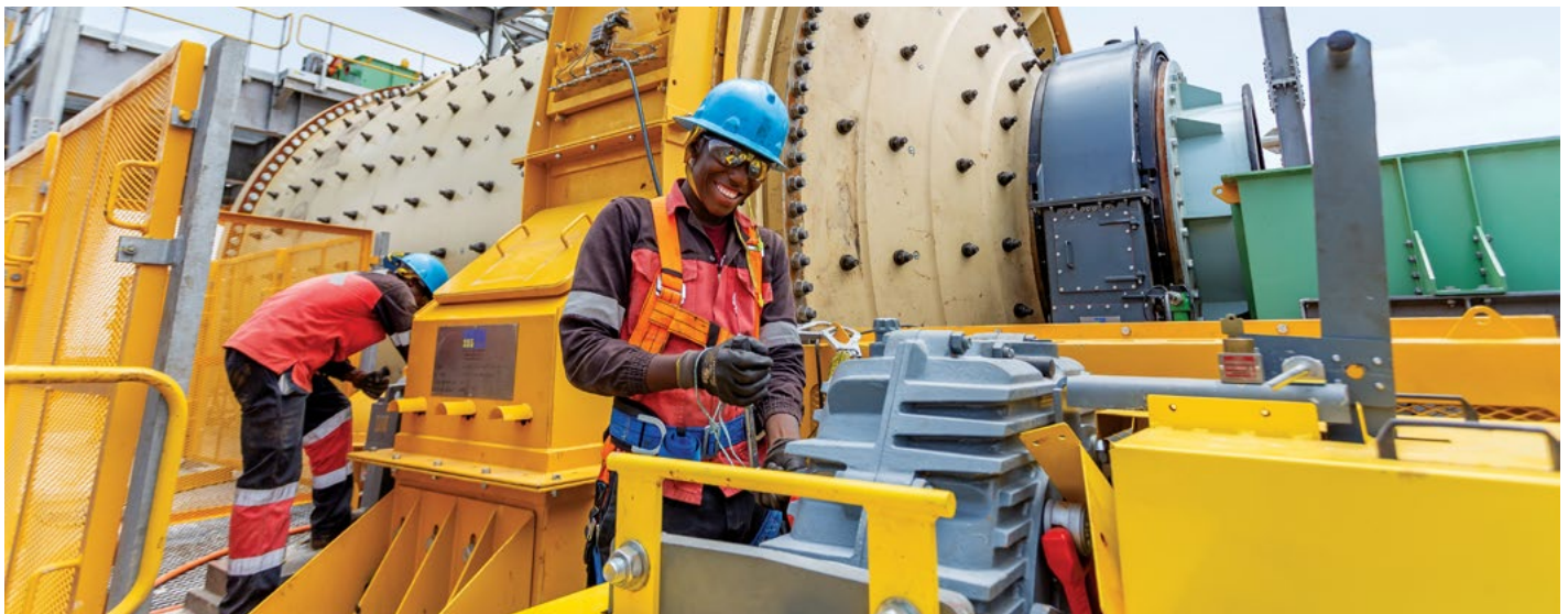
Shshephang Less, assists with the installation process of the ball mills at the Platreef Project's concentrator facility.
