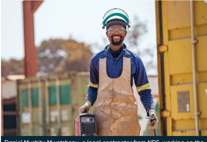
Daniel Mushitu Mwetshenu, a local contractor from NDS, working on the upgraded facility for the expansion of Chatuta Couture, one of Kamo-a-Kakula’s enterprise development initiatives.
