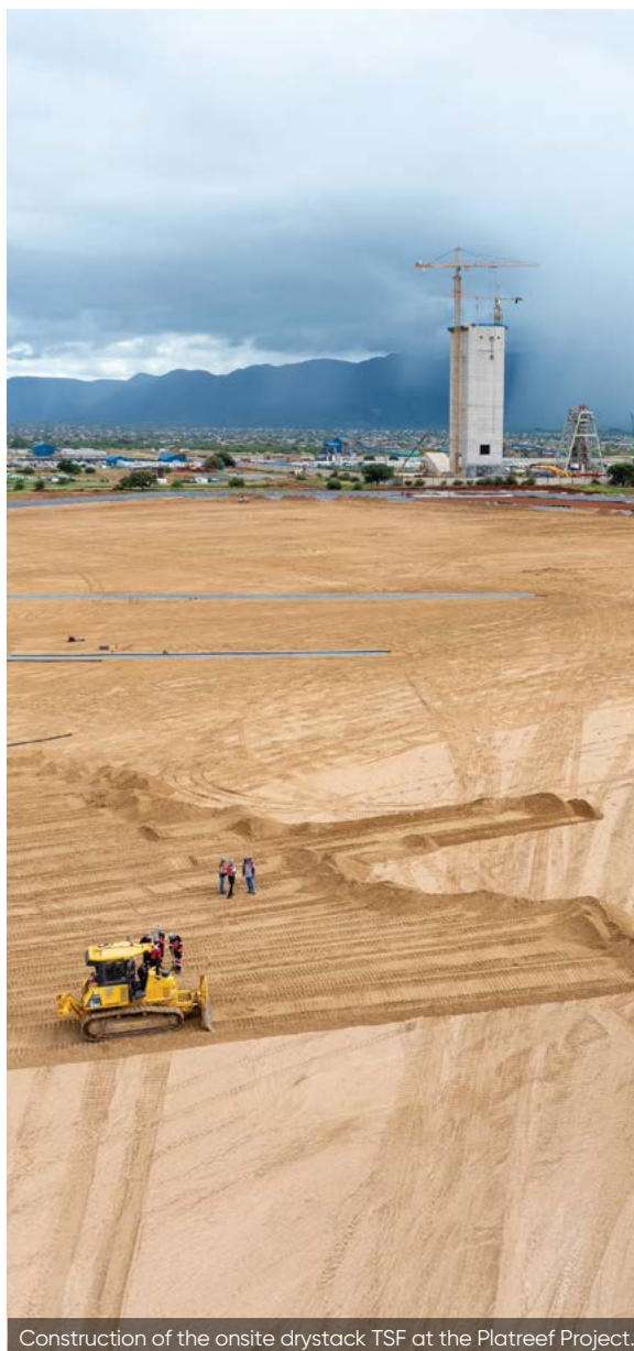
Construction of the onsite drystack TSF at the Platreef Project.
