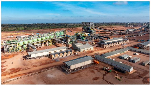
The Phase 3 concentrator is 30% larger in capacity compared with the Phase 1 and 2 concentrators. The process design is very similar, therefore the bulk of the equipment is the same or similar to that installed in the Phase 1 and 2 concentrators, resulting in a commonality of spare parts, while also leveraging prior operational and maintenance experience.
