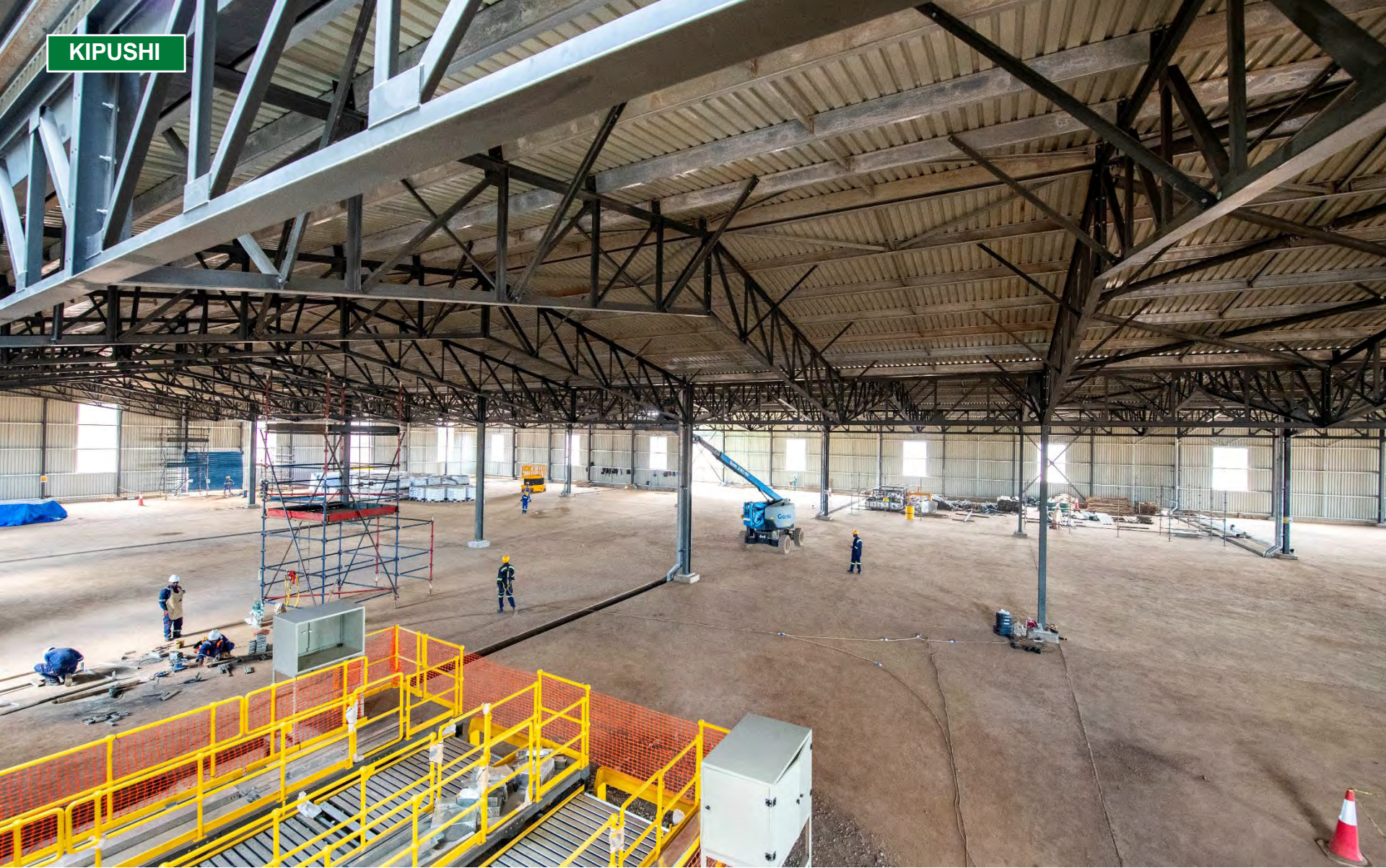
Electrical installation progresses well at Kipushi's concentrate storage shed.
