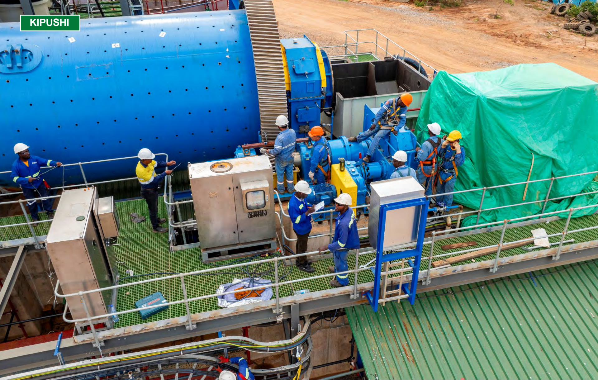
Crew members align the girth gear at the Kipushi ball mill.
