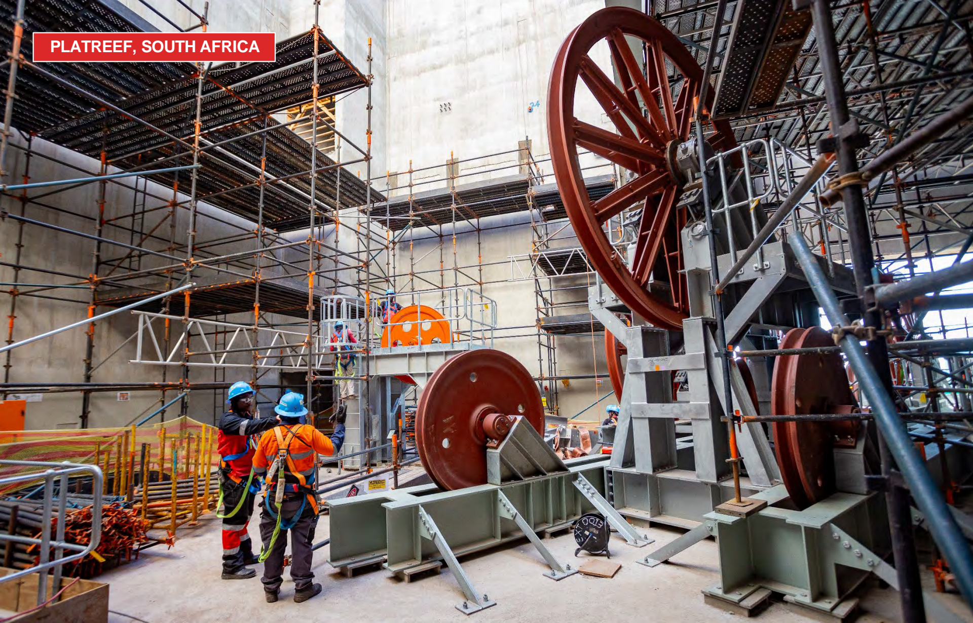
Construction crew on the main sheave deck inside Platreef's Shaft 2 headgear.
