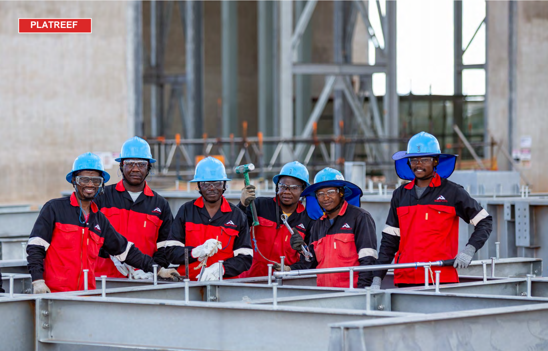
Platreef's construction team lay down steel inside the Shaft #2.
