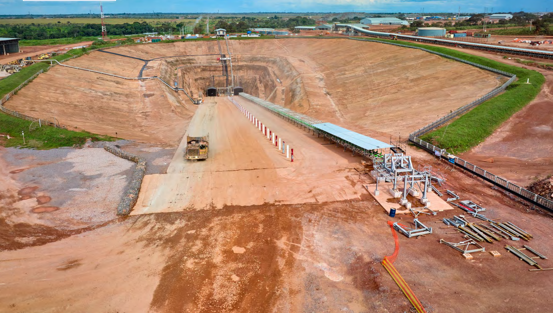
Assembly of the decline conveyor belt at the Kamoia 1 mine.
