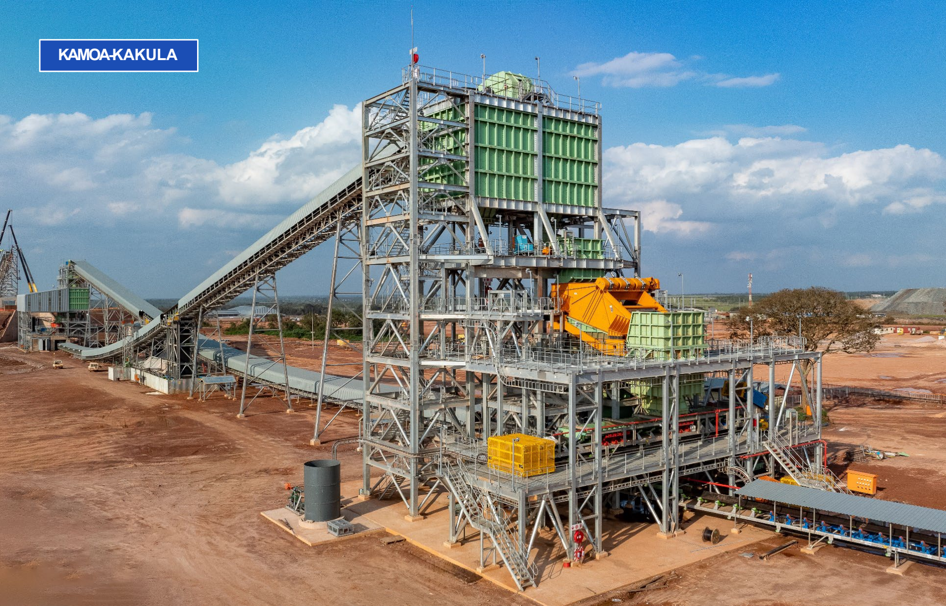
Construction of Kamoa-Kakula's Phase 3 screening building (foreground) and the crushing building in the background.
