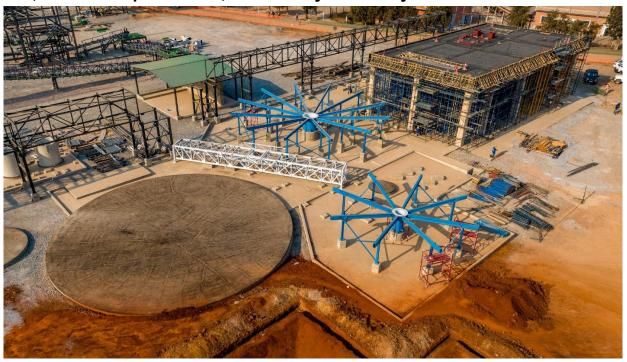
Kipushi steel erection commenced in April 2023 with 1,852 tonnes of a total of 2,214 tonnes dispatched to site.
