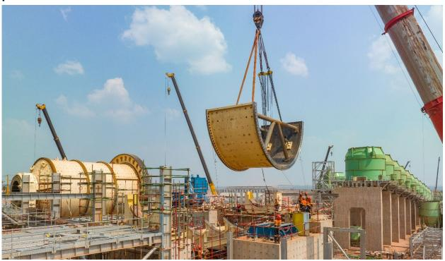
Construction of the concentrate thickener is progressing well at Kamoa-Kakula's Phase 3 concentrator site. The process design of the Phase 3 concentrator is very similar to that of the Phase 1 and 2 concentrators, but 30% larger.
