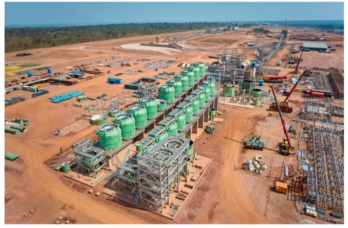
Installation of the first of the two ball mills has commenced at the Phase 3 concentrator site, with flotation cell installation also underway. The first lots of cone crushers, flotation cells, vibrating screens, concentrate filters, cyclone cluster, compressor and pump mechanical equipment packages are now on site or expected to be delivered to site imminently.
