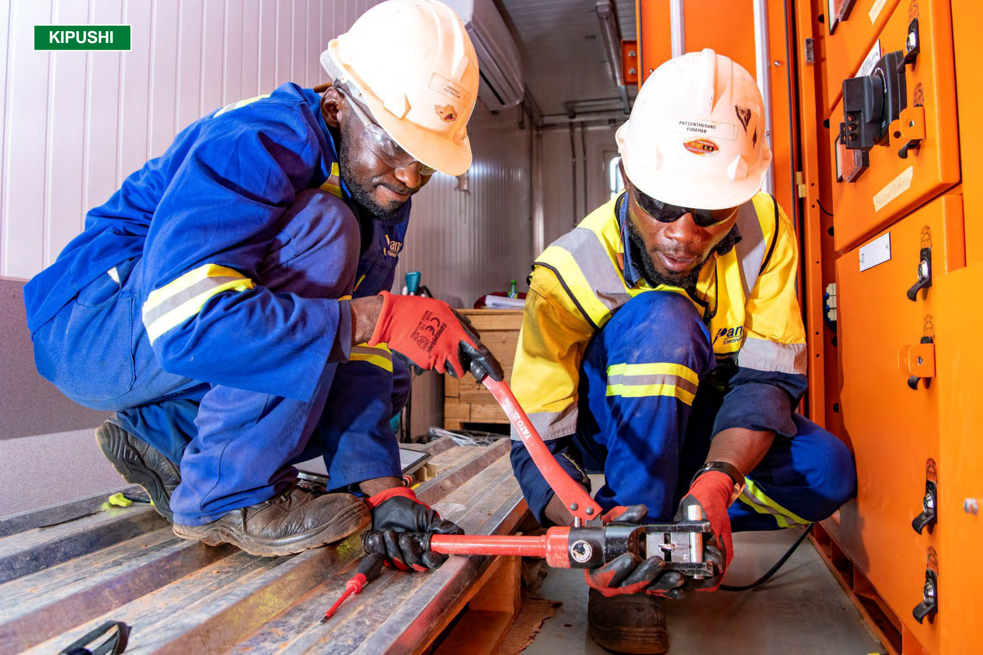
Cable installation in progress at Kipushi's remote substation.
