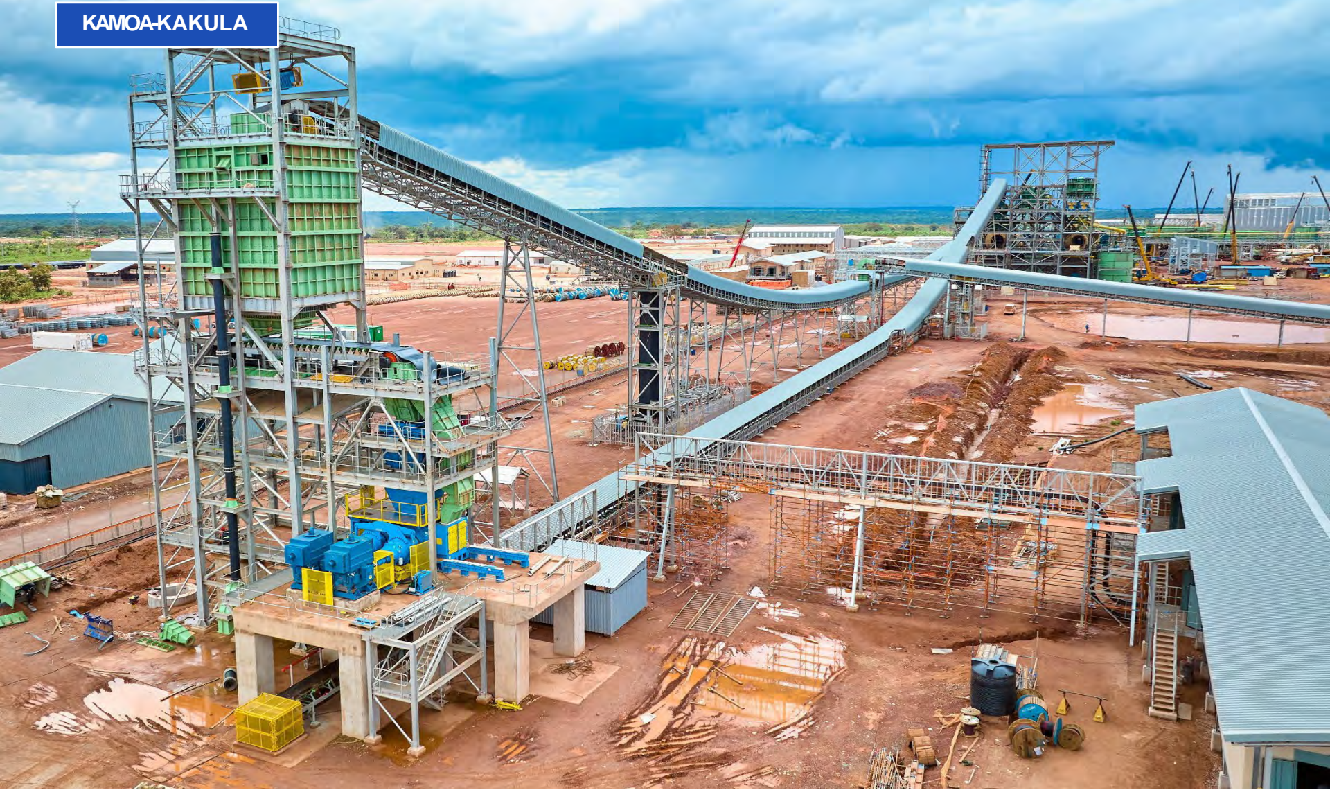
Construction of Kamoa-Kakula's Phase 3 high-pressure-grinding-rolls (HPGR) building.
