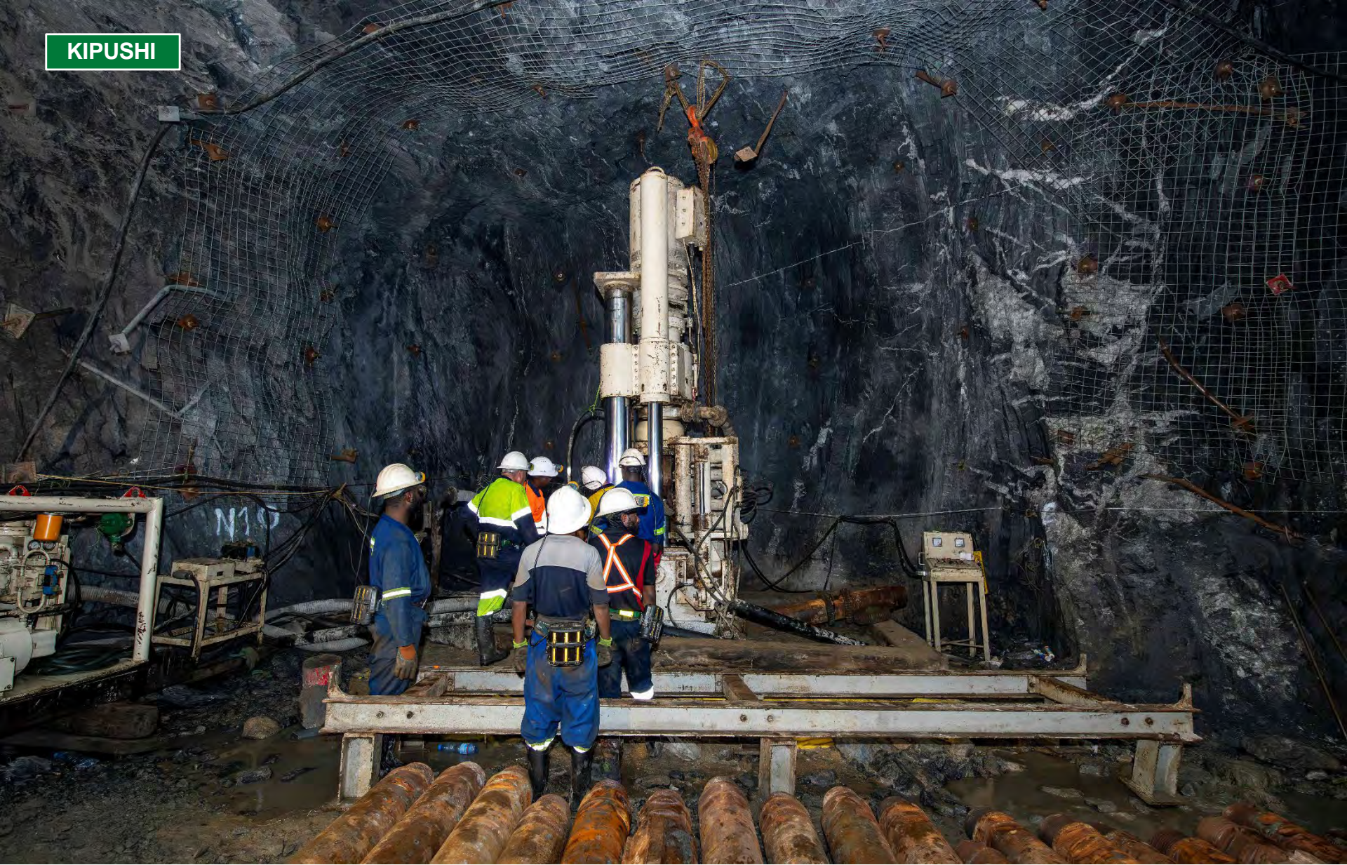
Underground crew members operating a raise-bore machine at Kipushi's 1,245-metre level.
