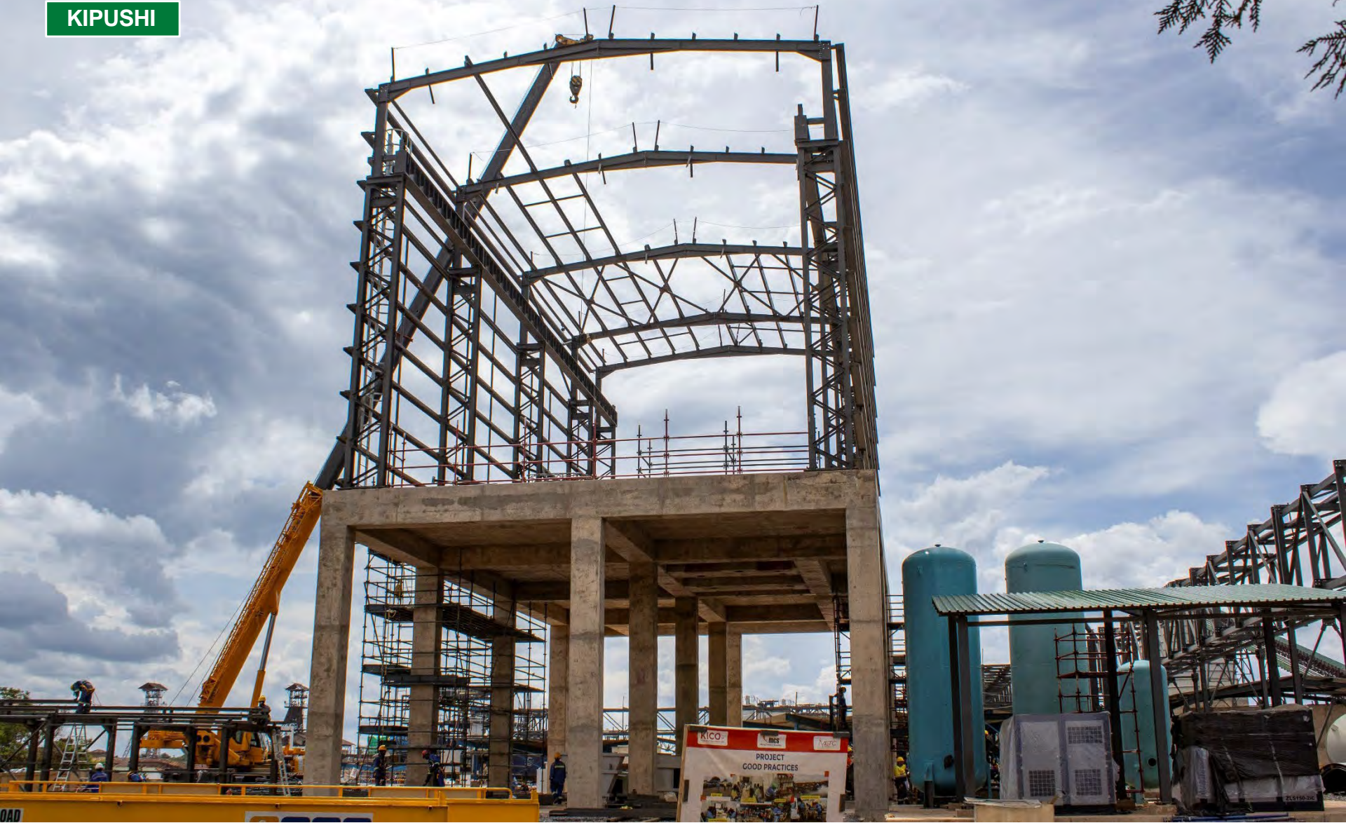
Roof installation at Kipushi's zinc filtration building.
