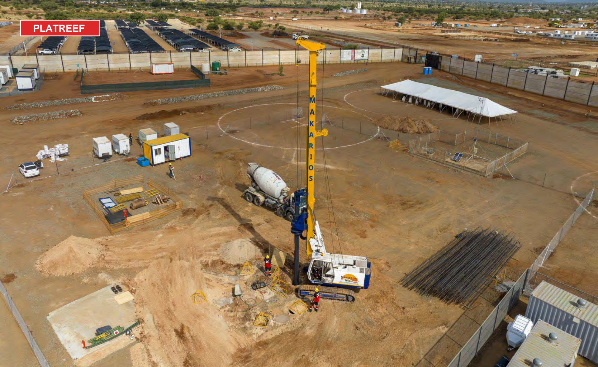
Pilot-hole drilling underway for Platreef's ventilation Shaft 4.
