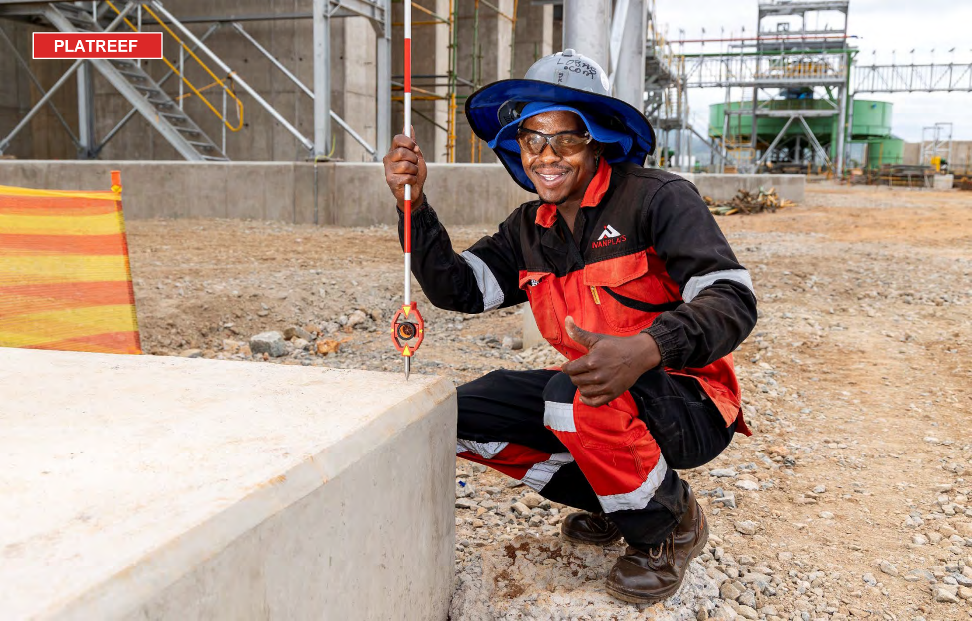
Collen Maloba (Surveyor Assistant) working at Platreef's concentrator site.
