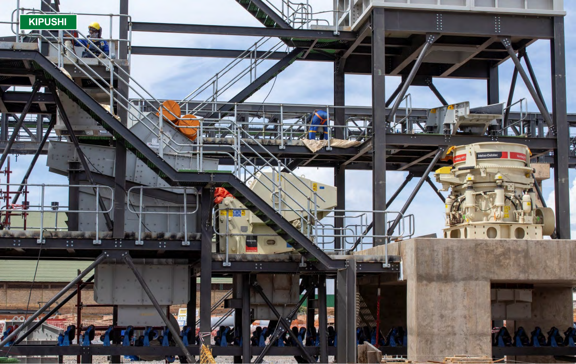
Kipushi's crusher building under construction.
