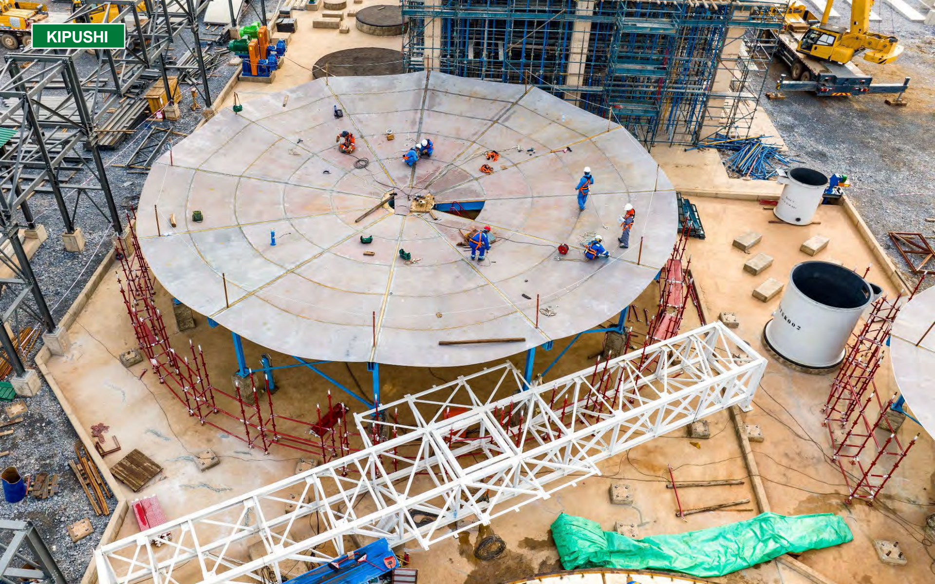
Kipushi's concentrate thickener base plate welding is nearing completion.
