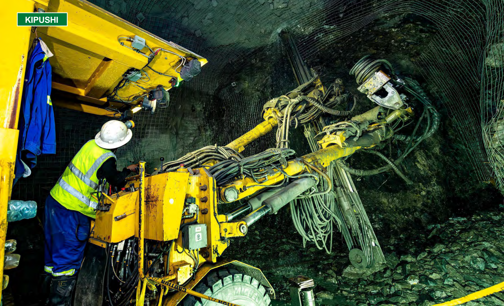
A development drill rig installing wire mesh support underground at Kipushi.
