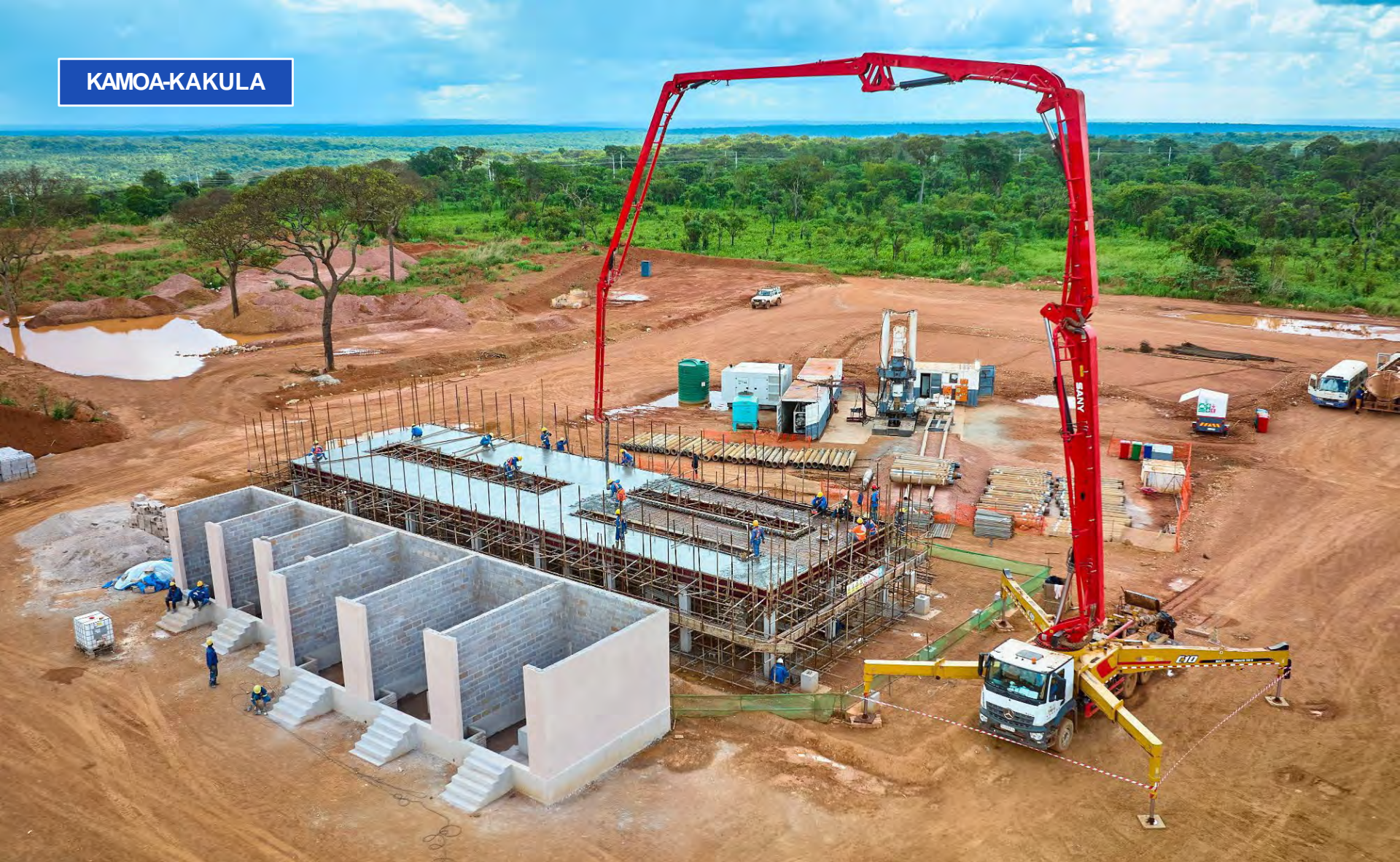
Crews constructing the Phase 3 southwest ventilation shaft substation.
