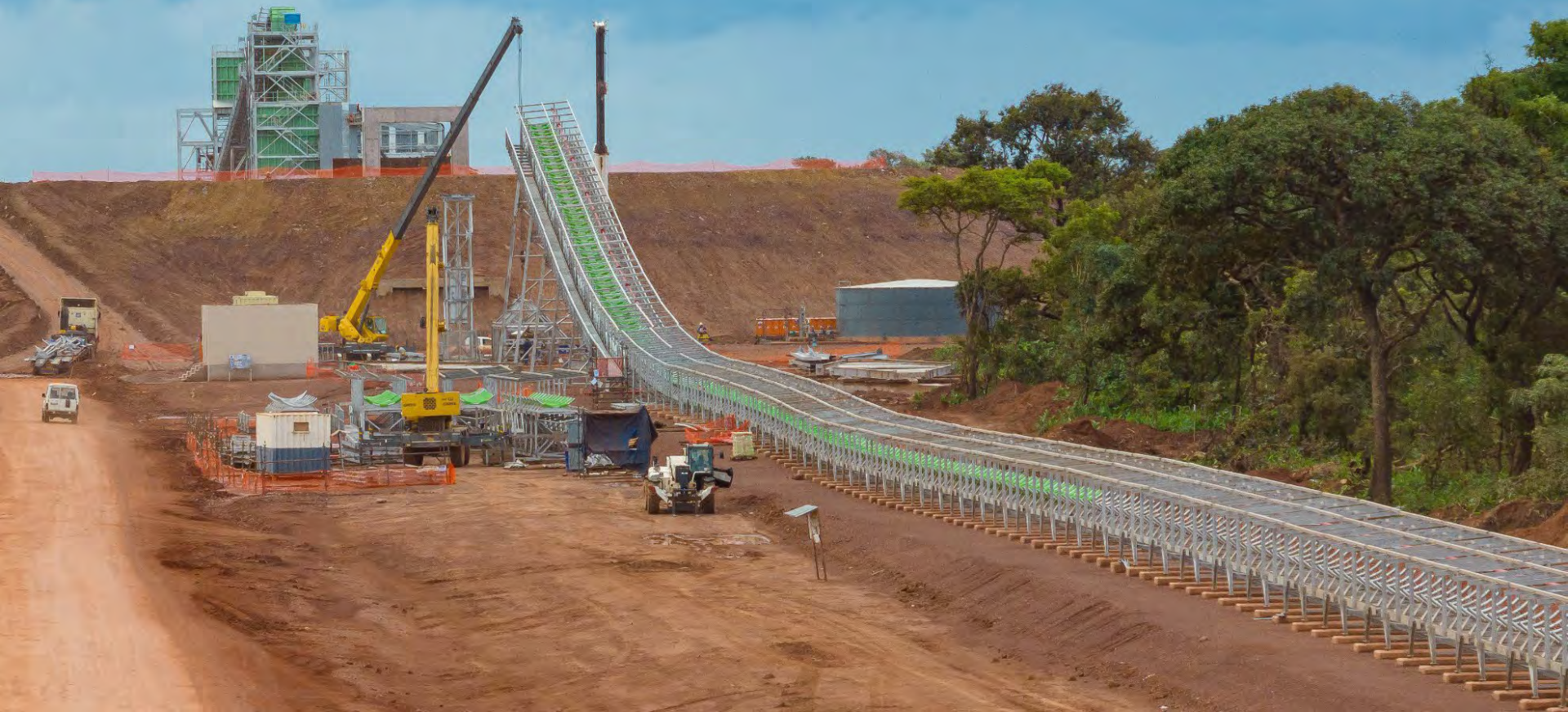
Assembly of the conveyor to Kamoa-Kakula's Phase 3 run-of-mine ore stockpile.
