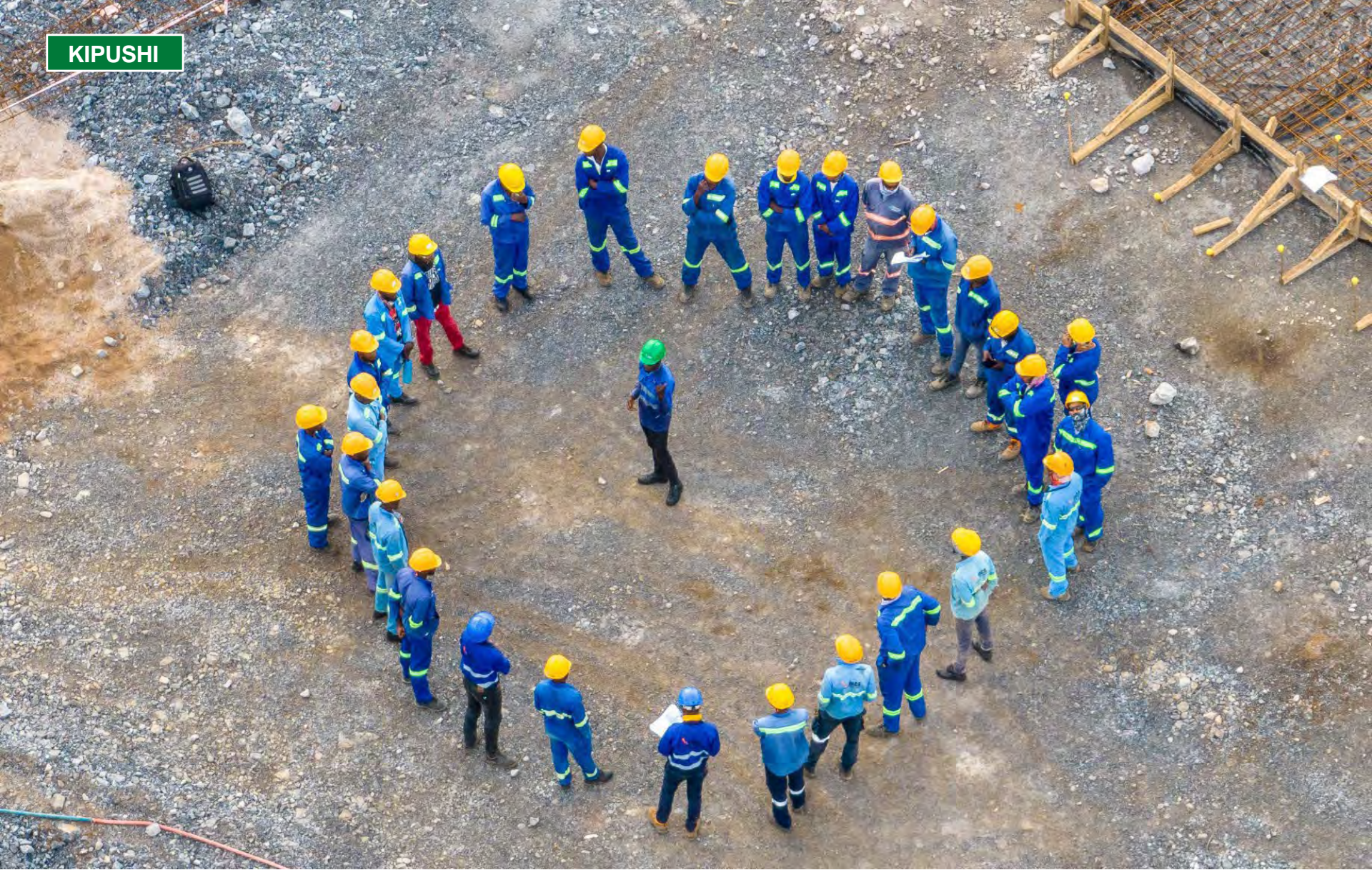
A morning safety share meeting is conducted with Kipushi construction surface crew.
