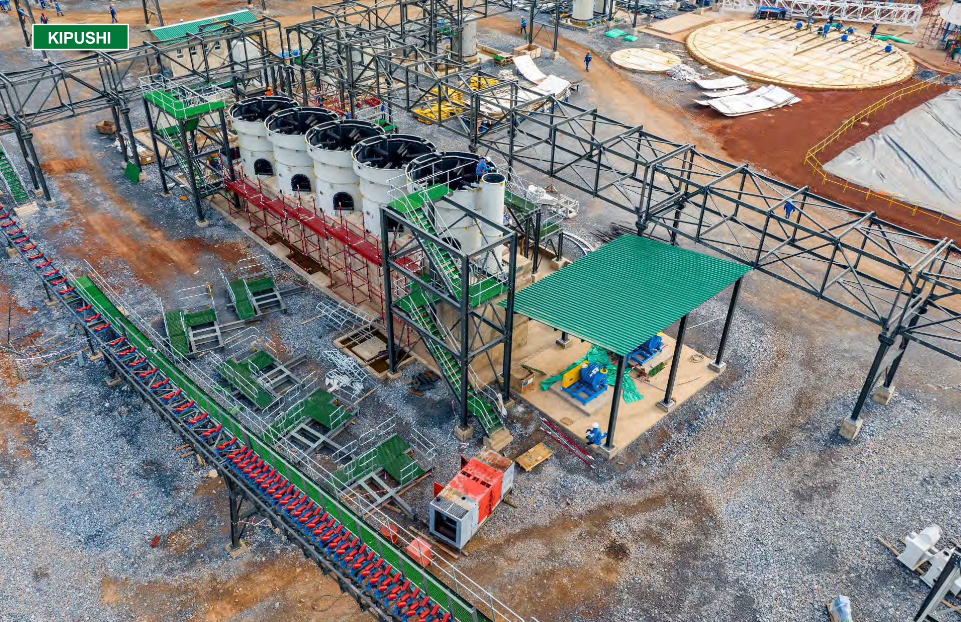
Float cell installation at the Kipushi concentrator.
