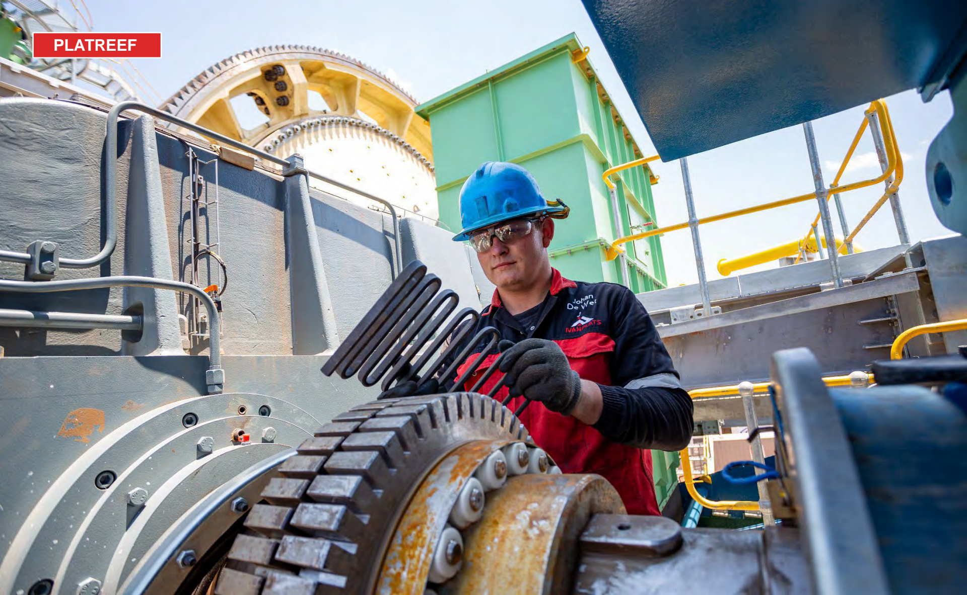
Ivanplats fitter, Johan de Wet, working on a motor and gearbox at the Platreef concentrator.
