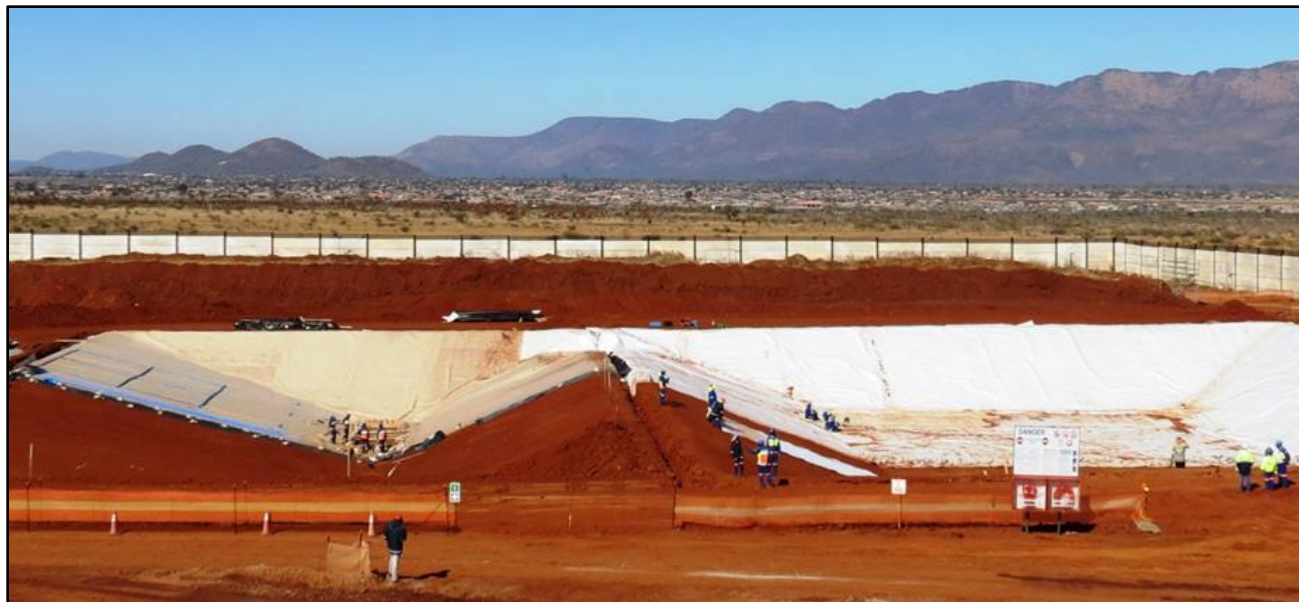
Figure 7: Construction of the lined storm-water pond.
