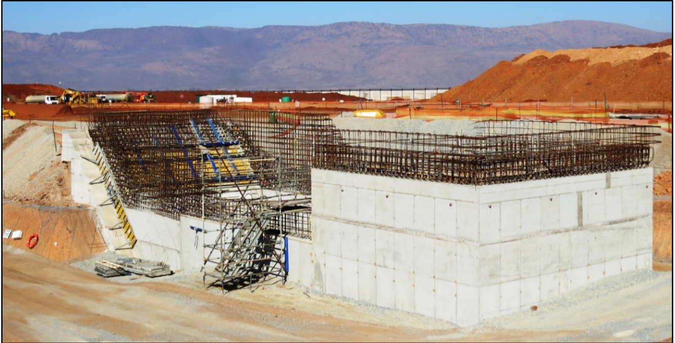
Figure 3: Shaft 1 collar and ventilation plenum construction, July 2015.
