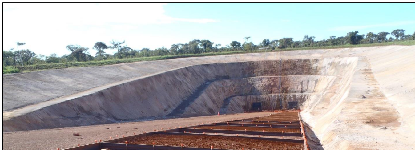
Figure 1: Completed box cut with access roadway under construction.
