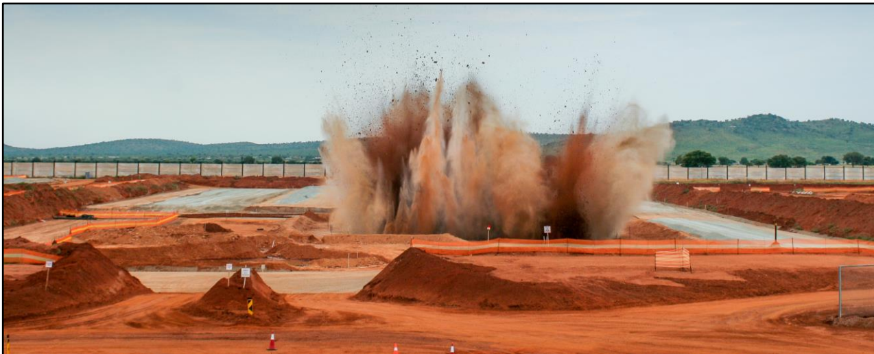
Figure 3: Shaft 1 box cut first blast.
