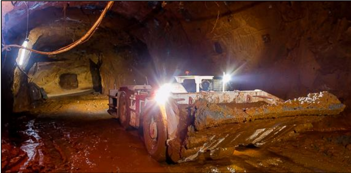
Figure 9: Underground tunnel upgrading work.
