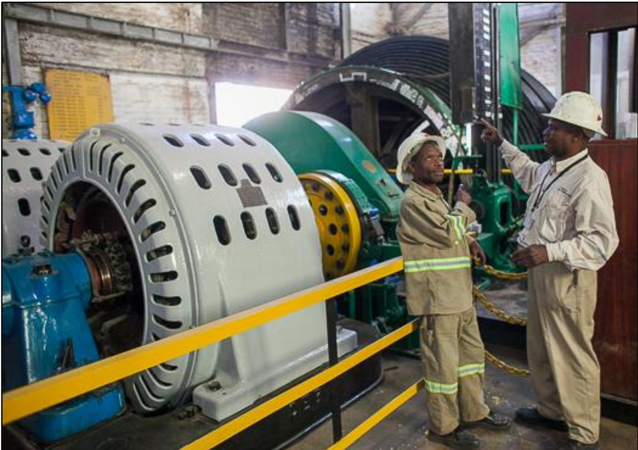
Figure 8: Refurbished shaft equipment.
