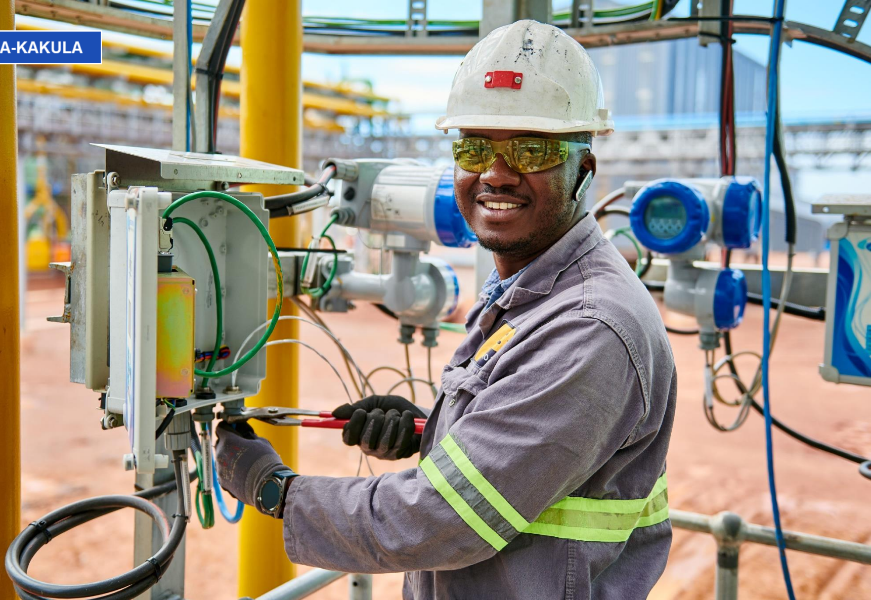
Electrician Tendai Hove terminating electrical cables at the Phase 2 concentrator plant.
