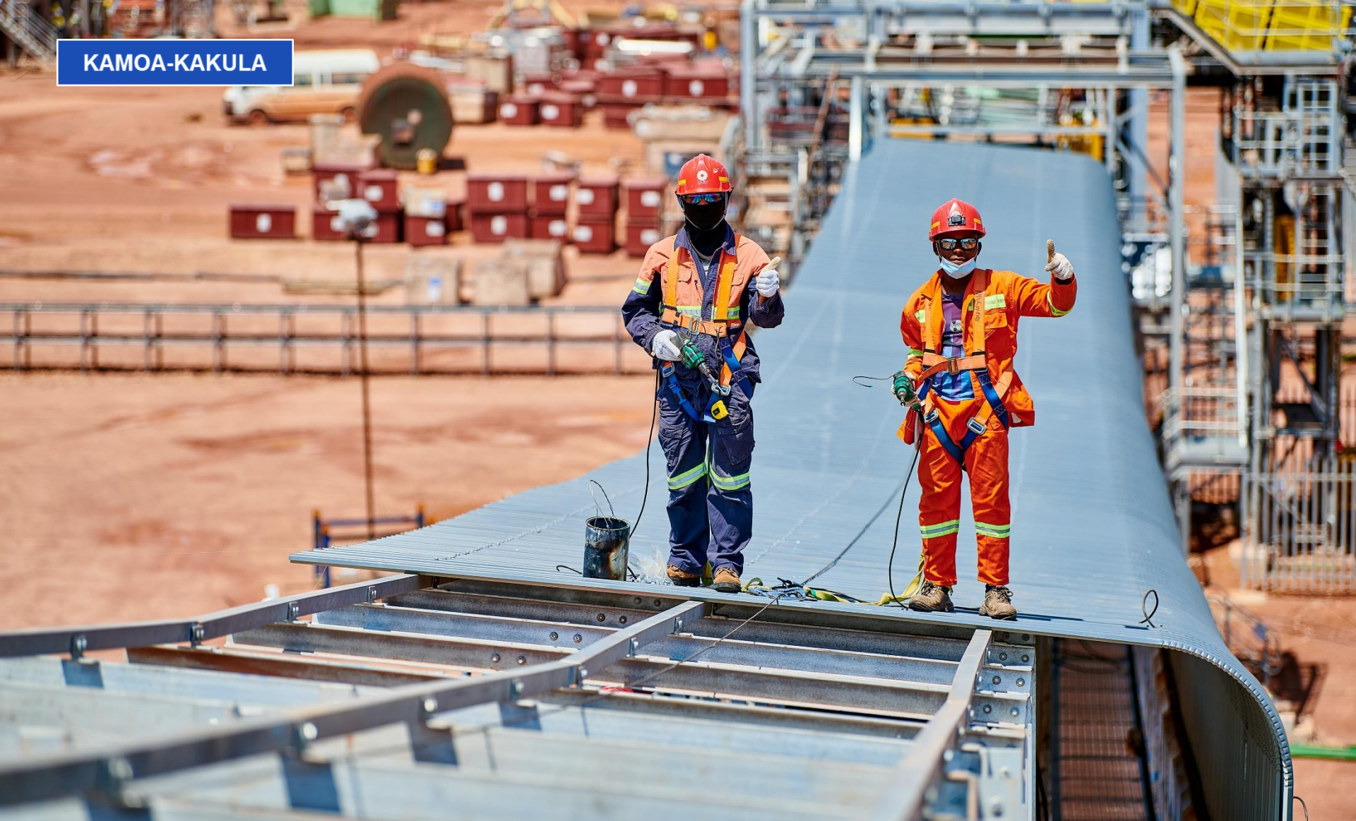
Wu Xingbao (left) and Maride Masiba installing roof paneling over one of the Phase 2 conveyor belts.
