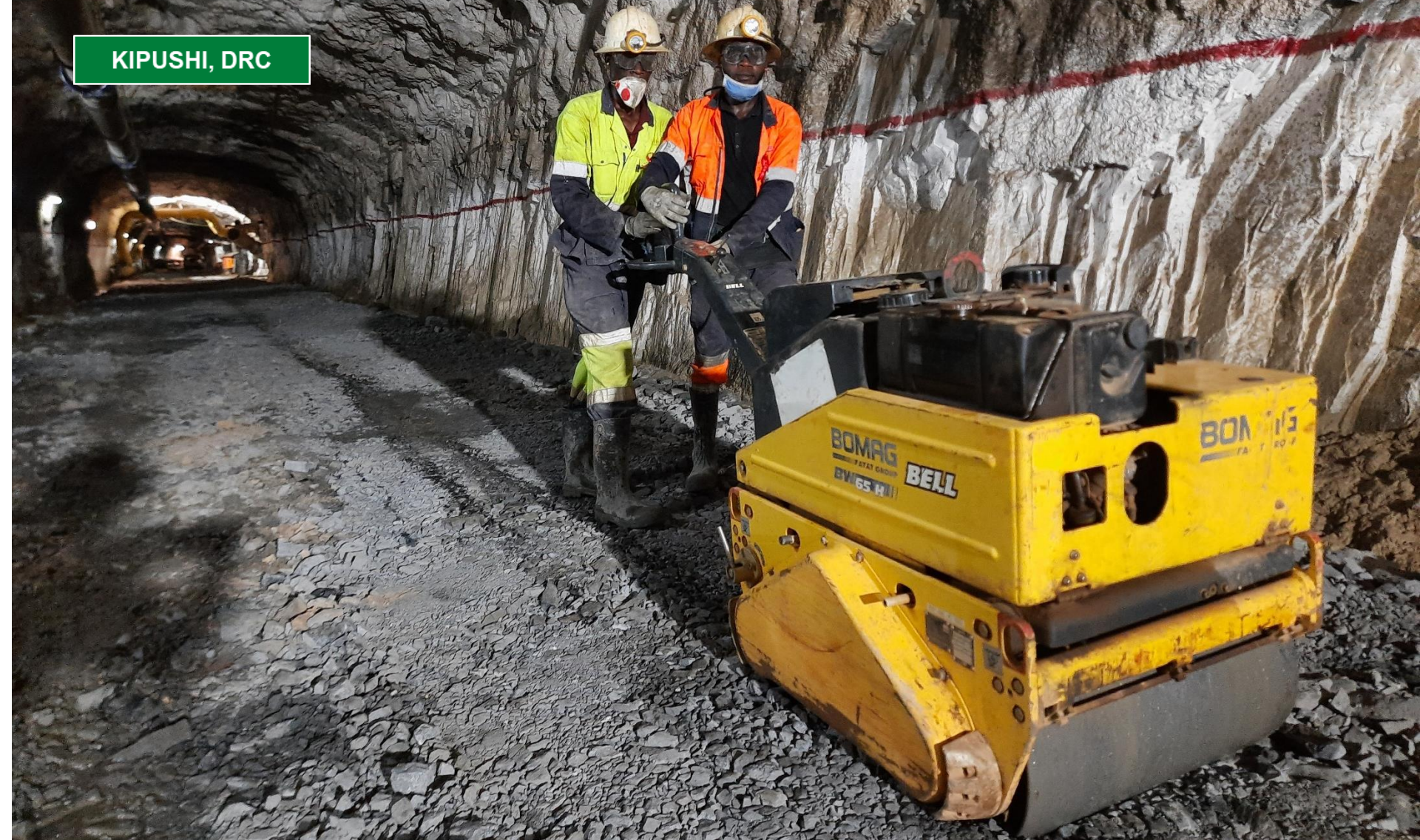
Kasamba (left) and Kanengo compacting and leveling the main ore haulage roadway leading to Kipushi's Big Zinc orebody.
