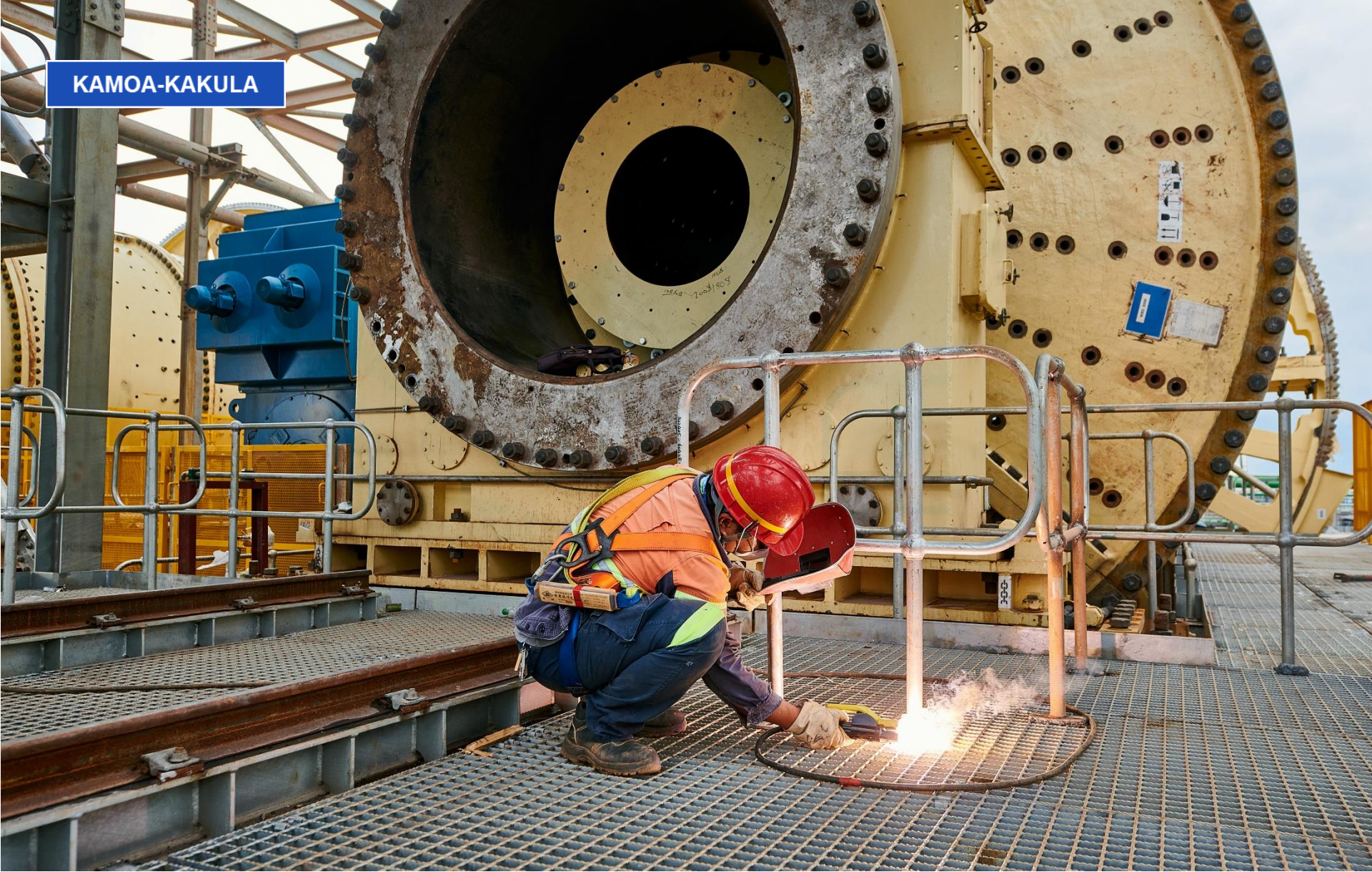
Xie WeiWei welding safety barricades in place at the discharge end of one of the new Phase 2 ball mills.
