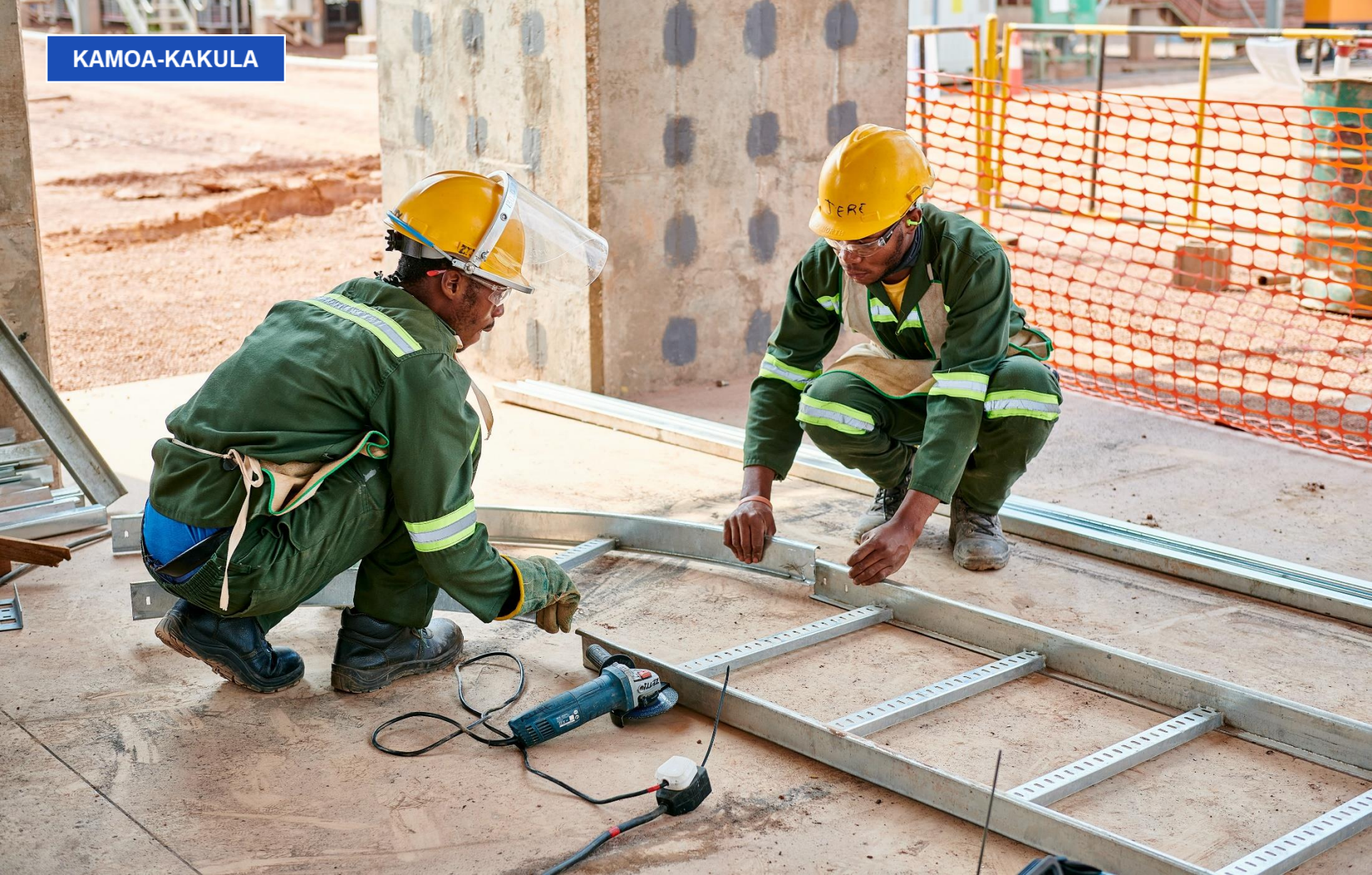
Zetty Musangu Sampind (left) and Jeremie Tshikwej assembling electrical cable racks for the Phase 2 concentrator plant.
