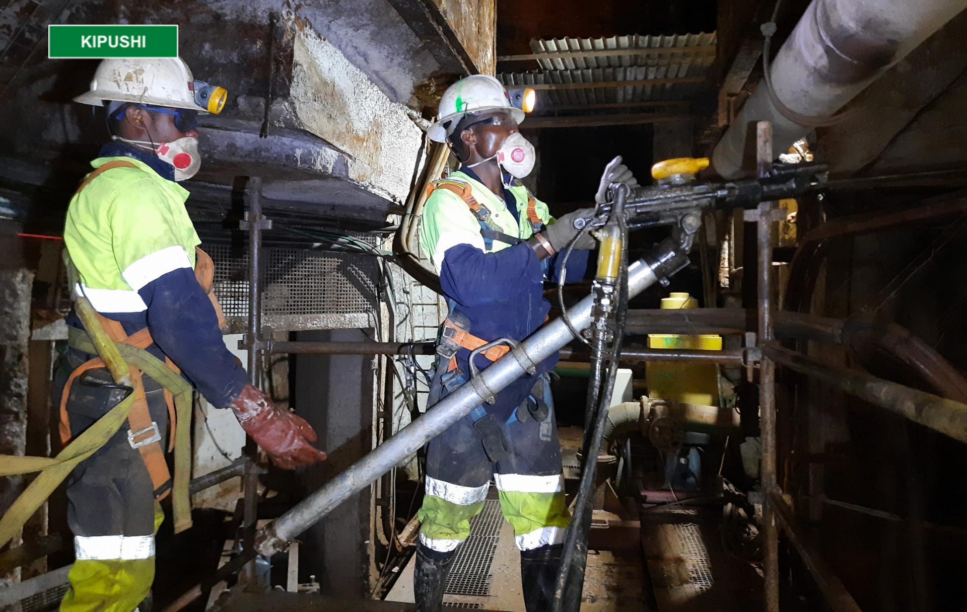
Miners Gael Shimatu (left) and Dela Mwamba drilling rock-bolt holes on Kipushi's 1,138-metre level to support pipes carrying water to surface from newly installed Peerless pumps.
