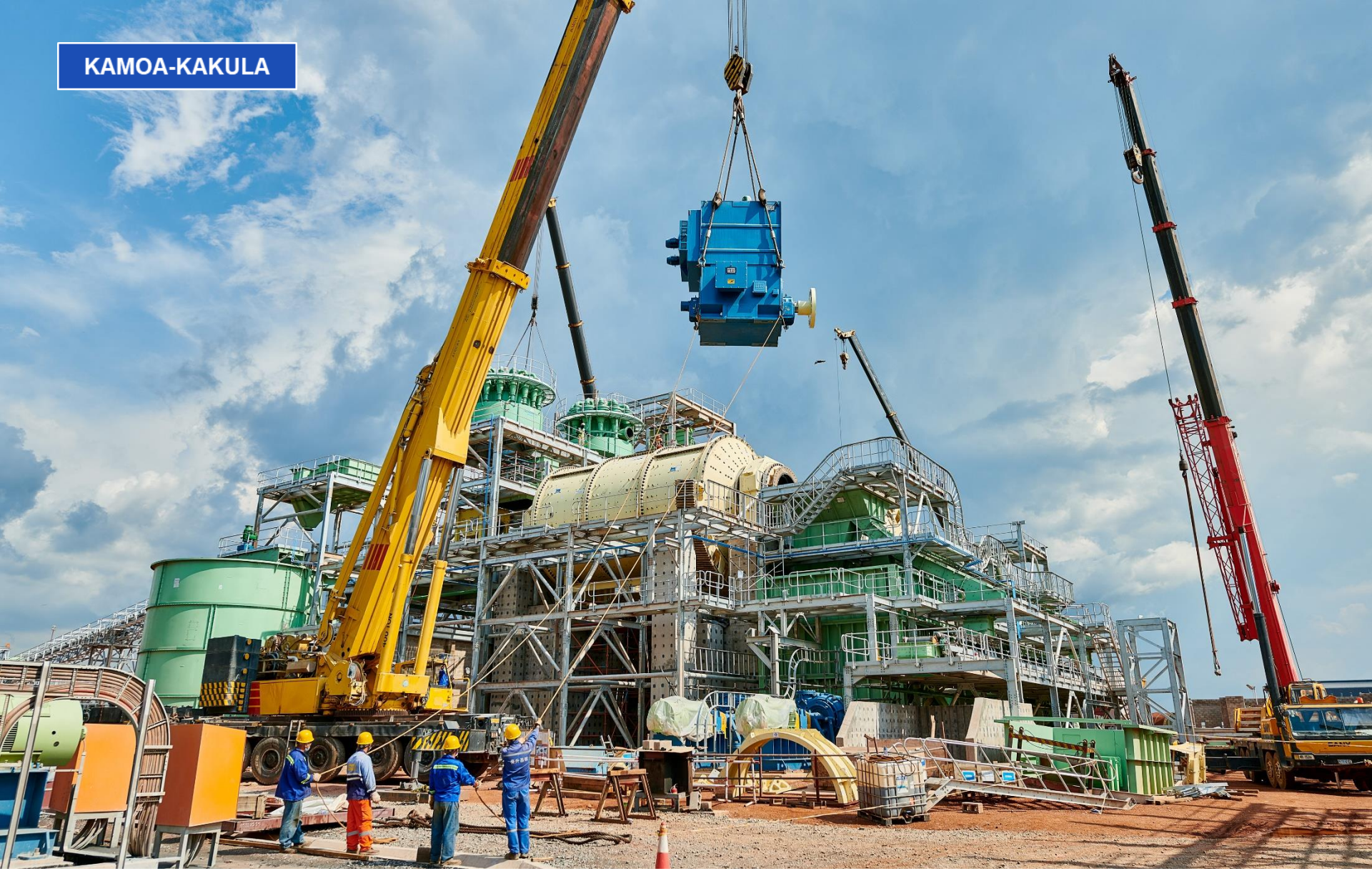
A 400-tonne crane lifting one of the 7-megawatt, variable-speed-drive Phase 2 ball mill motors. The motors were manufactured in Brazil by WEG Industries.
