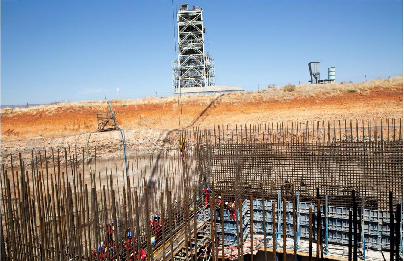
**Platreef's Shaft 2 will have a finished and concrete-lined internal diameter of 10 metres and be sunk to a planned, final depth of 1,104 metres below surface.**
