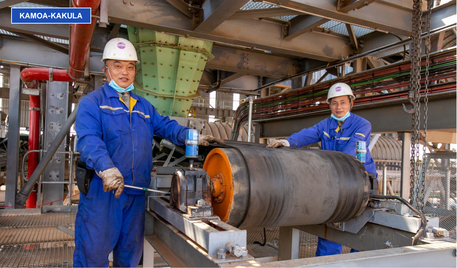
Mechanical Fitters Xuan Zhen Gang (left) and Zhang Yunfu, with Beijing-based CITIC Construction, adjusting a conveyor belt at Kamoa-Kakula's backfill plant, which is being commissioned.
