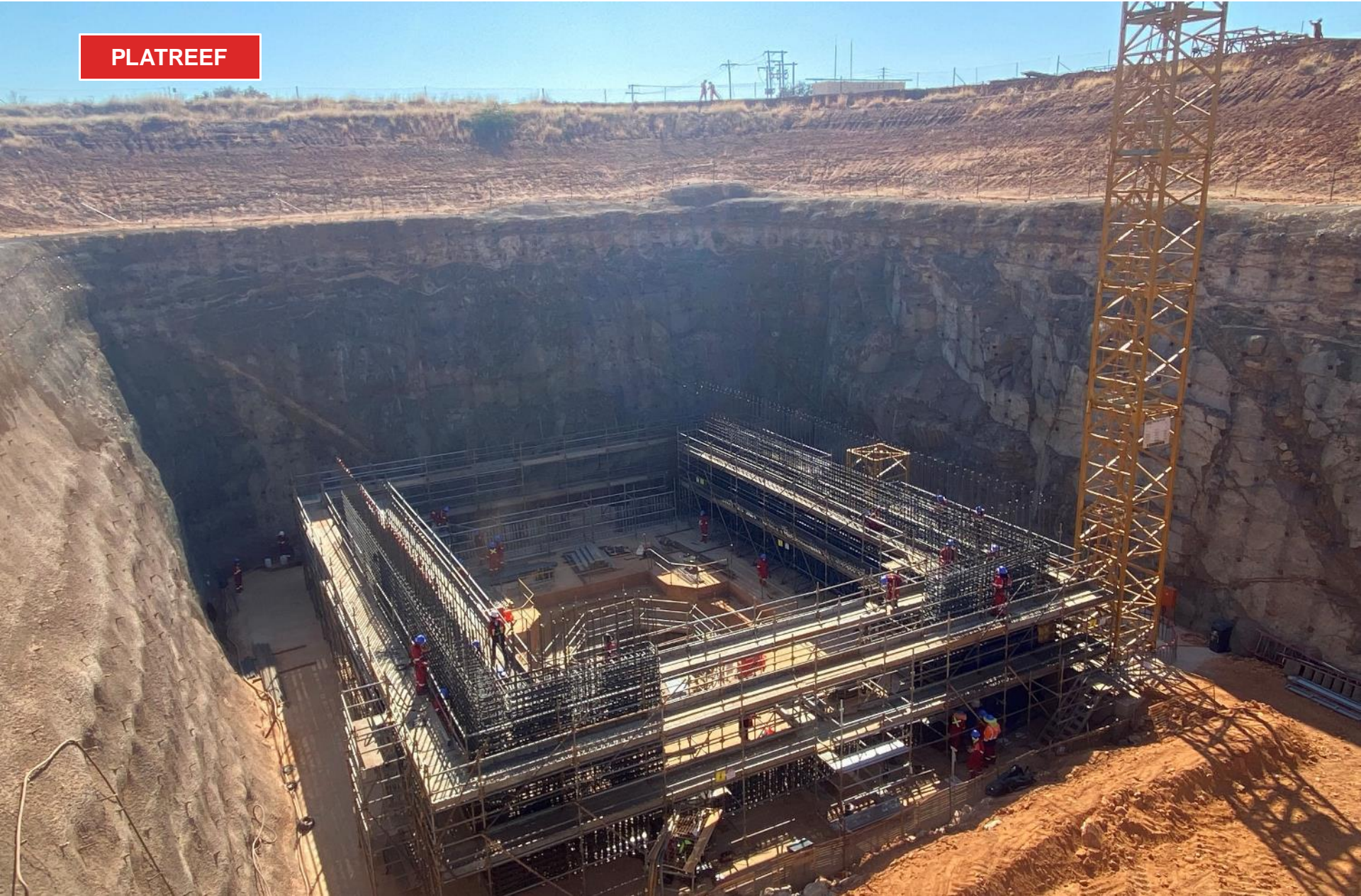
A closer look at the construction work at Shaft 2, which is raising the headframe foundations to surface.
