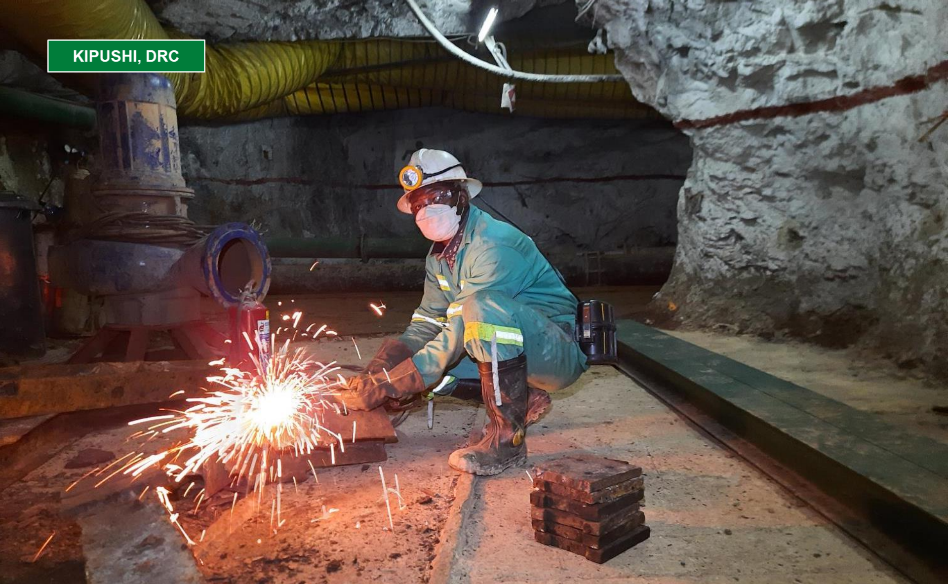
Bulunga Silas, Boilermaker, repairing a water pipe in the Kipushi Mine.
