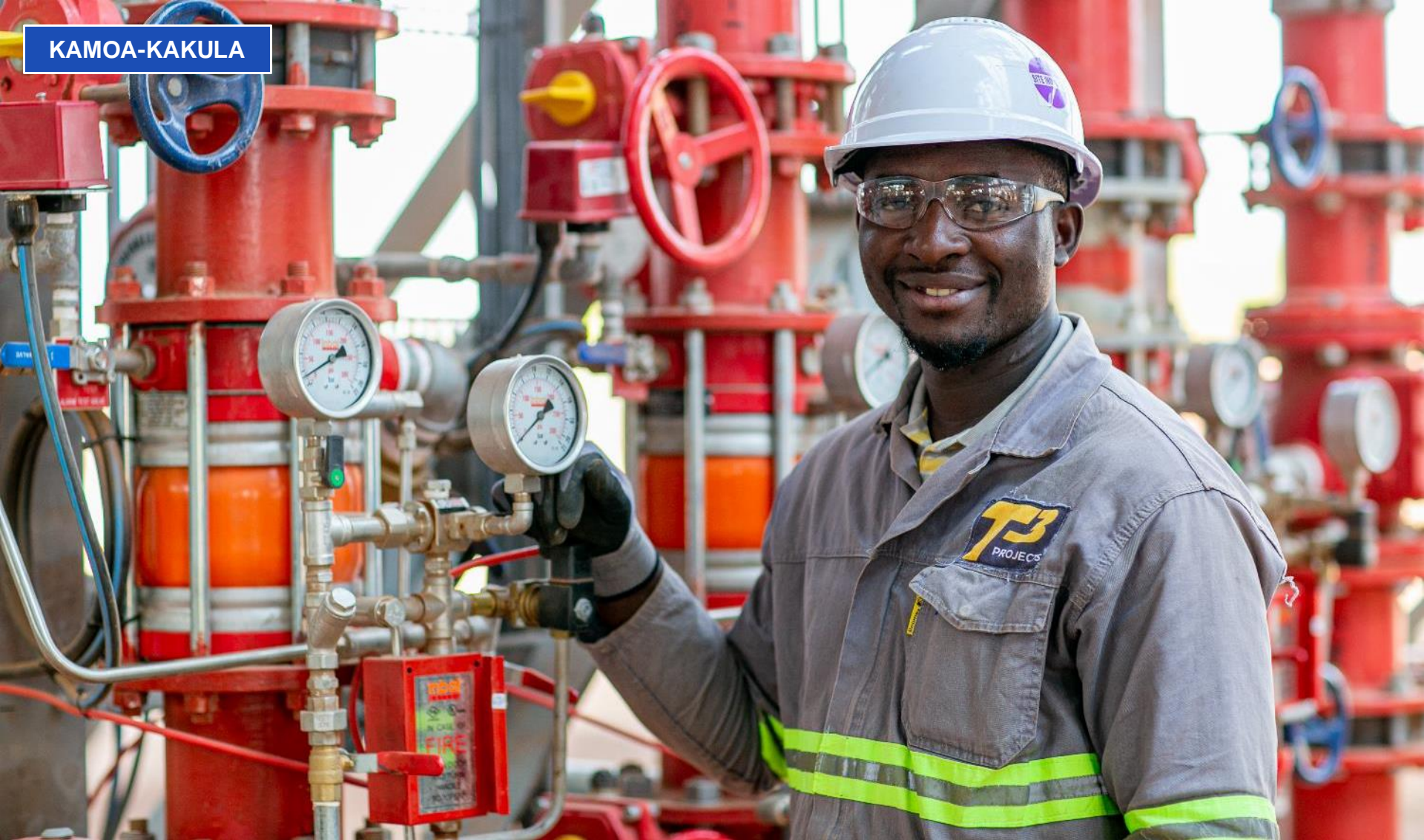
Monga Floribert, Electrician with South Africa-based T3 Projects, monitoring the fire suppression system at the Kakula Phase 1 concentrator plant.
