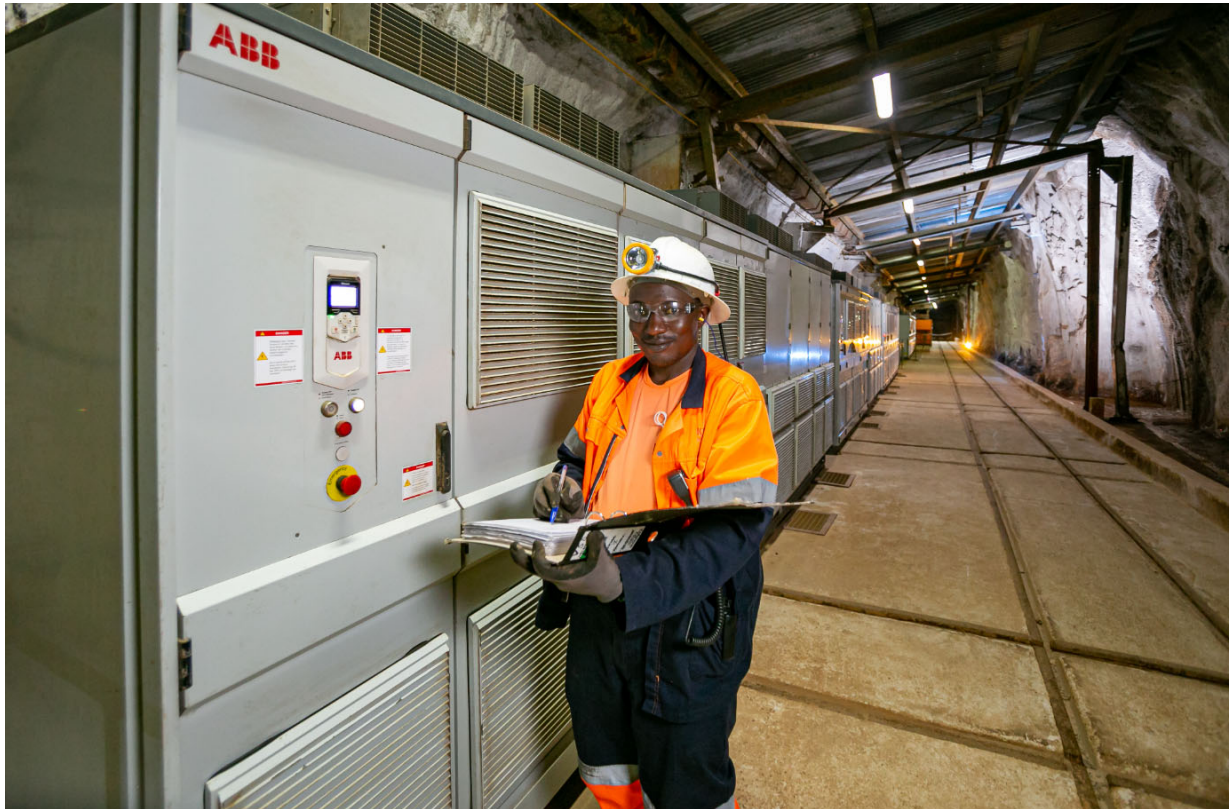
Photo: Cyril Muke checking the variable speed drives for the large-capacity Grifo water pumps that are keeping Kipushi's underground operations dry.
