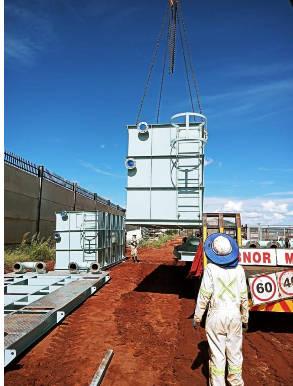
Platreef team members offloading the two water tanks for the permanent shaft-pumping system.
