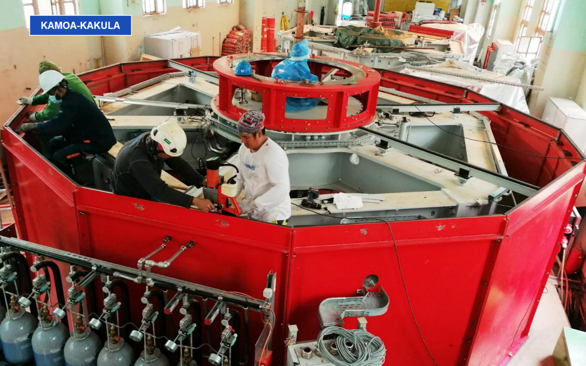
Electricians from Andritz Hydro, of Vevey, Switzerland, installing the alternator for the second of six new turbines at the Mwadingusha hydropower plant.
