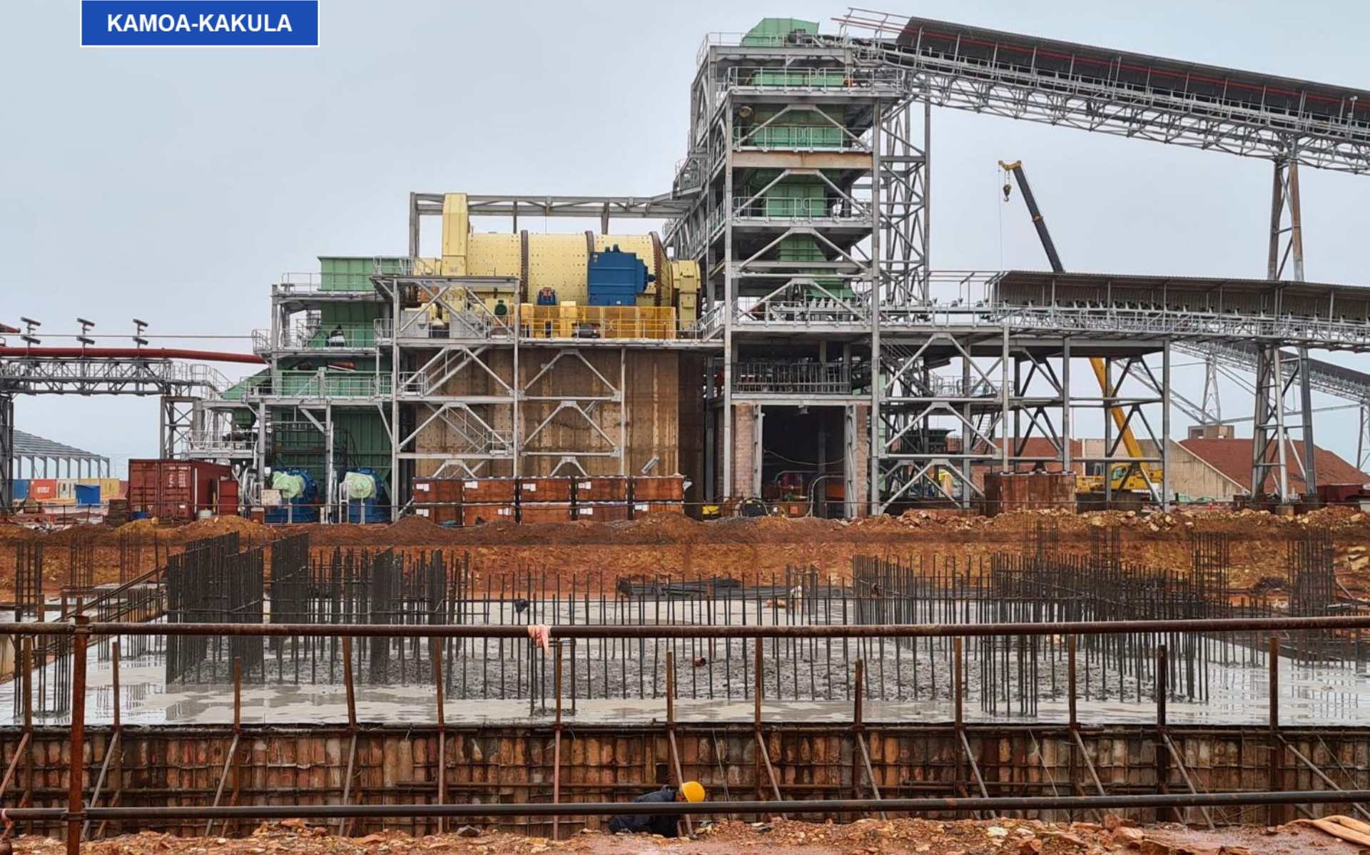
Concrete base poured for Kakula's Phase 2 ball mill foundations.
