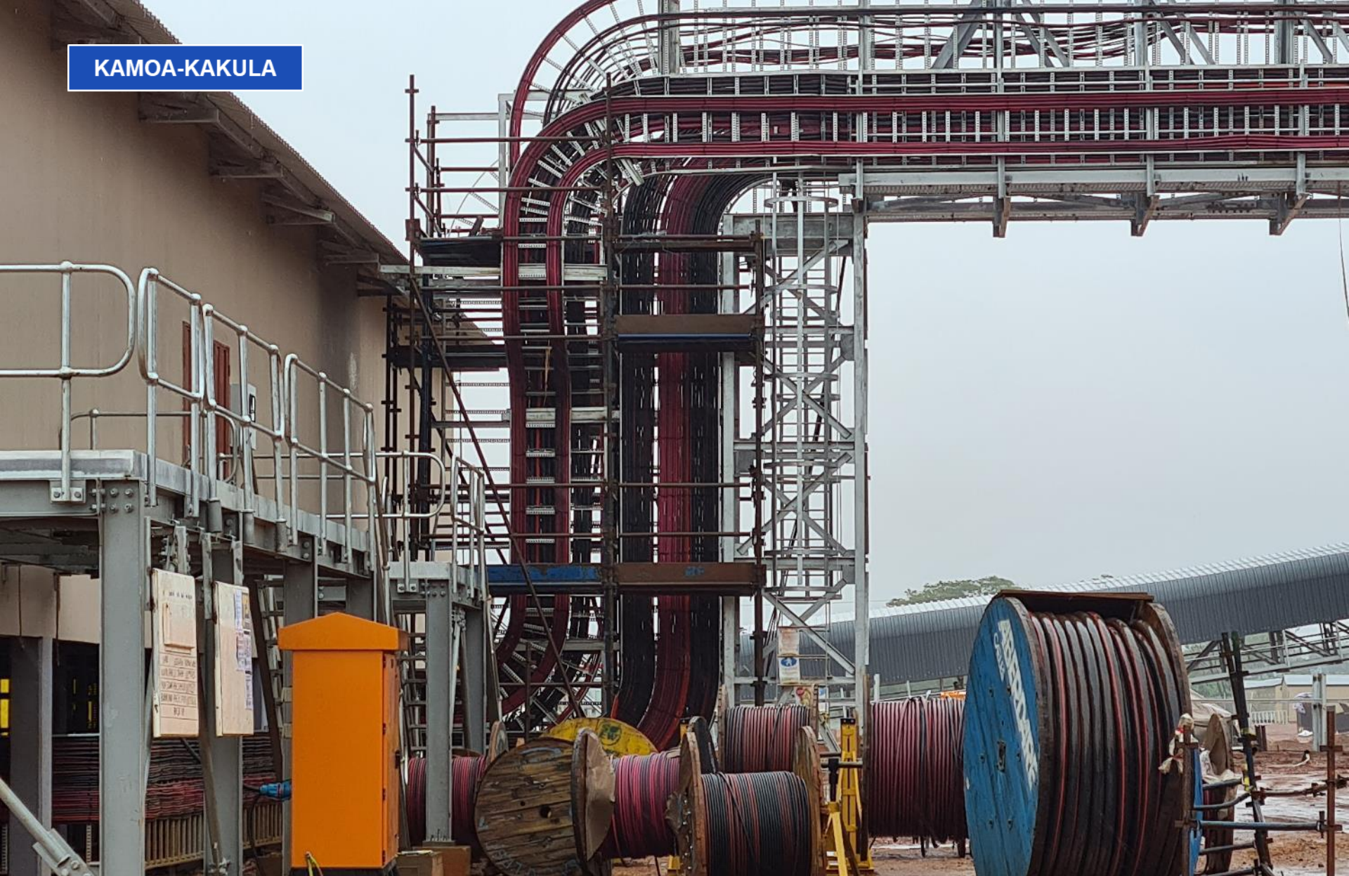
Installation of copper electrical cables at the Phase 1 concentrator.
