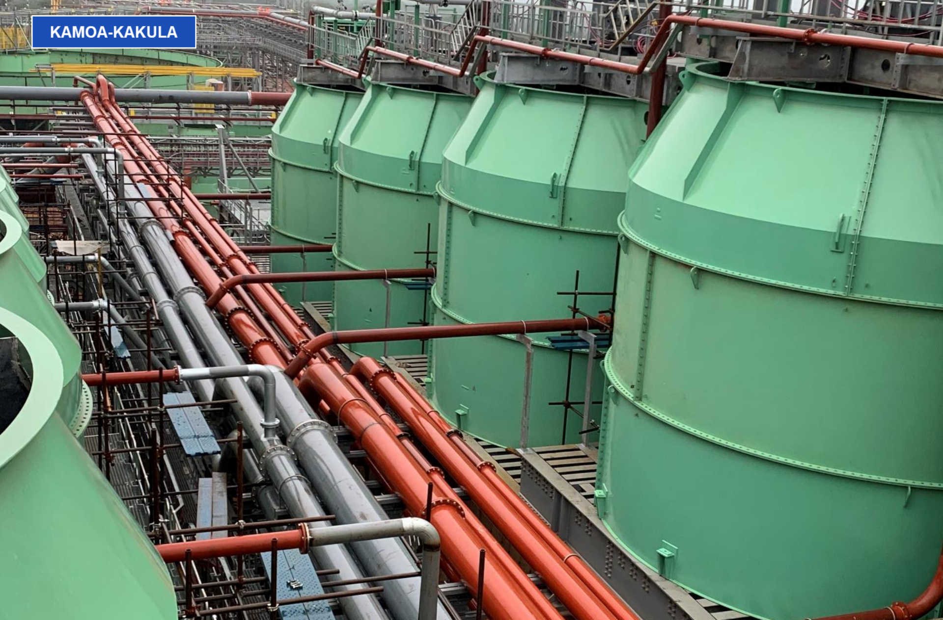
Piping installed for the rougher and cleaner flotation cells at Kakula's Phase 1 concentrator.
