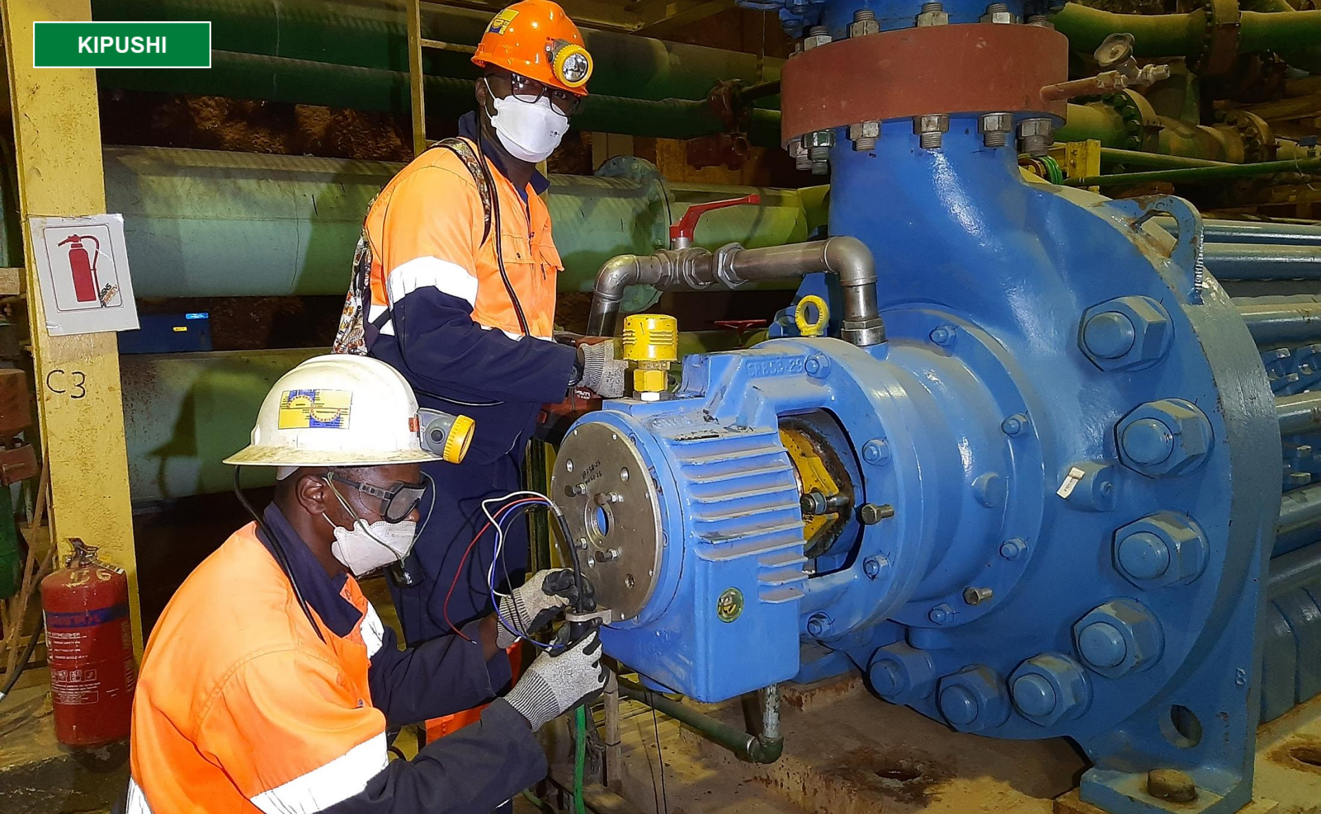
Kyungu Kabulo, Instrumentation assistant (left); and Junior Kisula Ngoy, Instrumentation Engineer (right), installing probes and a balance disk on a Grifo Pump at Kipushi's 1,200-metre pumping station.
