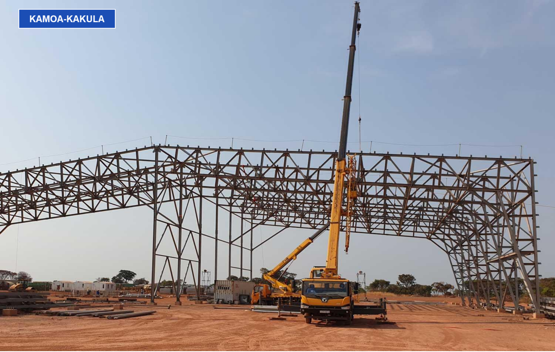
Construction of Kamoa-Kakula's copper concentrate storage building.
