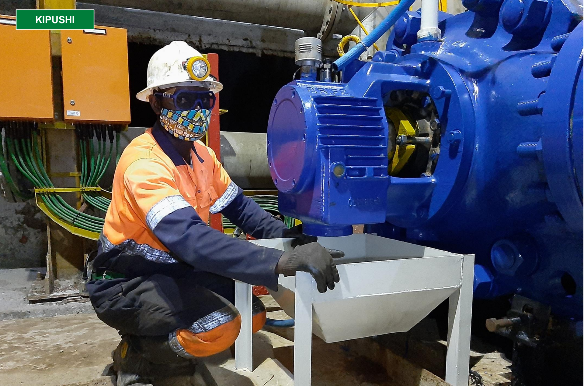
Mr. Samy installing a water collector on the Grifo pump no. 1 at the 850-metre level pumping station.
