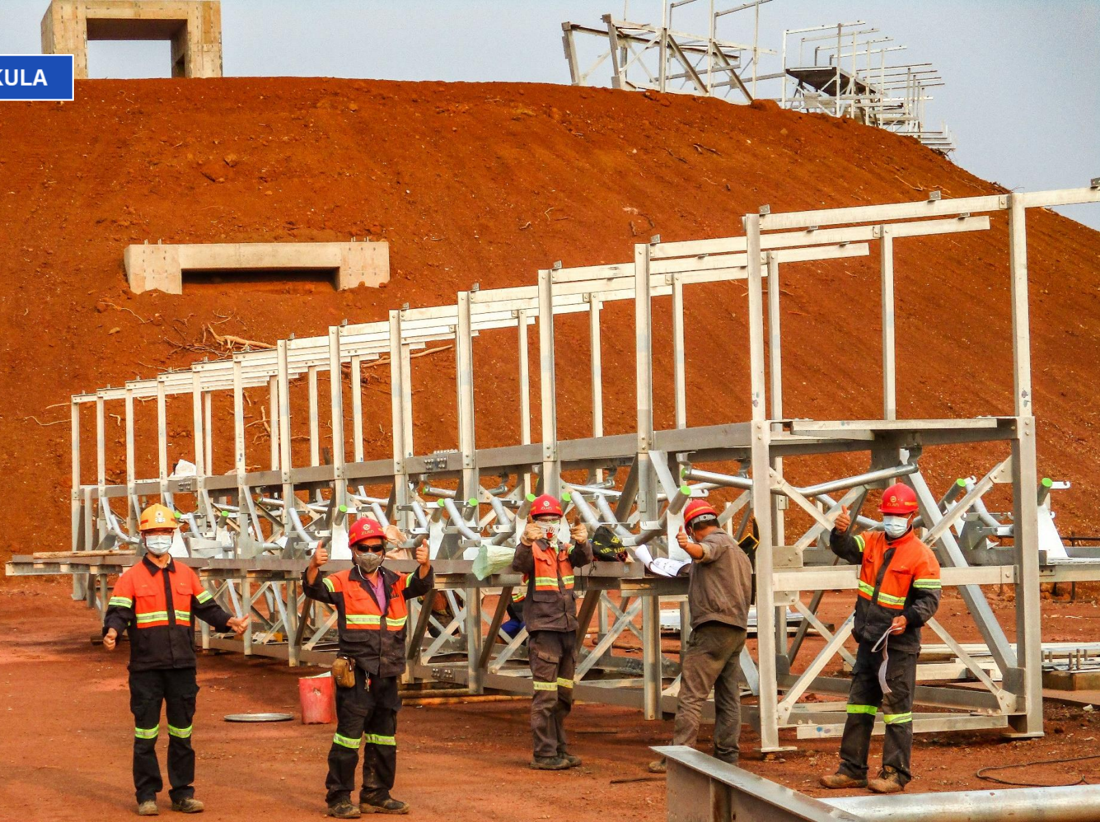
Construction workers assembling the conveyor feeder system for the processing plant's high-pressure grinding rolls.
