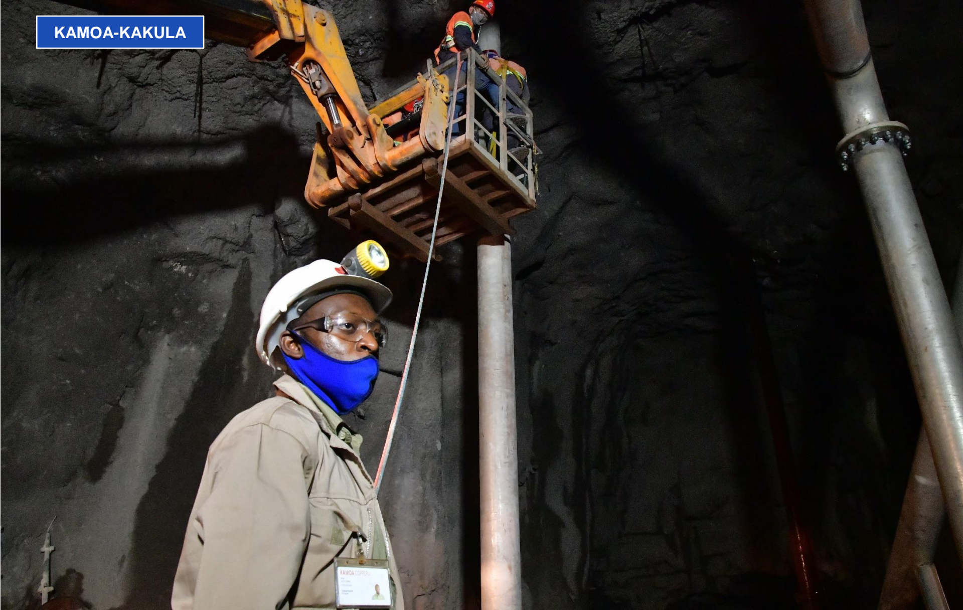
Abel Muyumba, Kamoia Technical Coordinator, supervising the installation of piping to carry water from Kakula's room-and-pillar underground dam to surface settling ponds.
