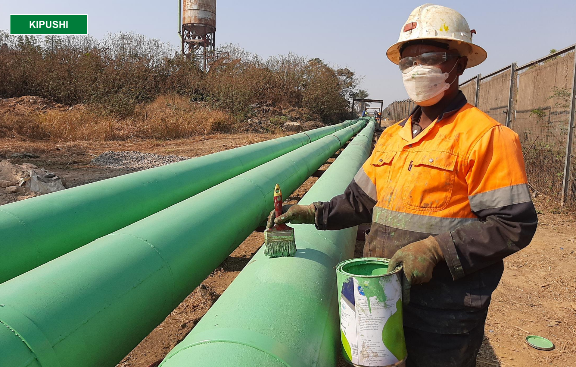
Kamanda Nyandwe painting new pipes carrying clean water from Kipushi's underground pumping station to surface settling ponds.
