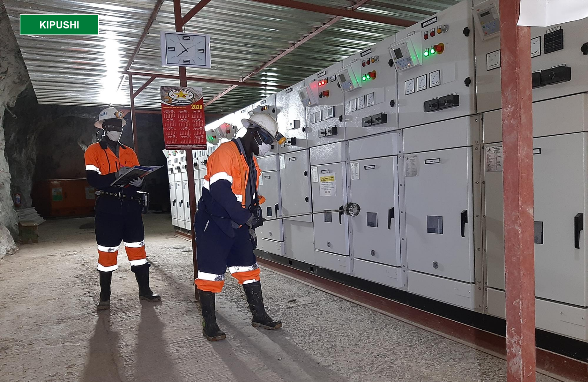
Samuel Ndembo (left) and Mbiya Africa (right) taking air flow measurements at Kipushi's 850-metre-level electrical substation.
