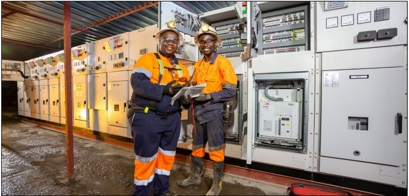
Photo: Prince Kaomba, Electrician (left), and Paul Dikwenda, Mining Manager (right), inspecting diagrams of the 17.5-megawatt variable speed drives for the five high-volume water pumps installed on Kipushi's 1,200-metre level.
