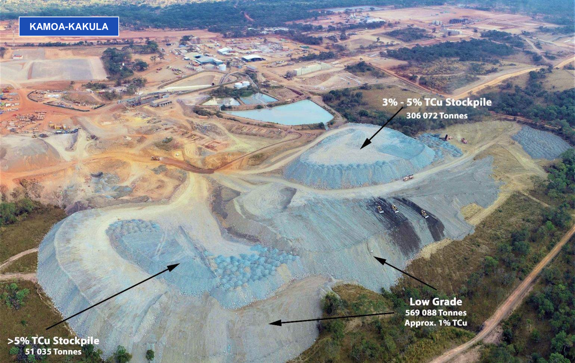
Aerial view of the Kakula Mine showing the tonnes and grade of the pre-production stockpiles. The main declines are in the center of the picture and the processing plant in the upper right corner.
