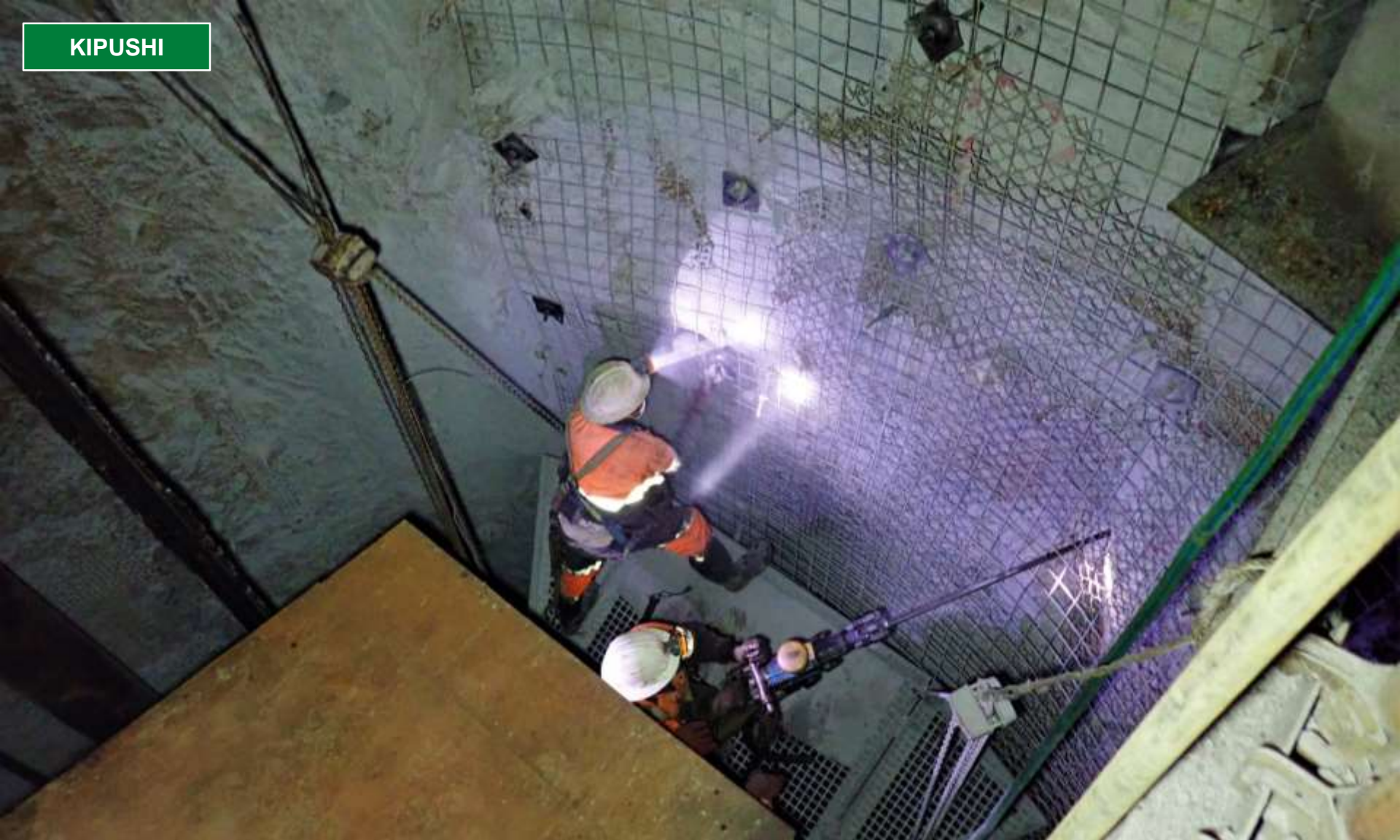
Miners Mpoyo Lenge (left) and Katende Muya (right) supporting shaft sidewalls with welded mesh and rock bolts in Shaft 5 at the 850-metre-level station.
