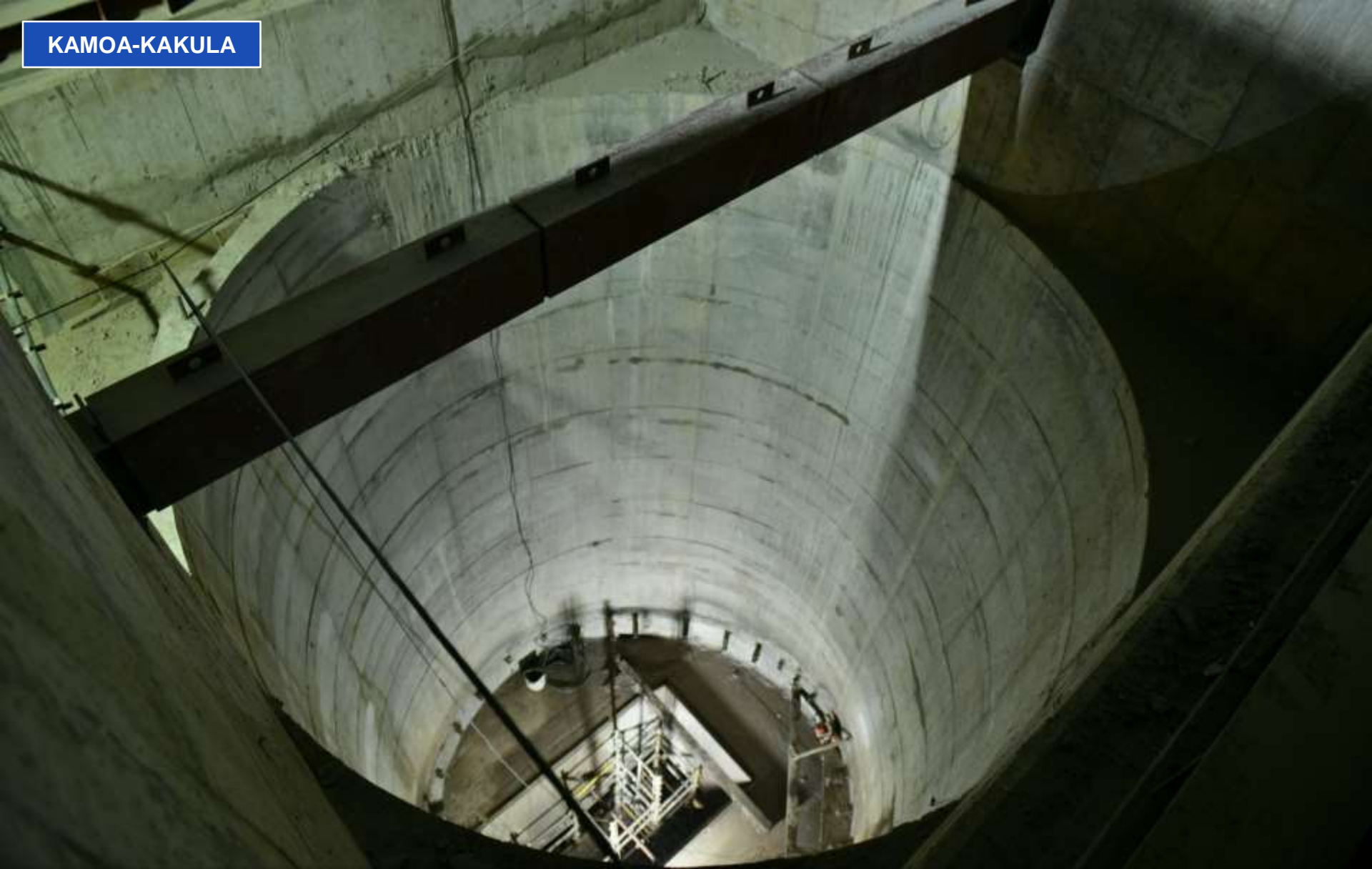
View looking down the east ore bin, one of two 5000-tonne underground ore bins currently being constructed at Kakula.
