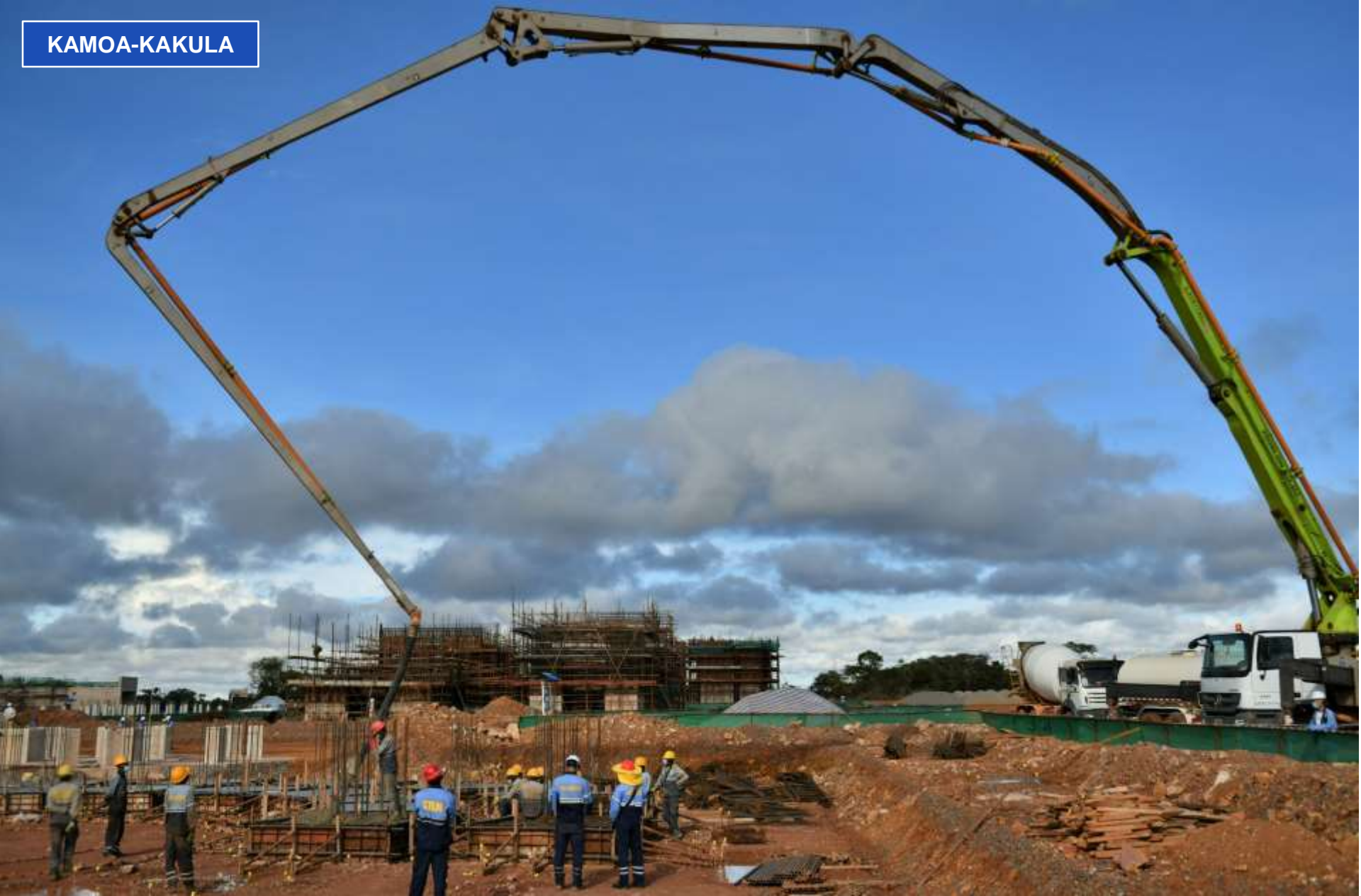
Pouring the concrete foundations for the processing plant's concentrate thickener.
