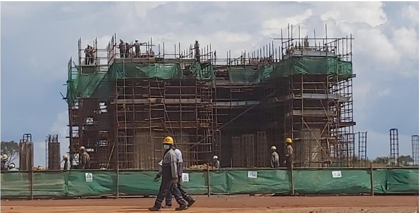
**Pouring the concrete foundations for the processing plant's concentrate thickener.**
