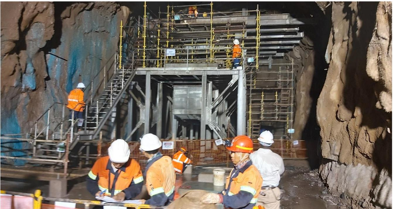
**Raise boring machine breaks through to surface, marking the completion of reaming the 5.5-metre diameter Ventilation Shaft 2 at the Kakula Mine.**
