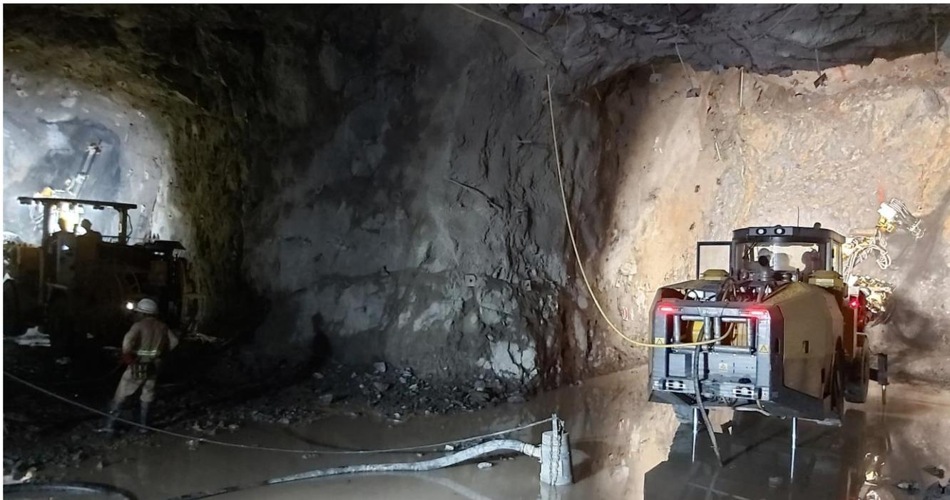
**Construction crew extending the wall at Kakula's main underground water storage dam.**
