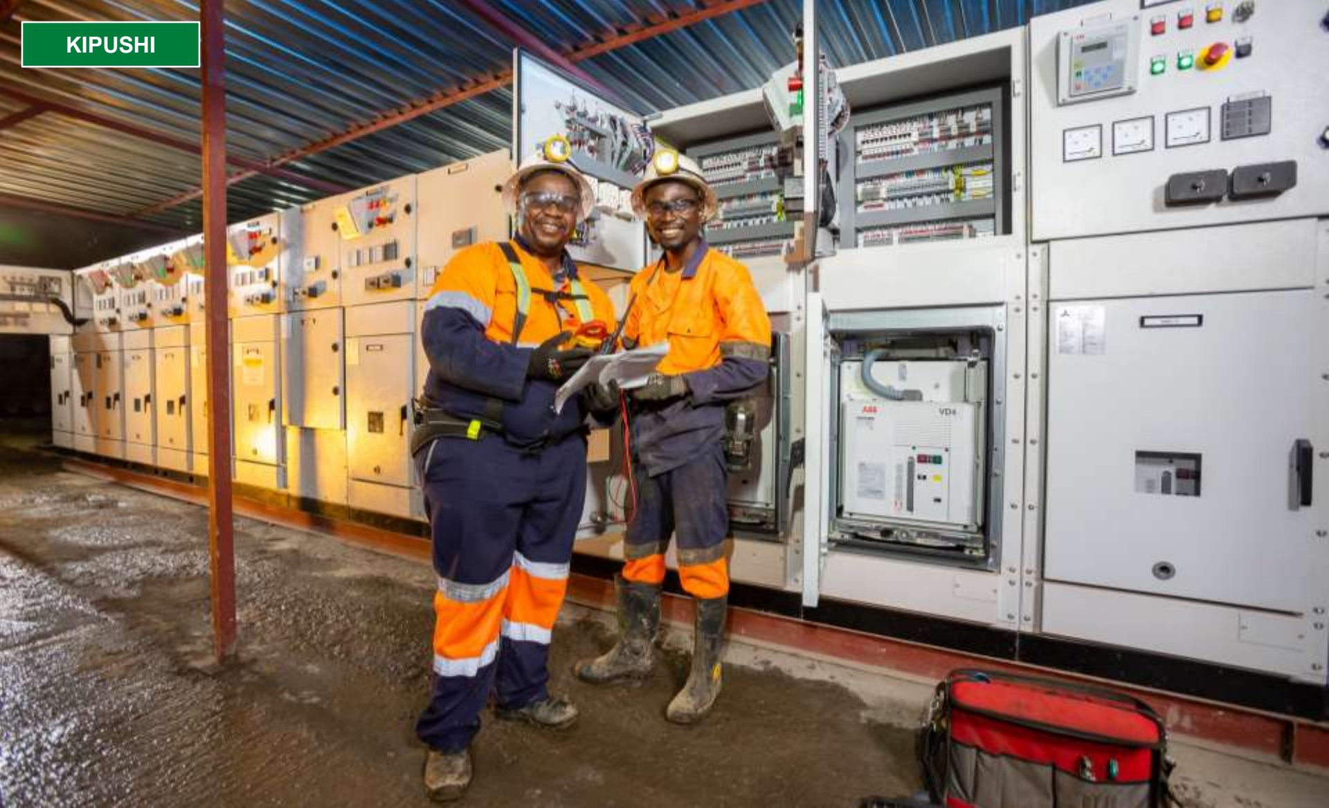
Alfons Molepo, Senior Electrical Foreman (left), discussing the electrical drawings with Tshilay Pascal, Electrician (right), at the newly installed, medium voltage switchgear at the 850-metre-level pump station.
