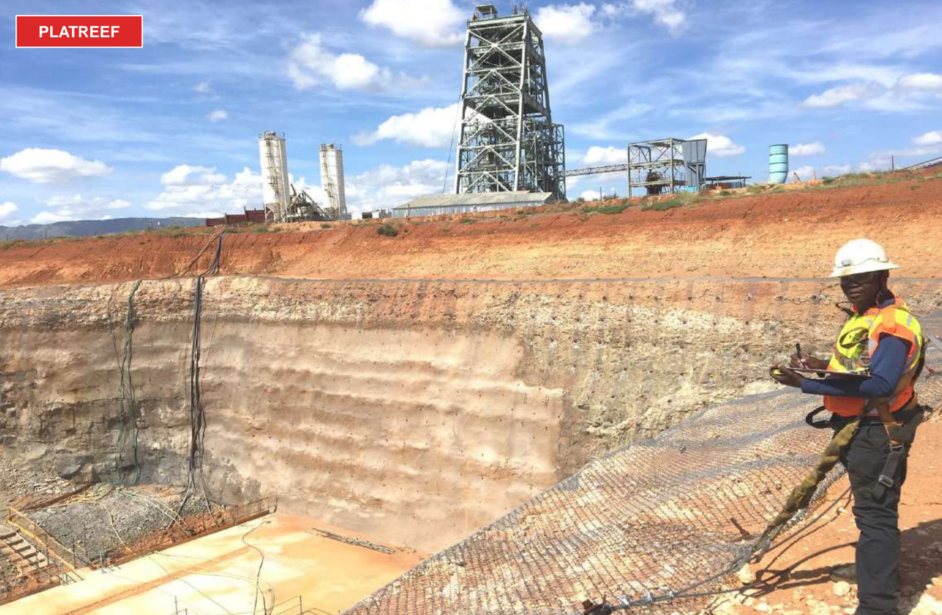
Johannes Nkhoma, Strata Control Observer Trainee, conducting a geotechnical inspection on the 5m bench of the Shaft 2 box cut.
