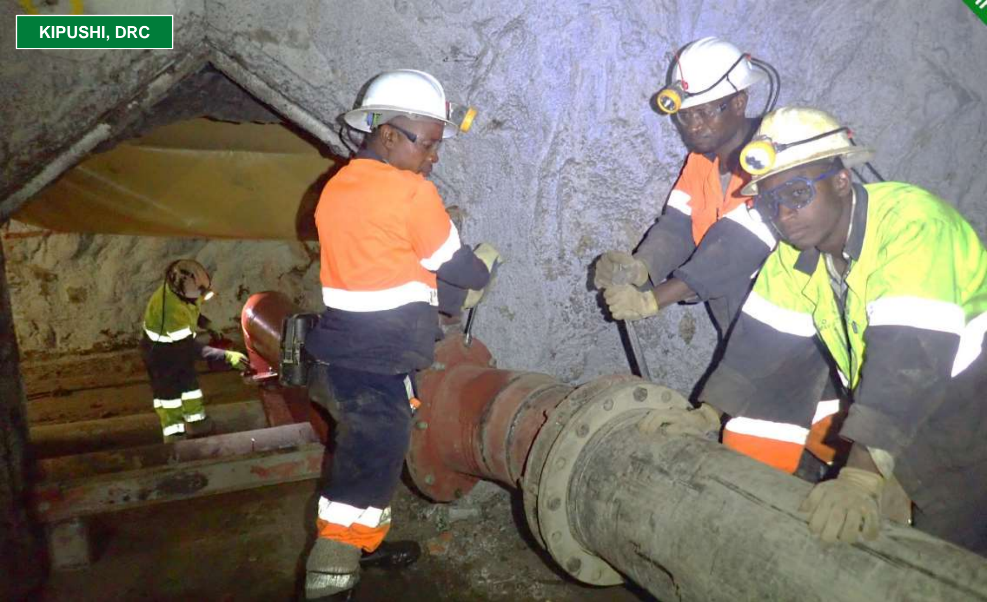
Kamanda, Mario and Henock install a pump column to Kipushi's 850-metre-level pump chamber.
