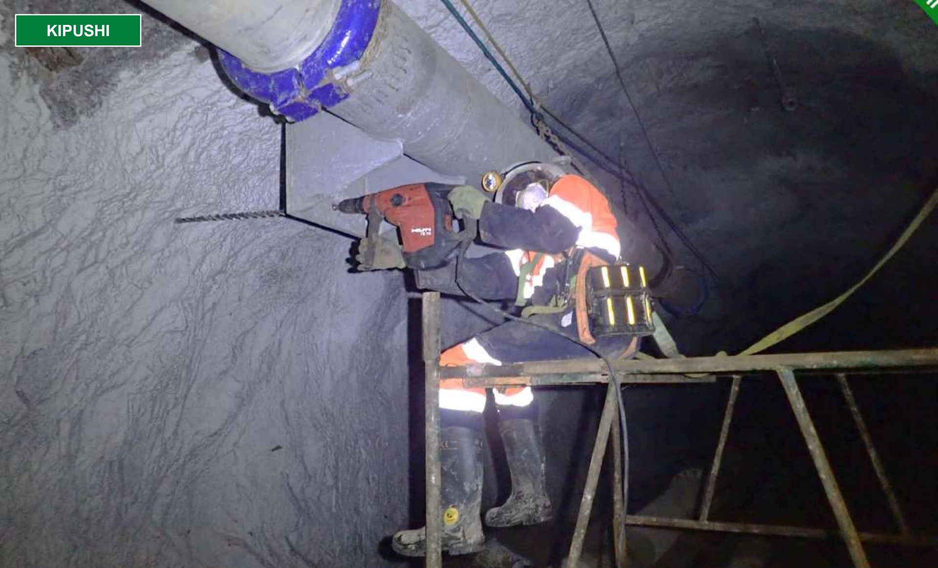
Mpoyo drilling pin holes for support for a water pump column.
