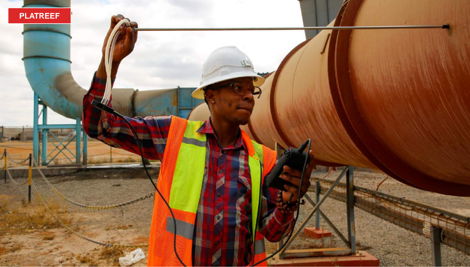
William Makhafola taking air-flow measurements from a ventilation pipe at Platreef's Shaft 1.
