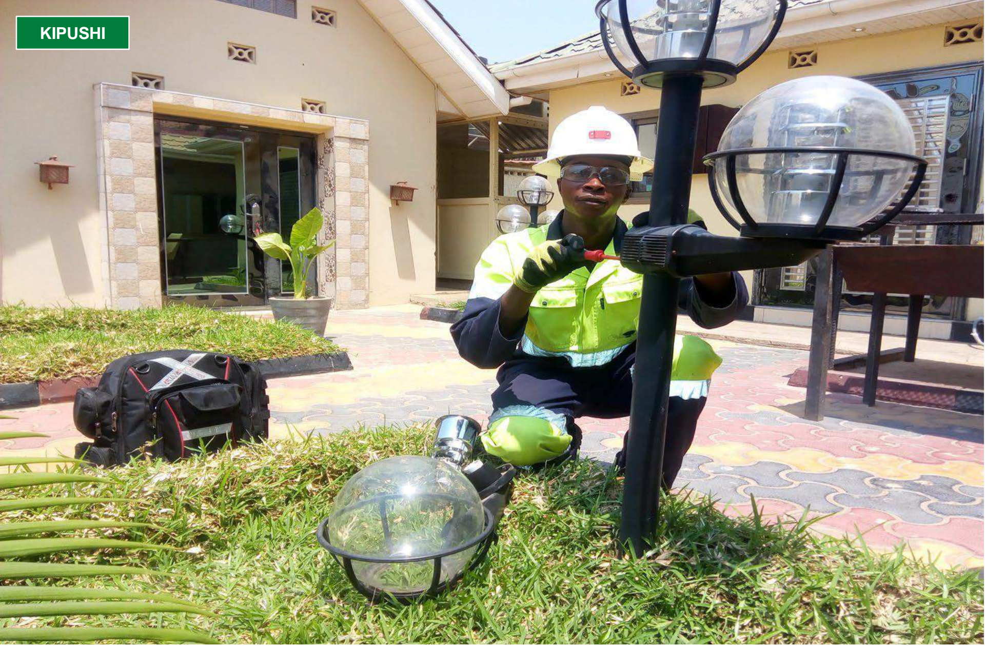
Electrician Ngeleka Elie installing lights at the guest houses at Kipushi.
