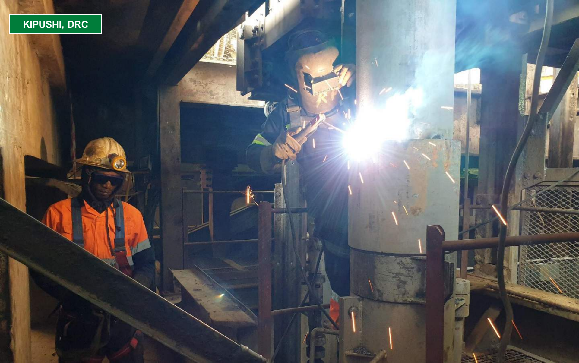
Mulamba Belly (left) and Rudolph Pienaar (right) welding a new water pipe for Kipushi's new pumping station at the 850-metre level.
