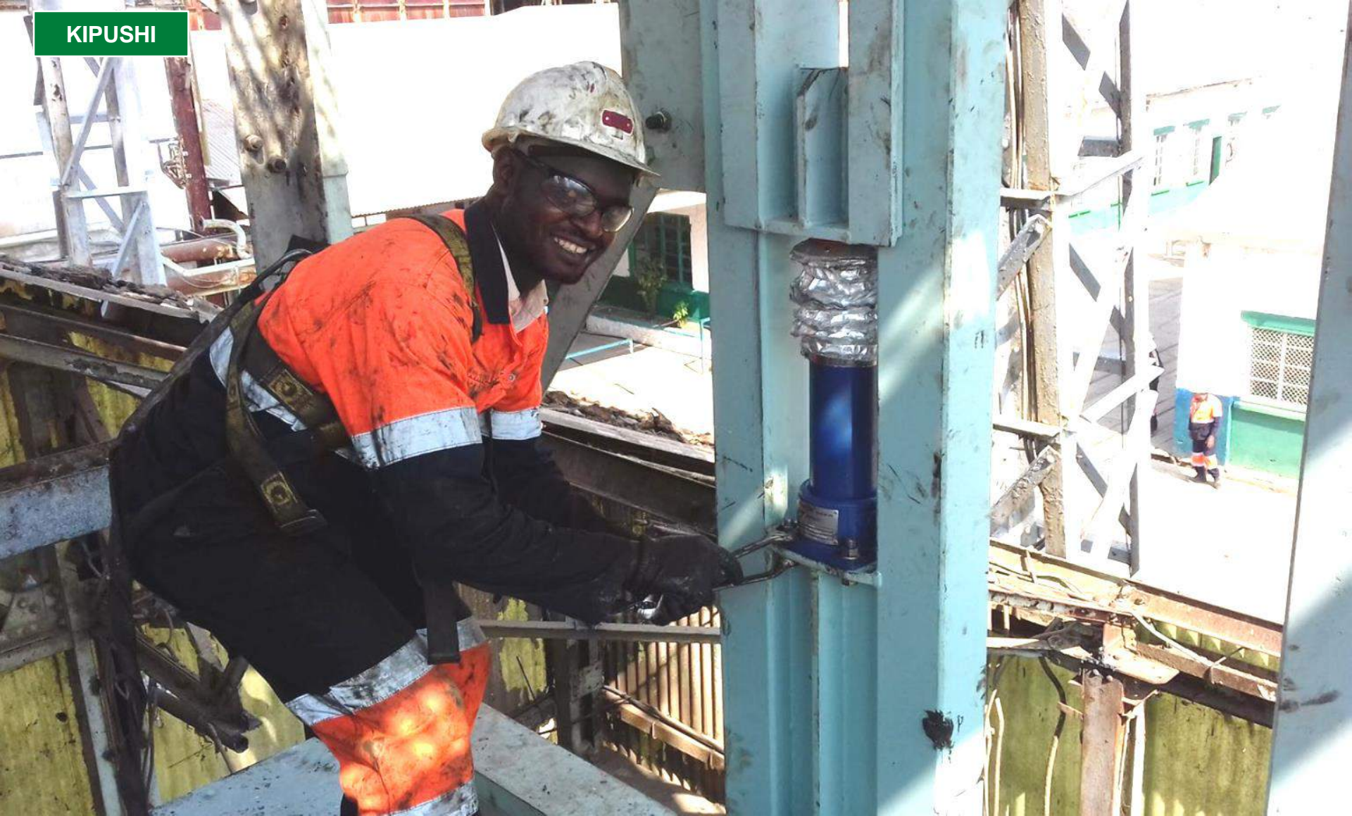
Ilunga Kabinga, a winder fitter, installing jack catches on Kipushi's Shaft 2 headgear.
