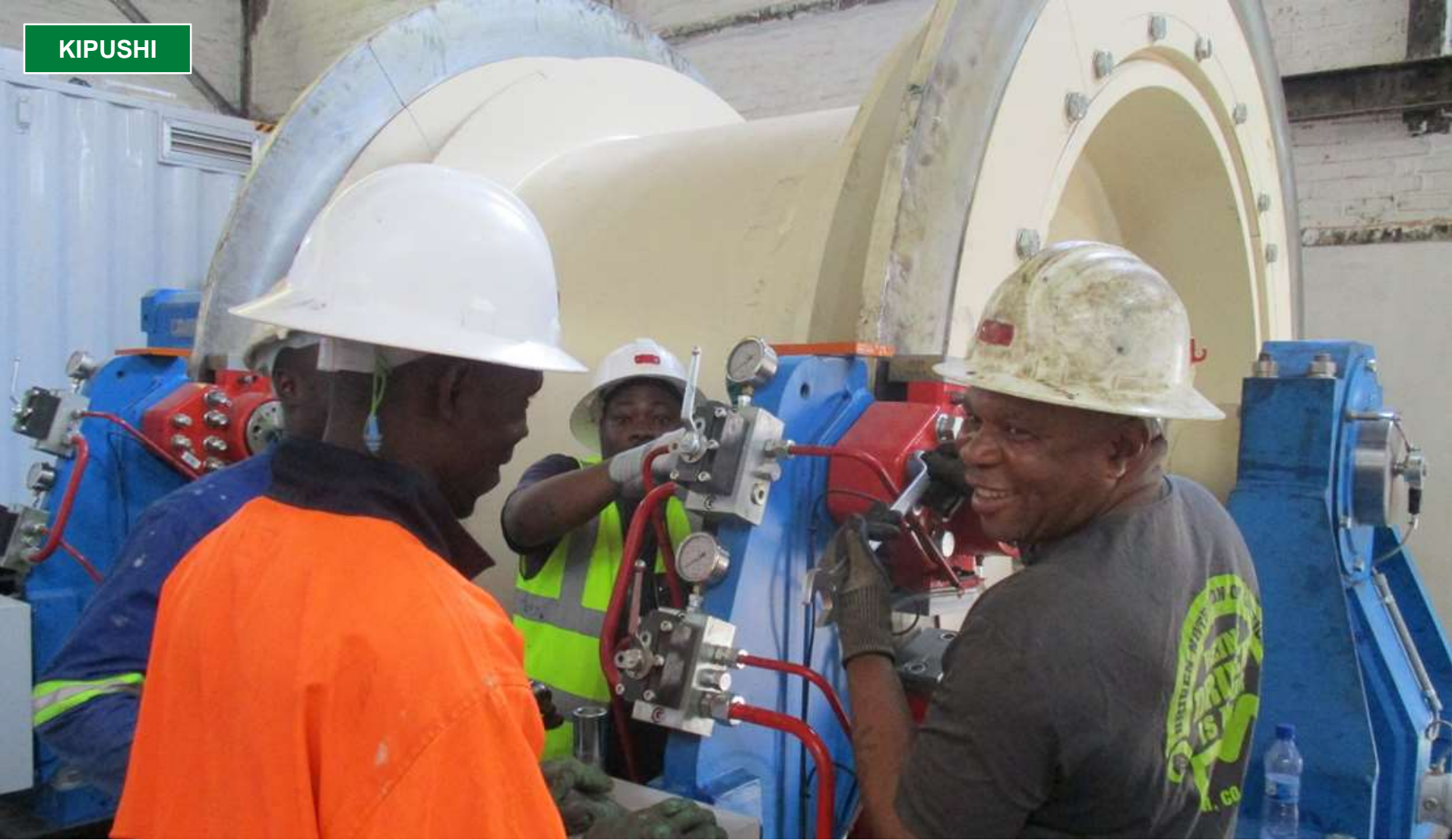
Mulambe Kafwimbi (right) and members of DRC contractor Tech-Edge installing brakes calipers on Kipushi's new Shaft 2 winder.
