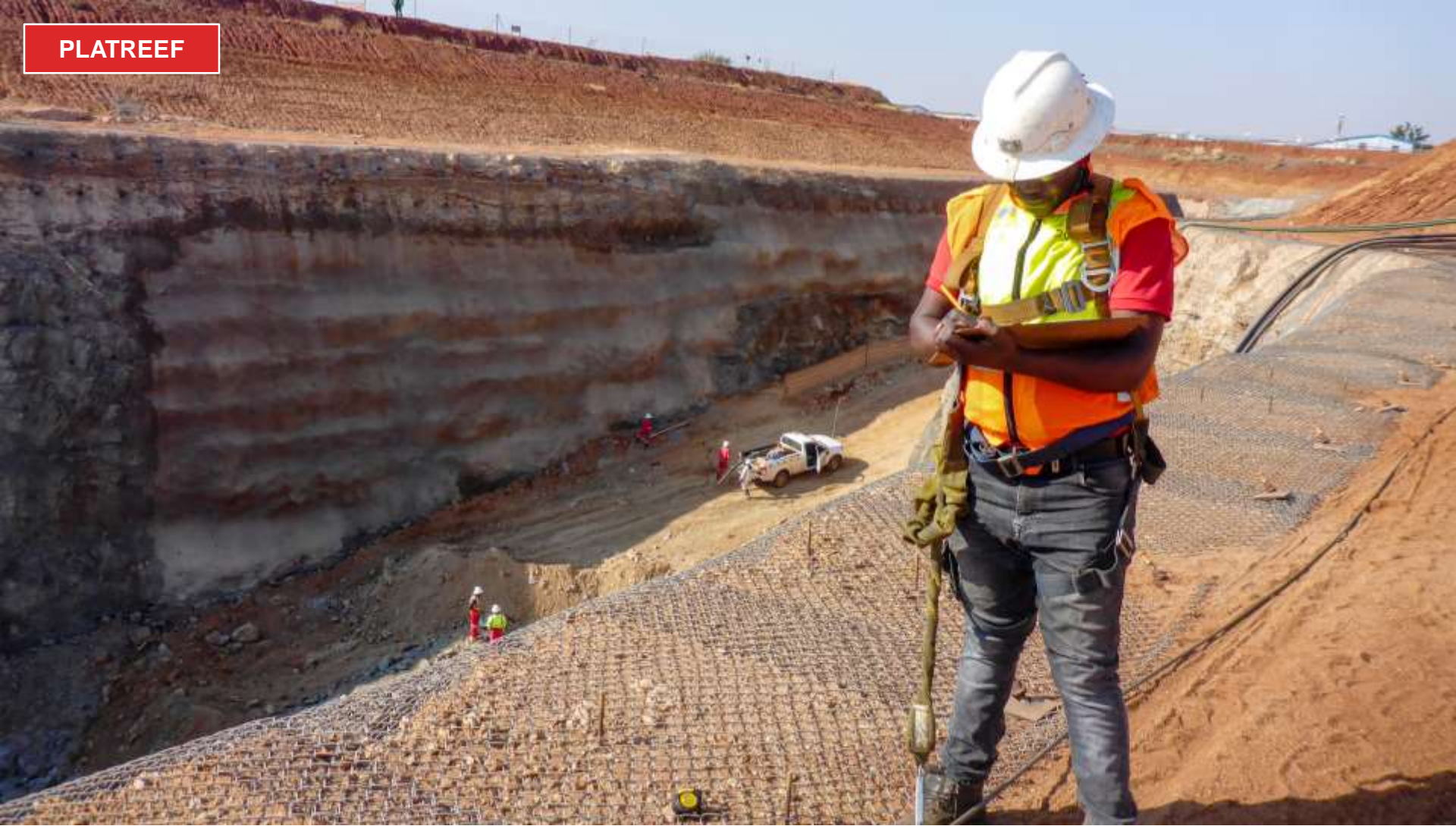
Geotechnical trainee Johannes Nkhoma conducting a weekly inspection on the five-metre bench of the Shaft 2 box cut.
