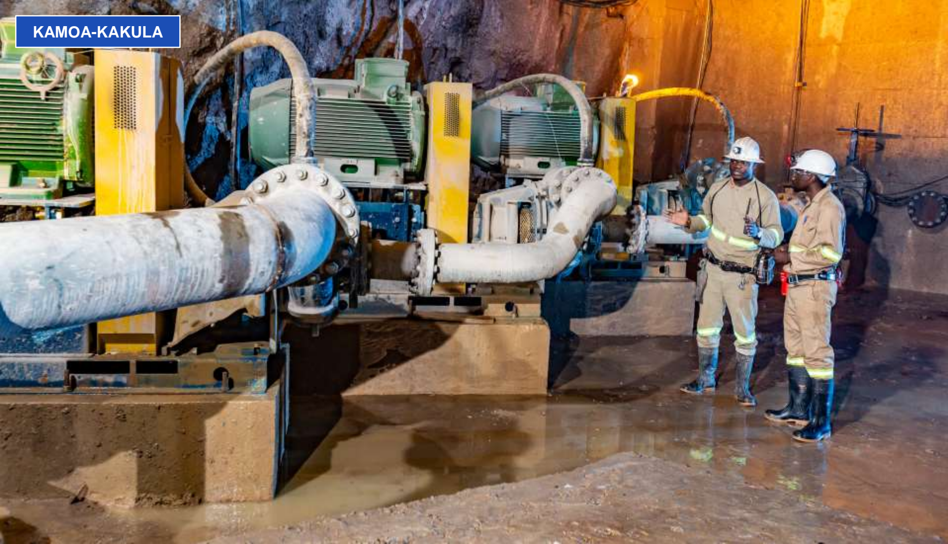
Members of the Kakula underground development team conducting tests at the new pumping station.
