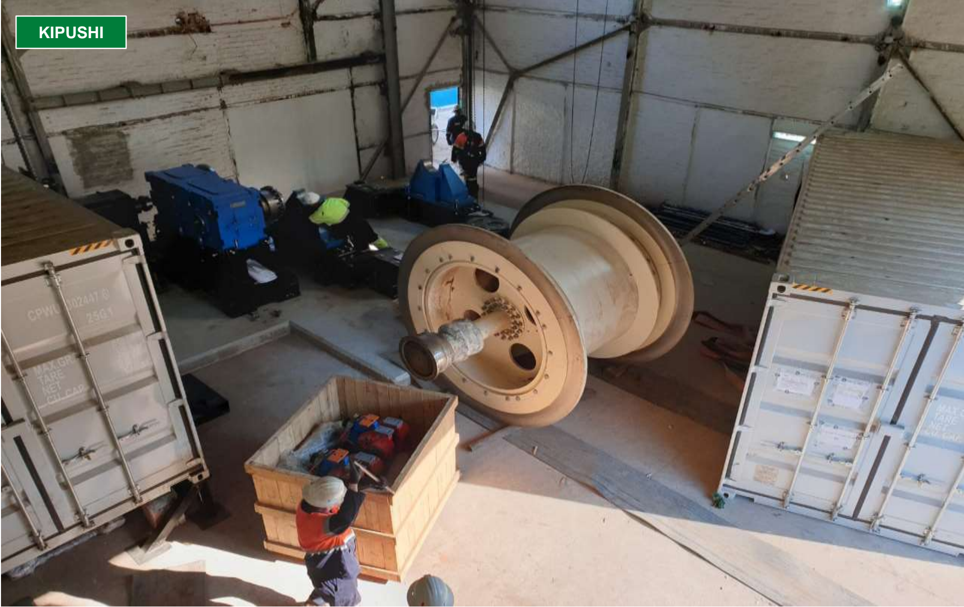
Installing Kipushi's new P2 winder.
