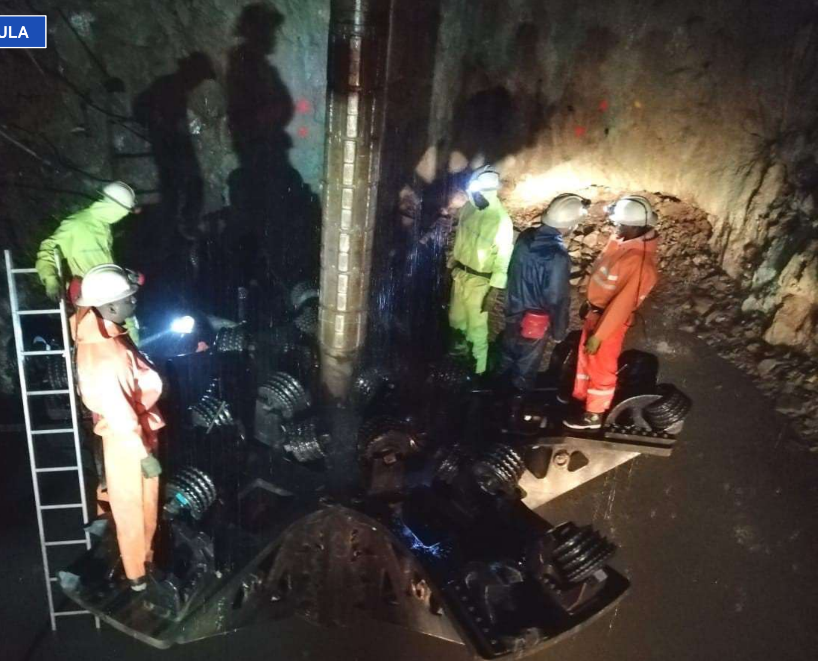
Hooking up the reamer unit to the drill rods at Kakula's ventilation shaft 1.
