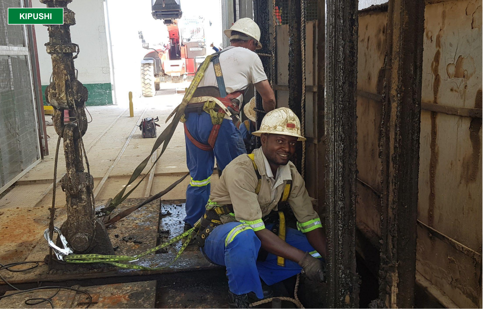
Ilunga Kabinga, Kipushi's engineering foreman (front), removing a component from the old P2 cage.
