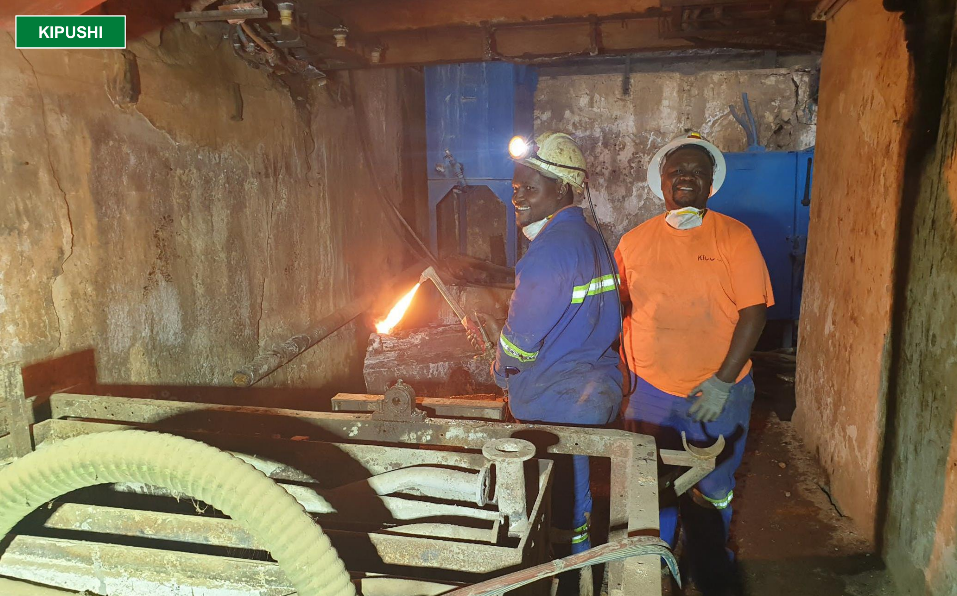
Cheridan Kasongo (left) and Alpheus Molepo cut out old components from the 1924 hoist as part of the P2 Shaft upgrading.
