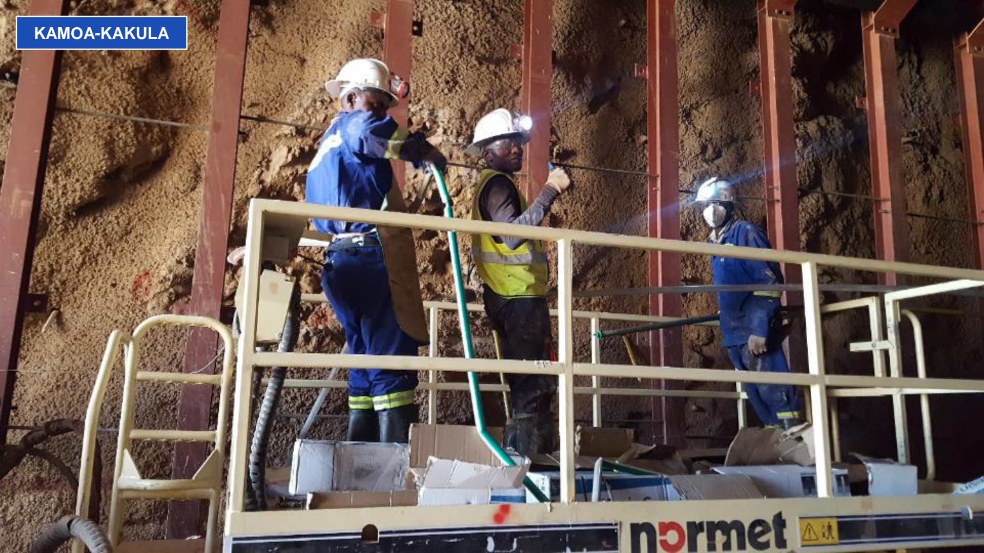
Installation of supporting steel sets in Kakula's southern decline.
