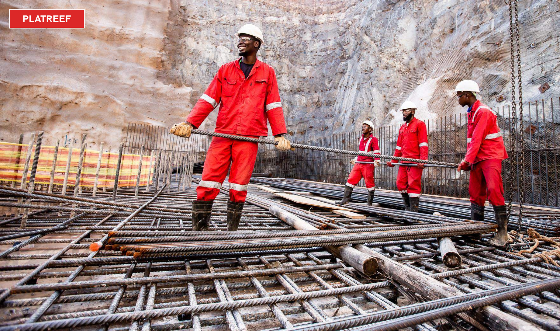
Anthony Baloyi, Mokopane Micraas, Abatian Manmela and Ruddy Malete (left to right), of South Africa-based Malecombo Steel Fixers, installing steel rebar for Shaft 2's concrete foundation, which is expected to be completed mid-2019.
