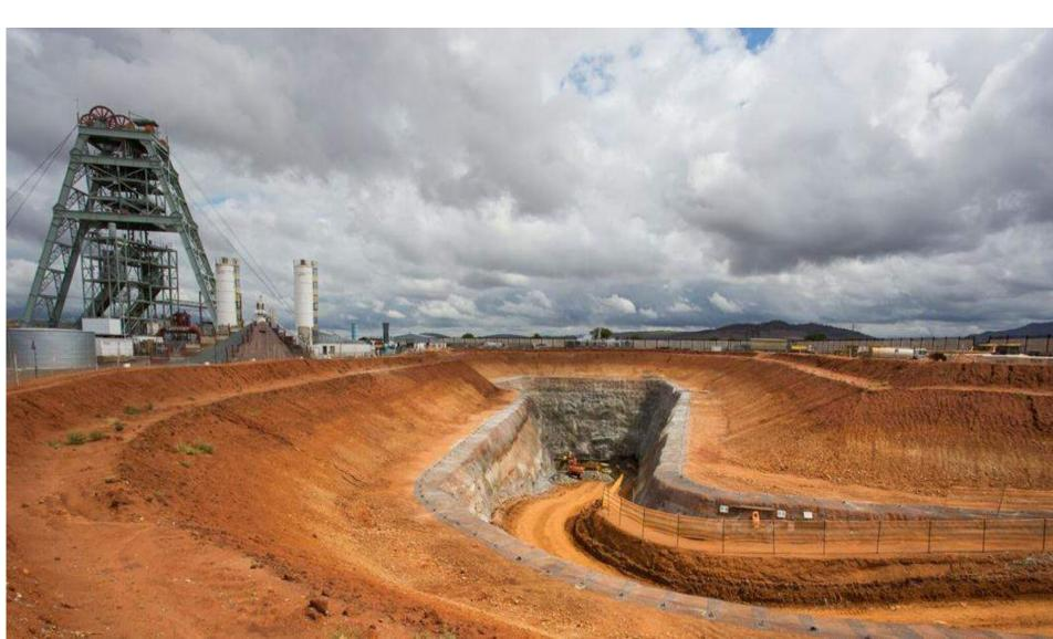
Platreef's Shaft 2 box cut, with the 11.5-metre shaft ring set-up for the 10-metre internal diameter shaft.
