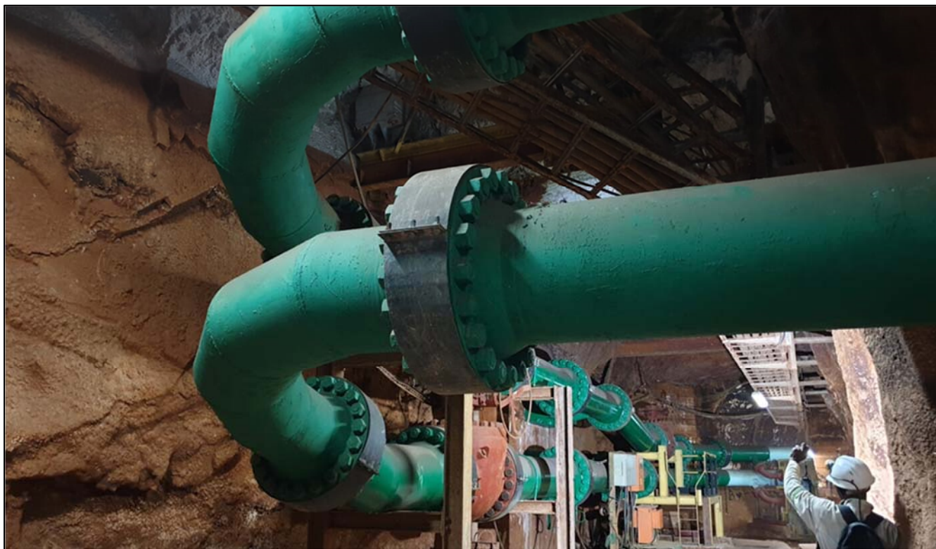
Photo: High-volume water pipes to keep Kipushi's underground workings dry.
