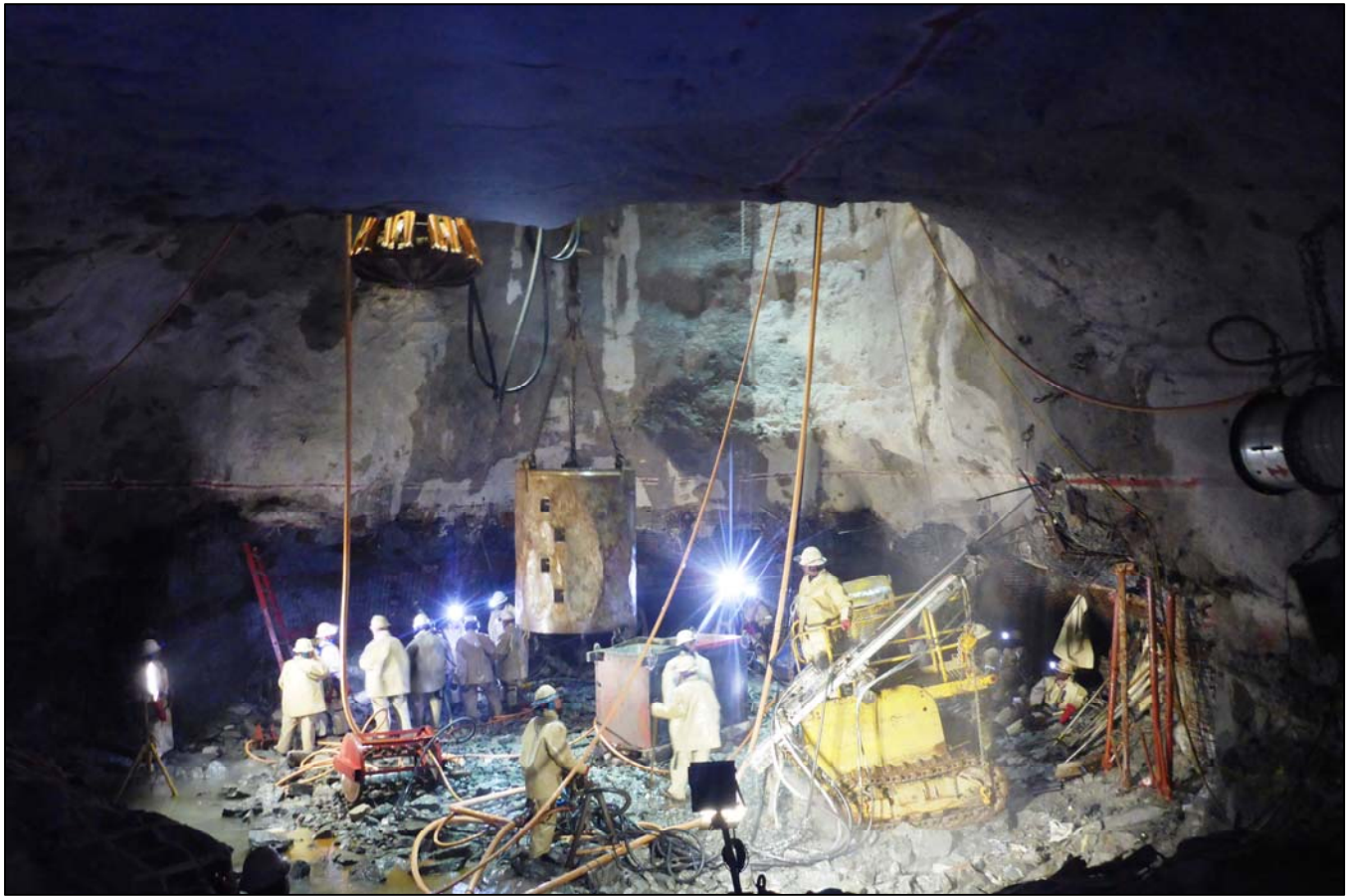
Photo: Spraying shotcrete over 6.5-metre anchor bolts and wire mesh to reinforce the brow at Shaft 1's 850-metre-level mine access station.
