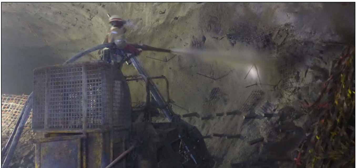
Photo: Spraying shotcrete over 6.5-metre anchor bolts and wire mesh to reinforce the brow at Shaft 1's 850-metre-level mine access station.
