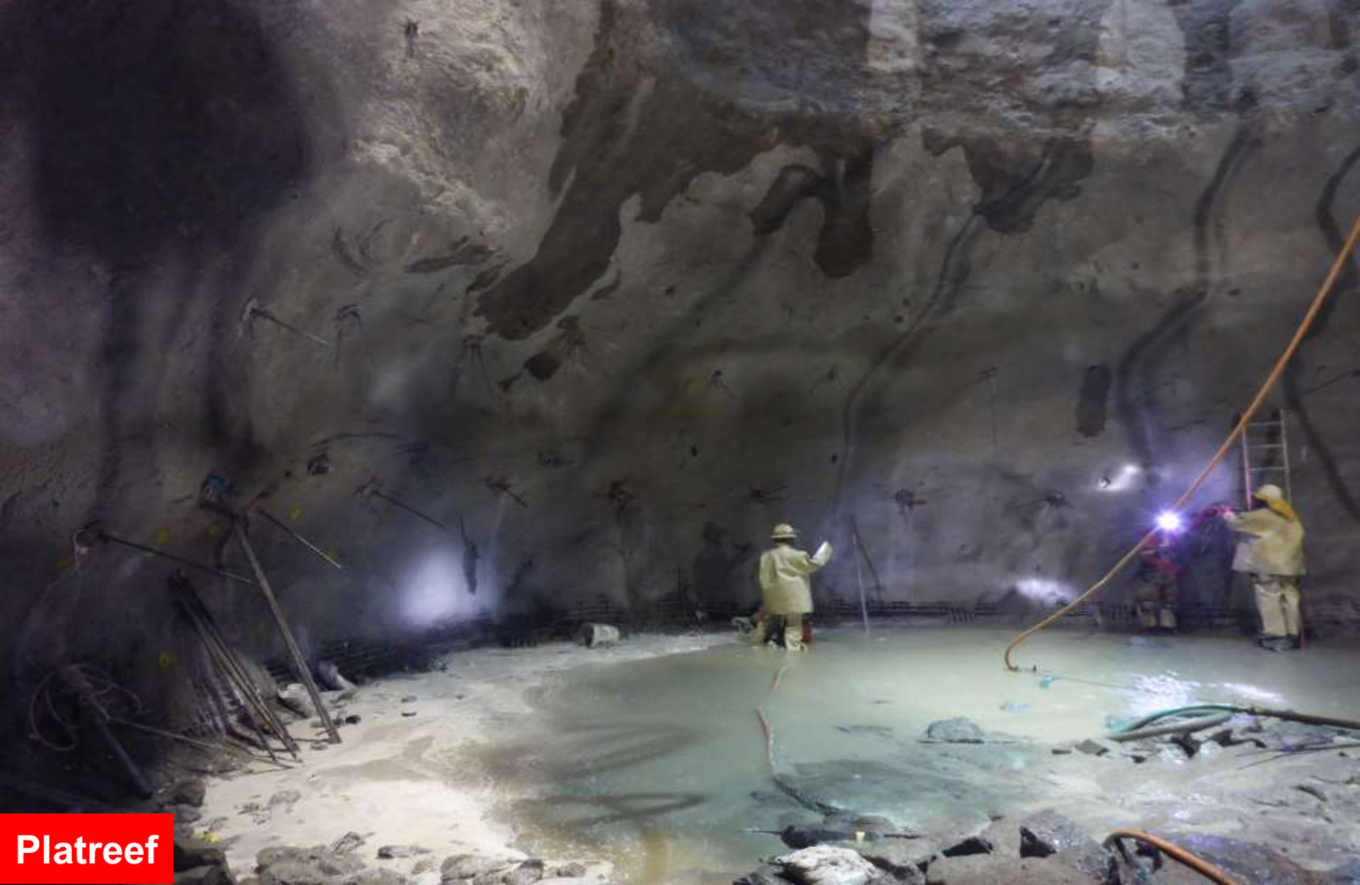
Final tensioning and grouting of 6.5-metre anchor bolts in the brow of the 850-metre-level station on Shaft 1.
