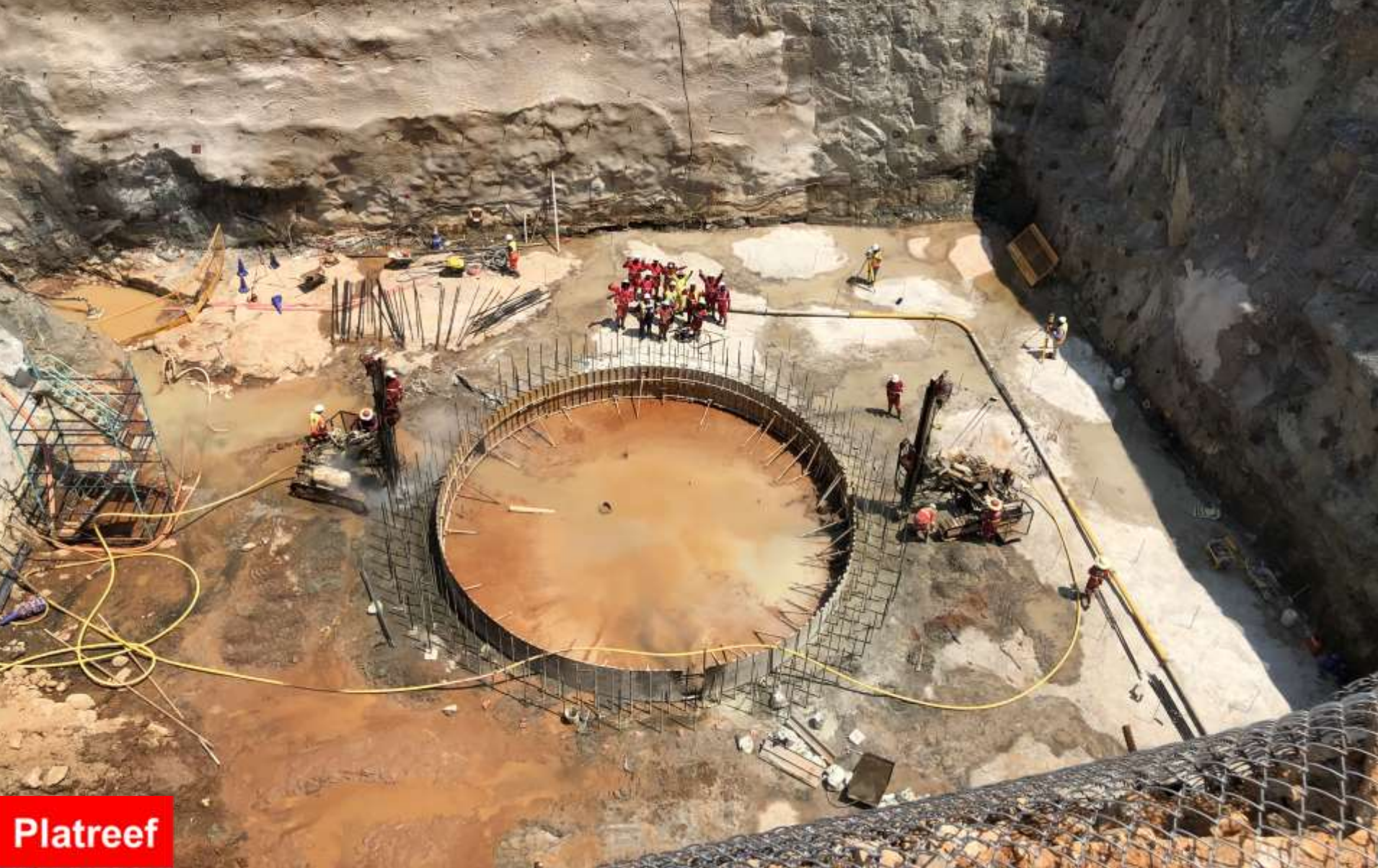
Contract employees from Gauteng, South Africa-based Terra Strata celebrating the completion of drilling for the steel pins (spiles) at the bottom of the concrete foundation that will support Shaft 2's headframe.
