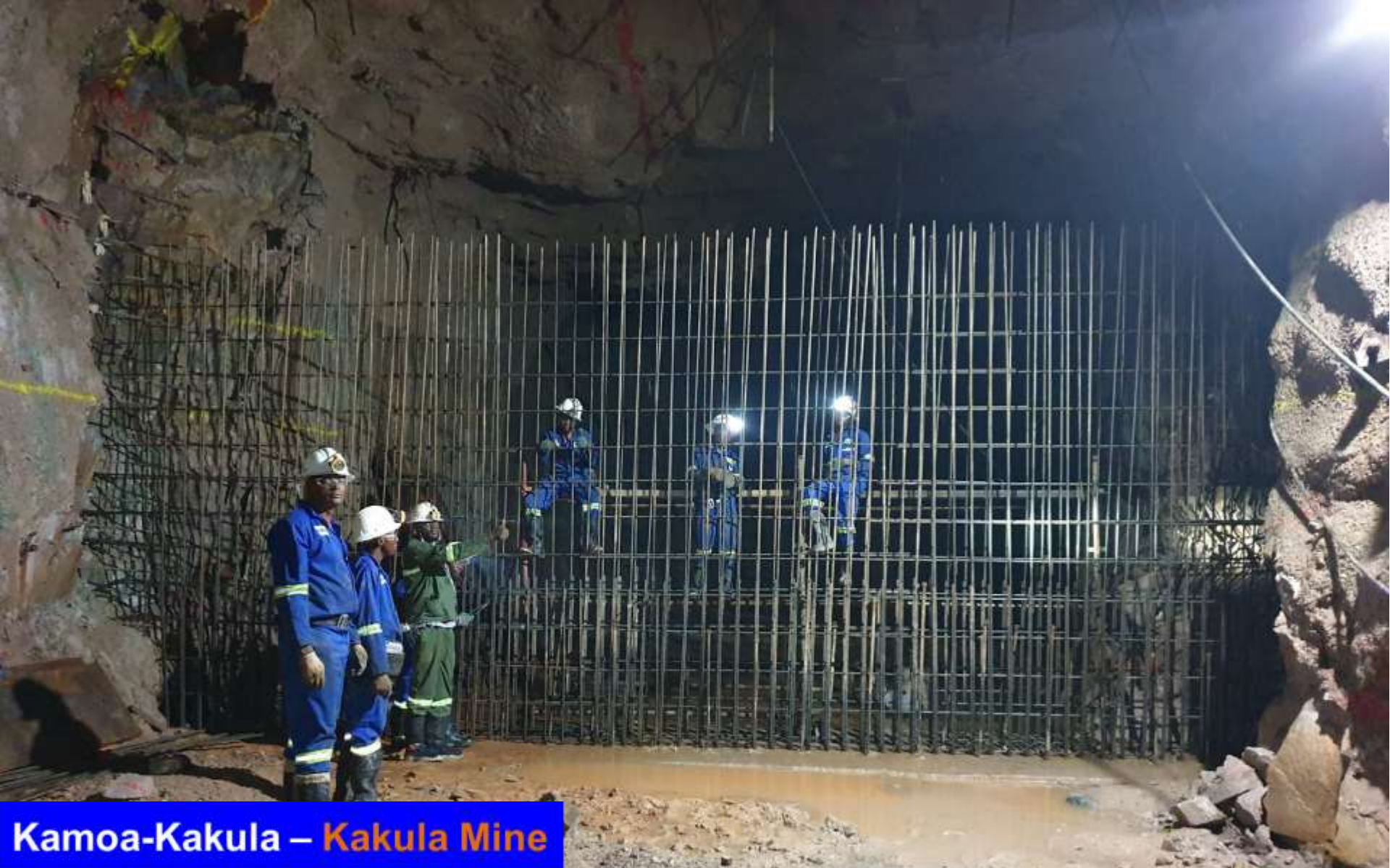
Construction of an underground dam at the Kakula Mine. The stored water will be used for mining operations, with the excess pumped to surface settling ponds.
