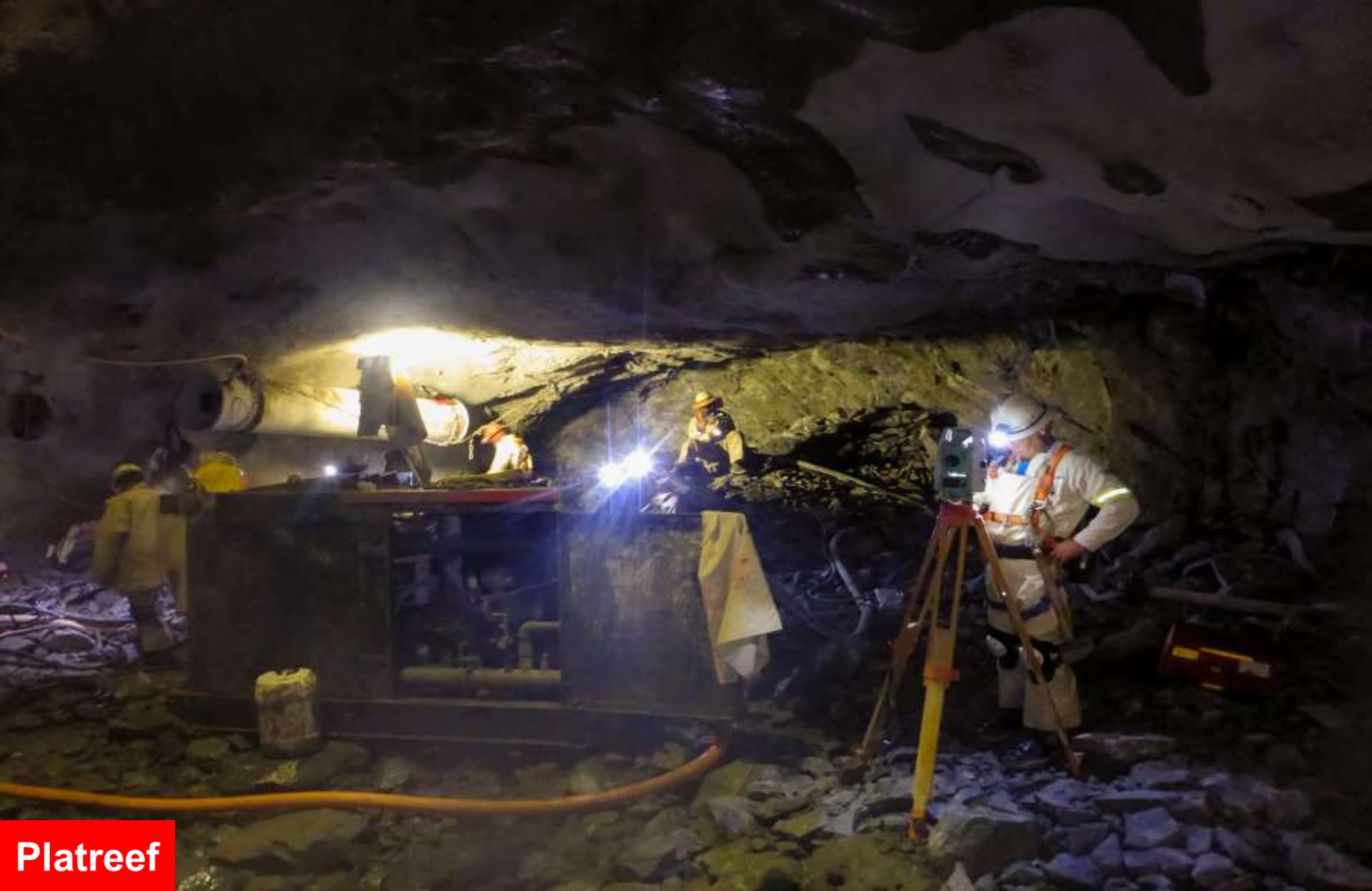
Shaft 1's 850-metre-level station development. The bottom of the shaft now is at a depth of 855 metres below surface.
