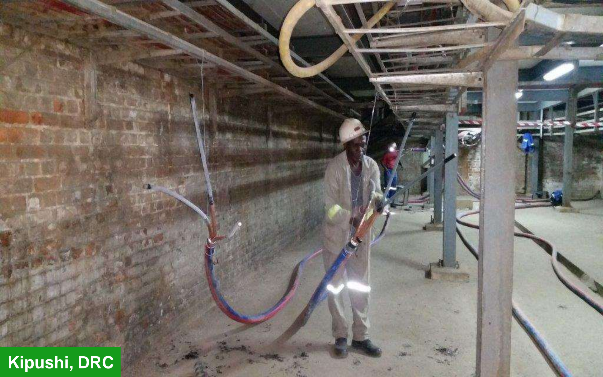
KICO electricians installing high-voltage electrical cables on Kipushi's 850-metre level.
