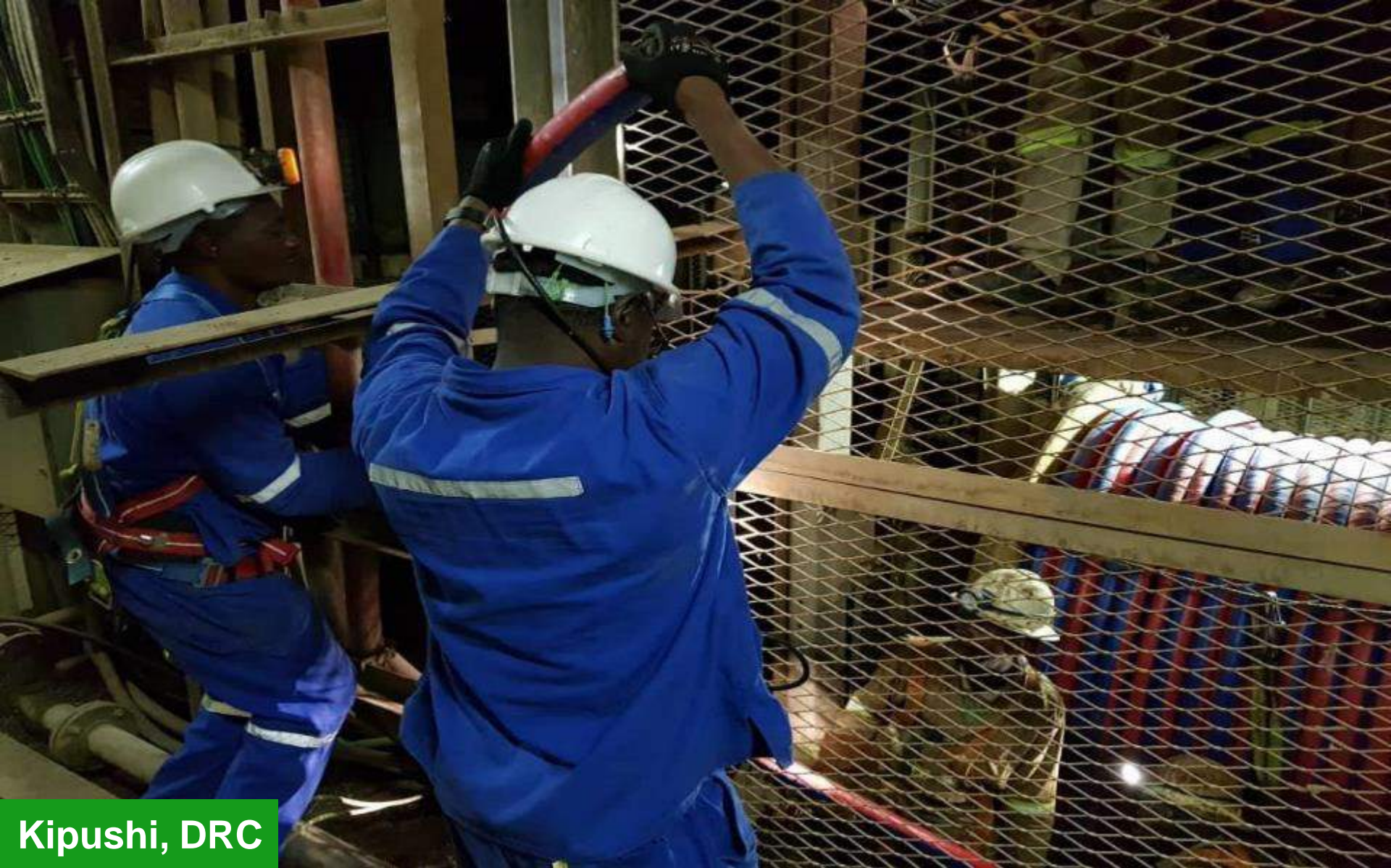
Workers installing a high-voltage electrical cable underground at the Kipushi Mine.
