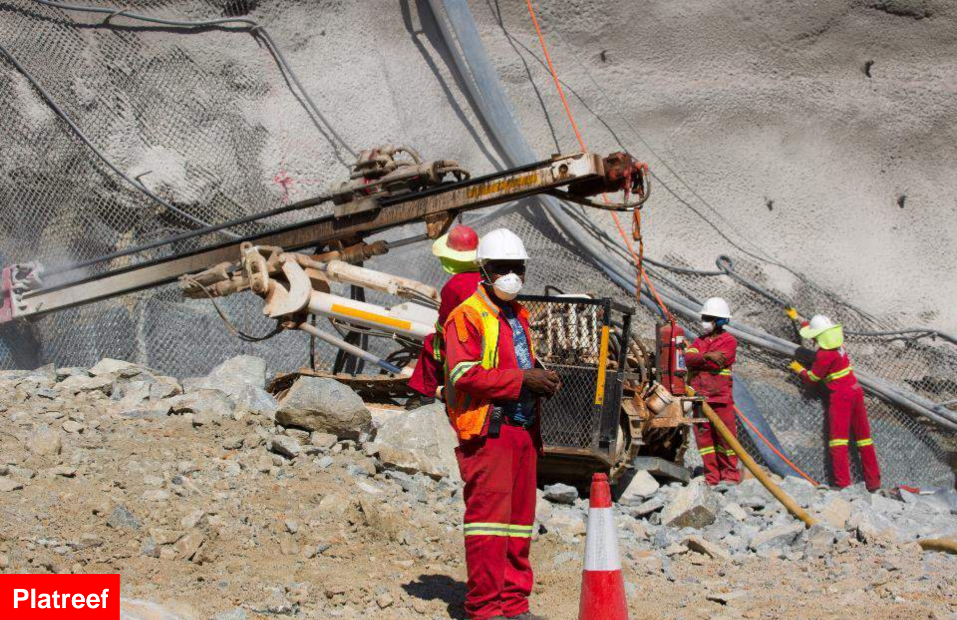
Installing slope-stability anchors in the box cut for Shaft 2.
