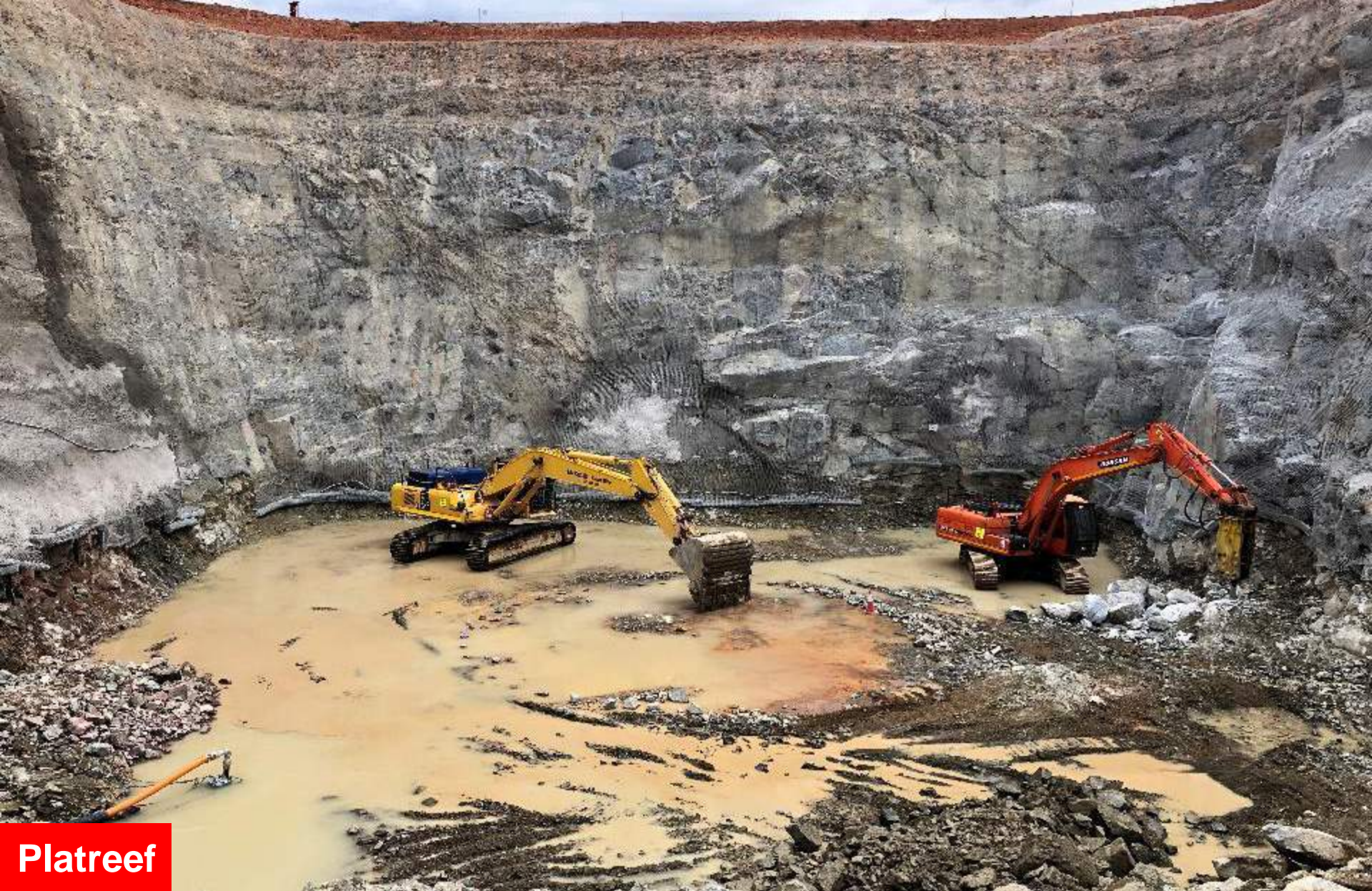
Bottom of the box cut for Shaft 2, showing the 10-metre-diameter outline for the planned shaft.
