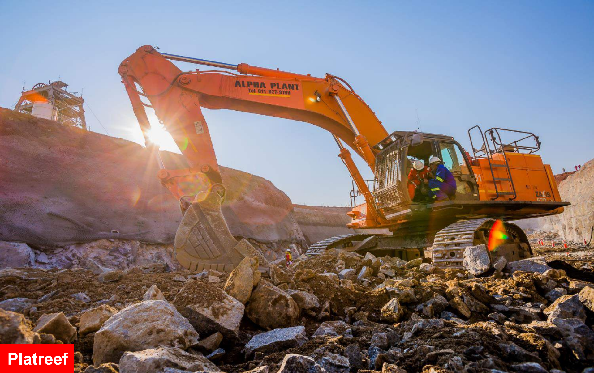
Removing blasted rock from the box cut for Shaft 2 at the Platreef Mine. Work on the box cut is expected to be completed early in 2019.
