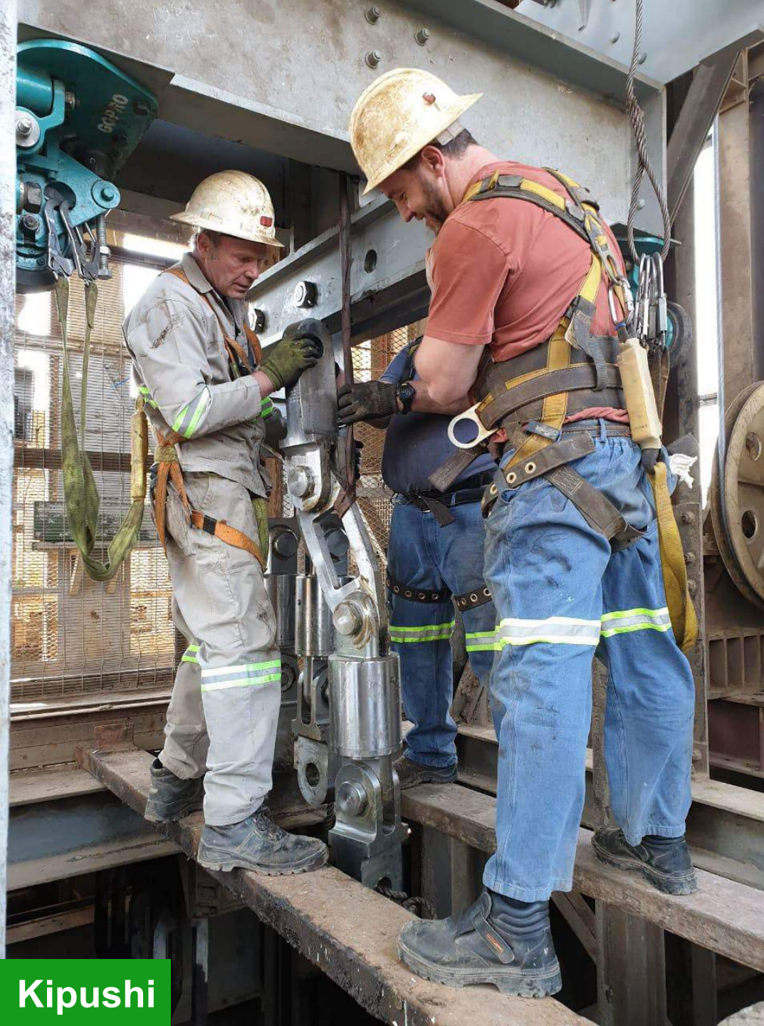
Rigger Eugene Botha (left) and fitter Graham Muldoon installing tail-rope attachments on the new Shaft 5 rock winder.
