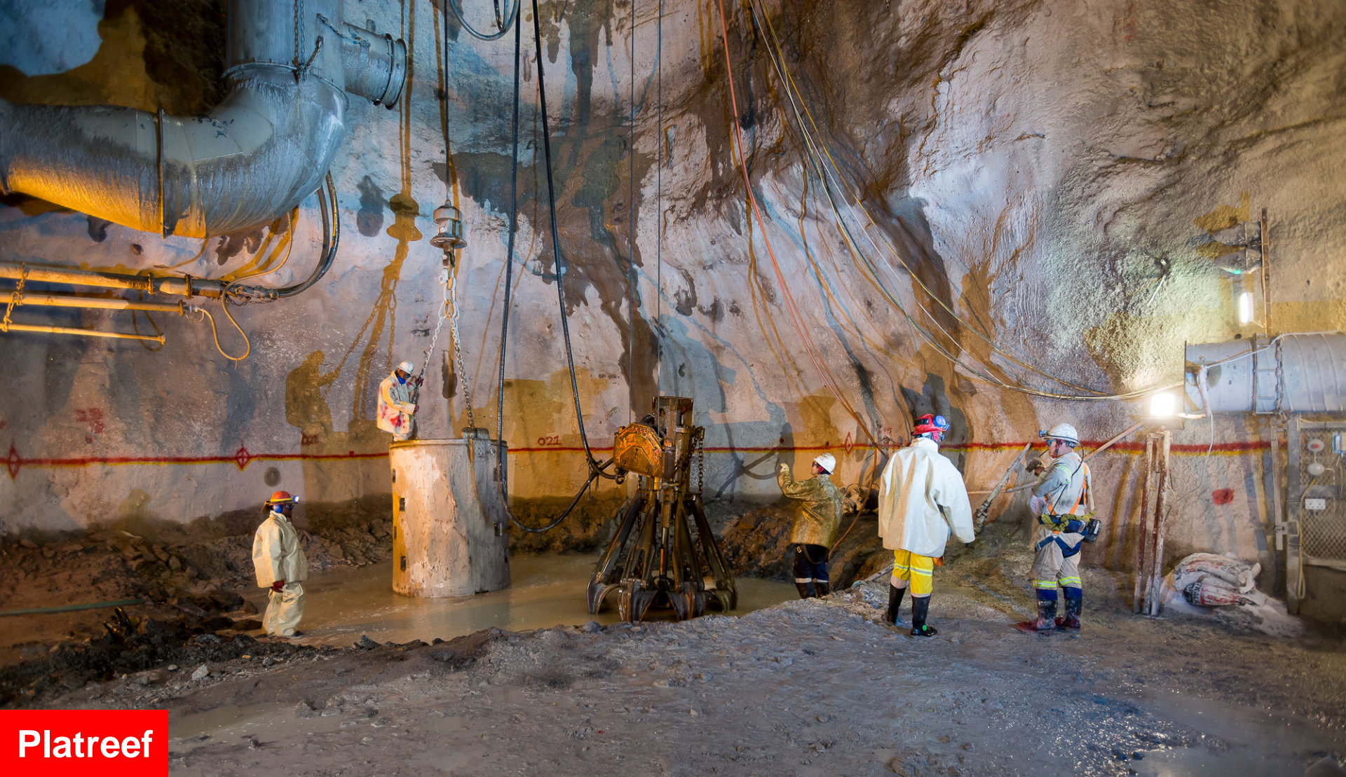
A kibble bucket (mid-left) and 'cactus grab' (mid-right) being used to collect and remove excavated rock at Shaft 1's 750-metre level after the resumption of shaft-sinking work earlier this month.
