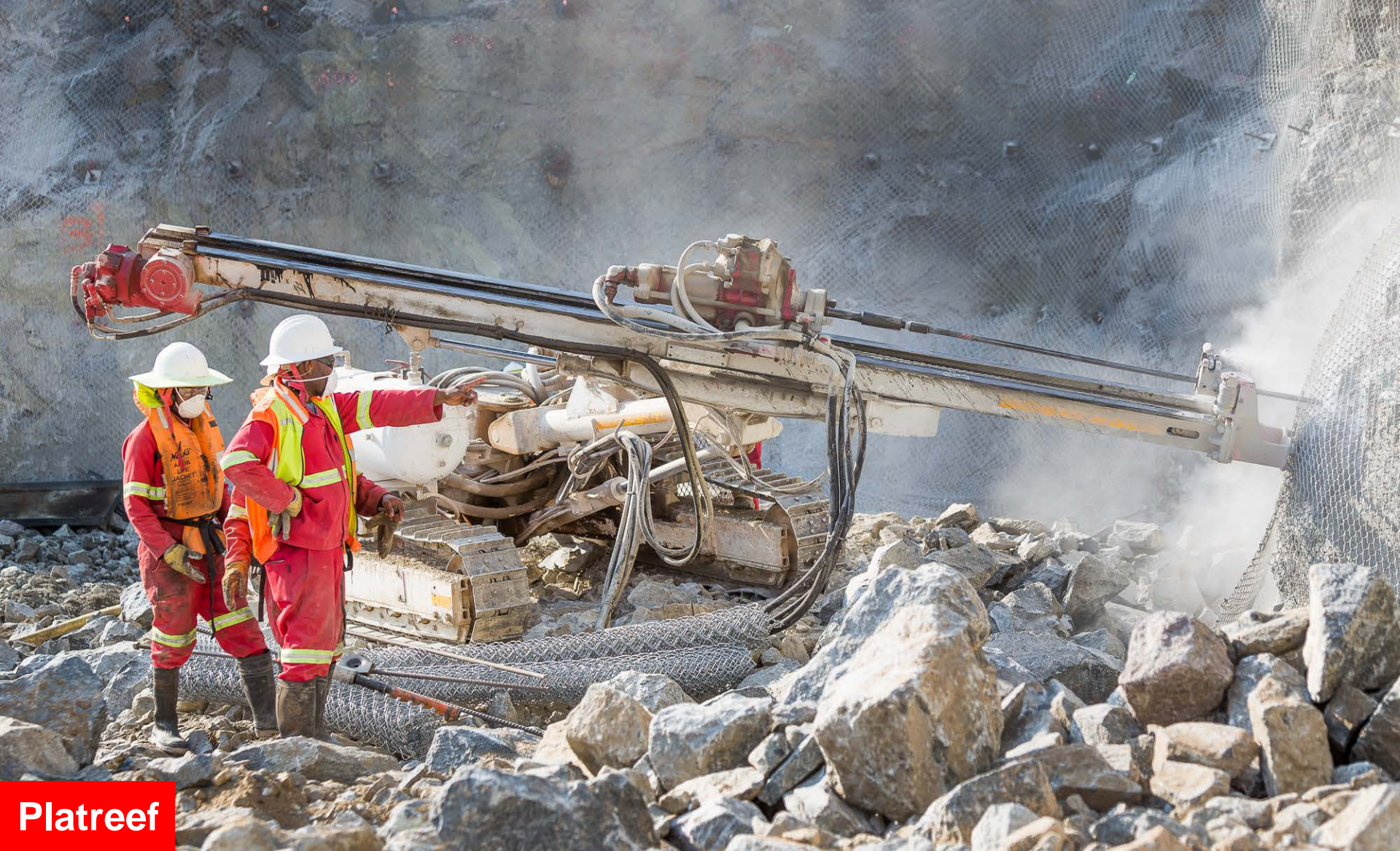
Horizontal drilling to insert rock bolts used to reinforce and support the walls of the Shaft 2 box cut.
