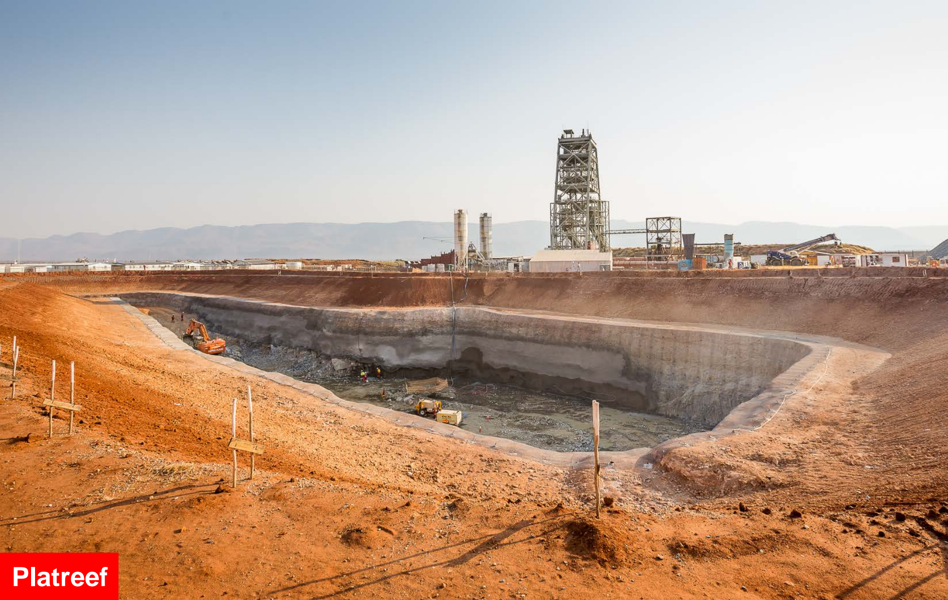
Platreef's Shaft 2 box cut, with Shaft 1 headframe in the background.
