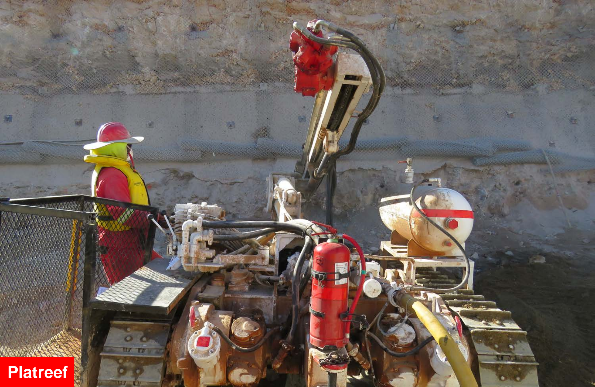
Horizontal drilling to insert rock bolts used to reinforce and support the side walls at the box cut for Shaft 2.
