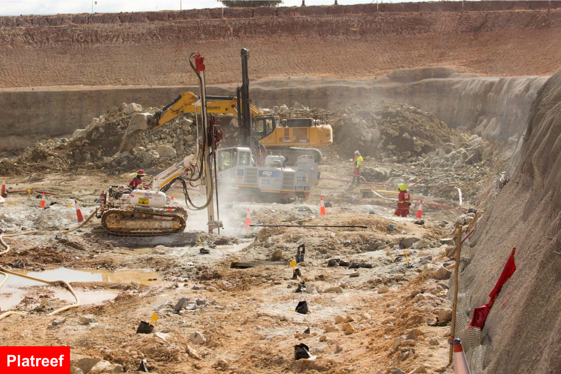
Vertical holes being drilled for explosives in preparation for another blast to deepen the box cut for Shaft 2.
