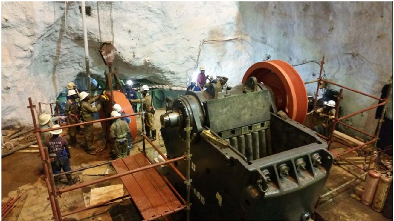
Figure 8: Installation of the two fly wheels (orange) onto the main frame of the new, primary rock crusher at Kipushi's 1,150-metre-level crusher station.
